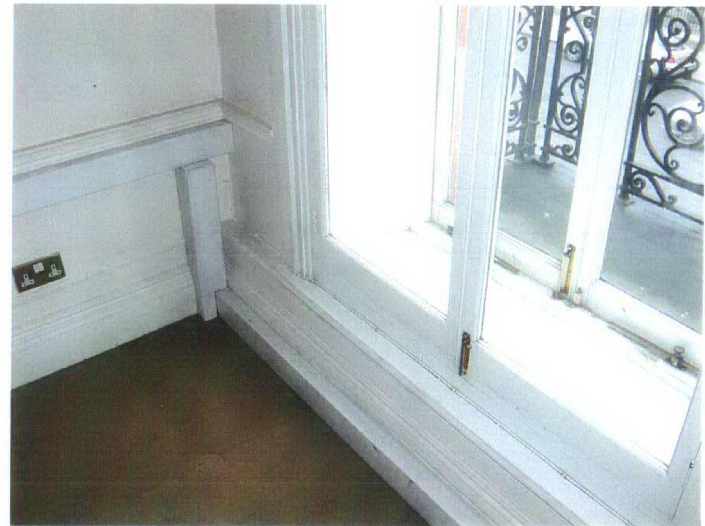
20 Existing secondary glazing first floor front room No.52
