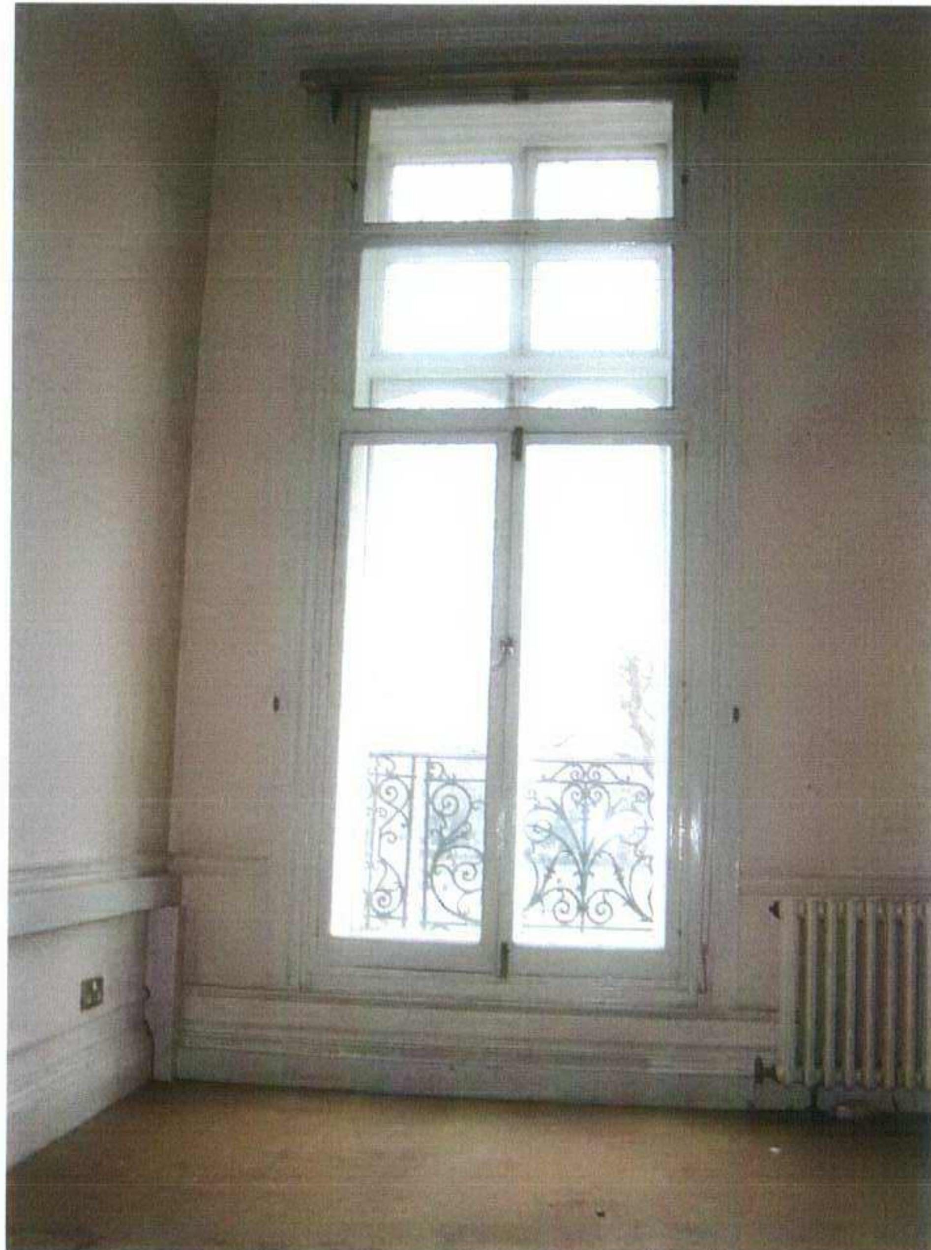
19 Existing mis-aligned secondary glazing first floor front room No.52
