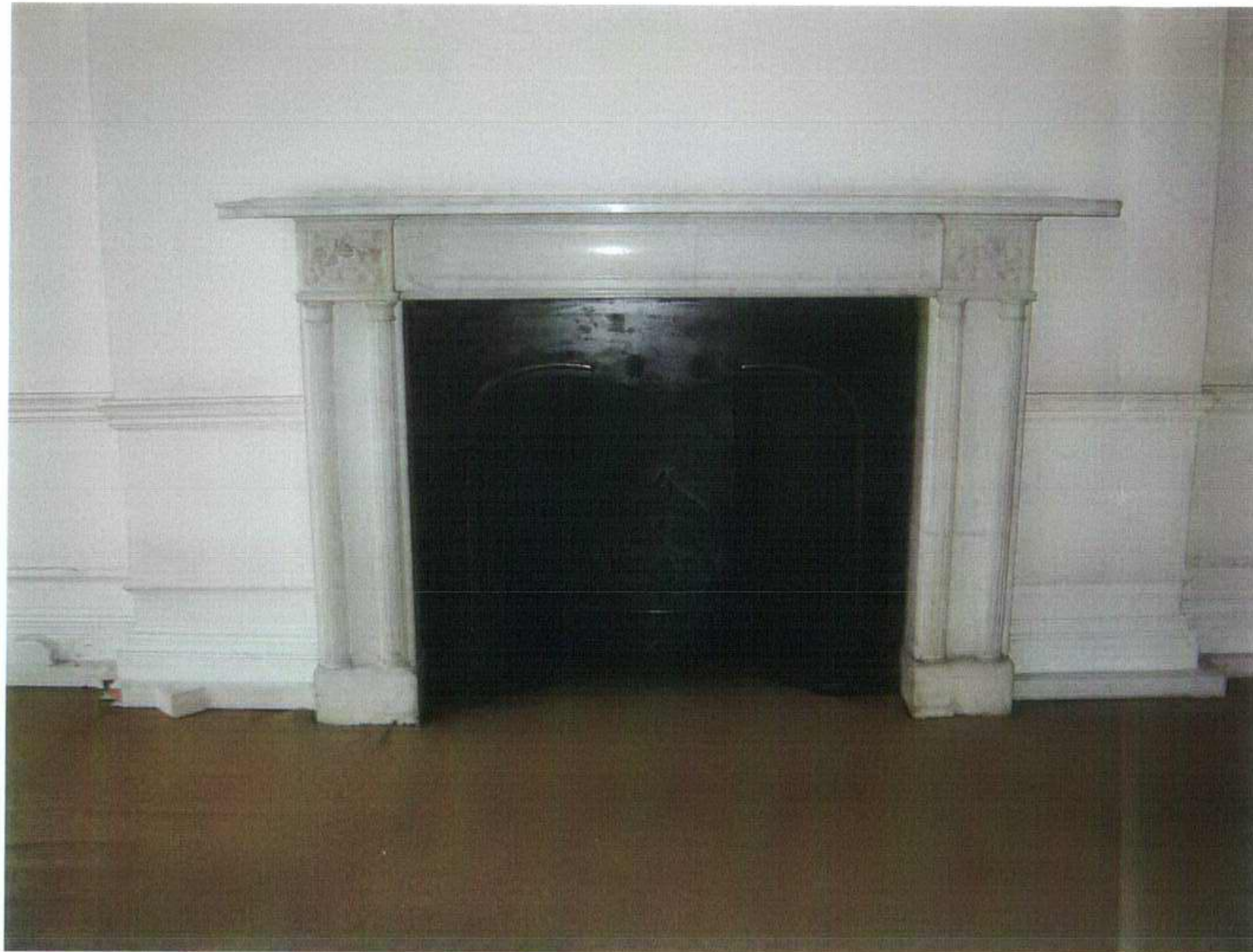
17 Existing fireplace first floor front room No.53
