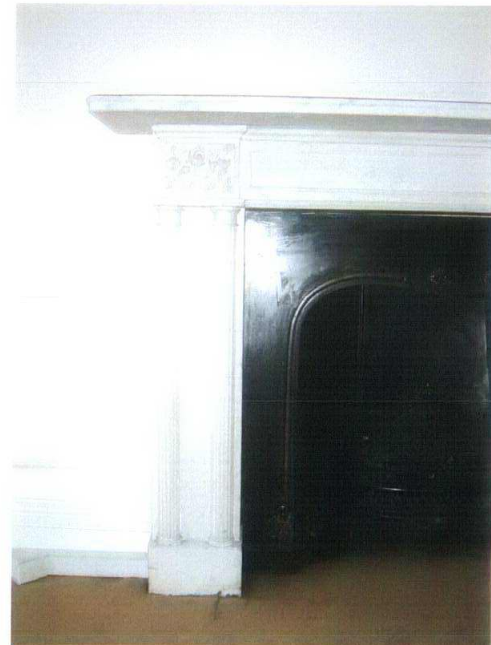
18 Existing fireplace first floor front room No.53
