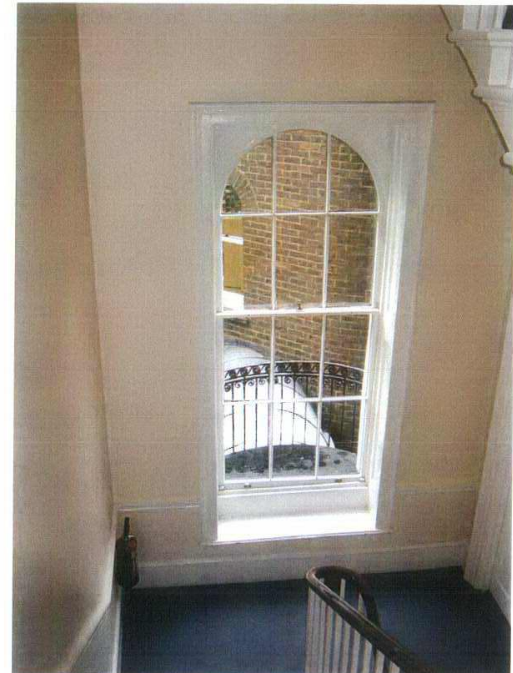
16 Stair landing window No.53
