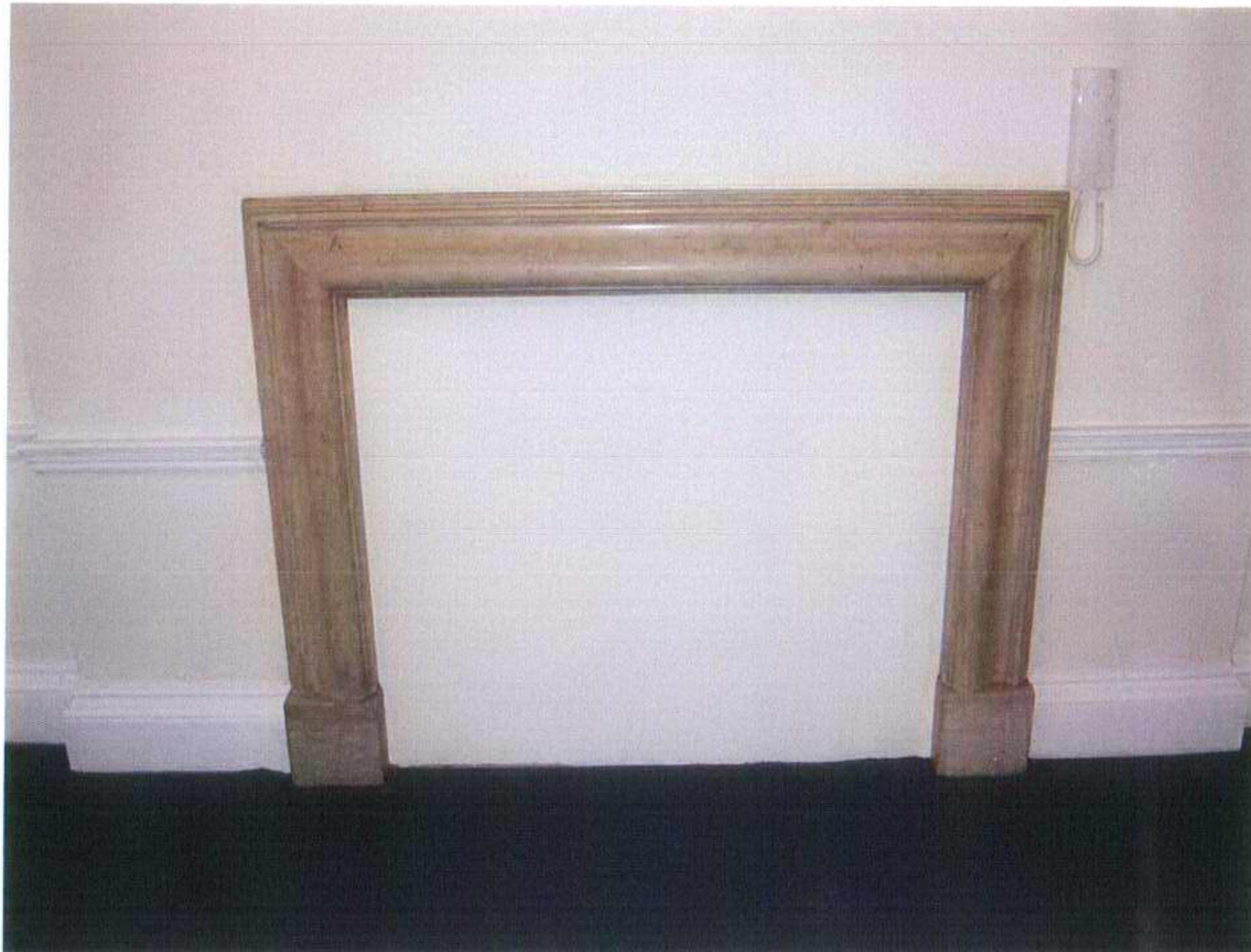
09 Existing fireplace ground floor front room No.52
