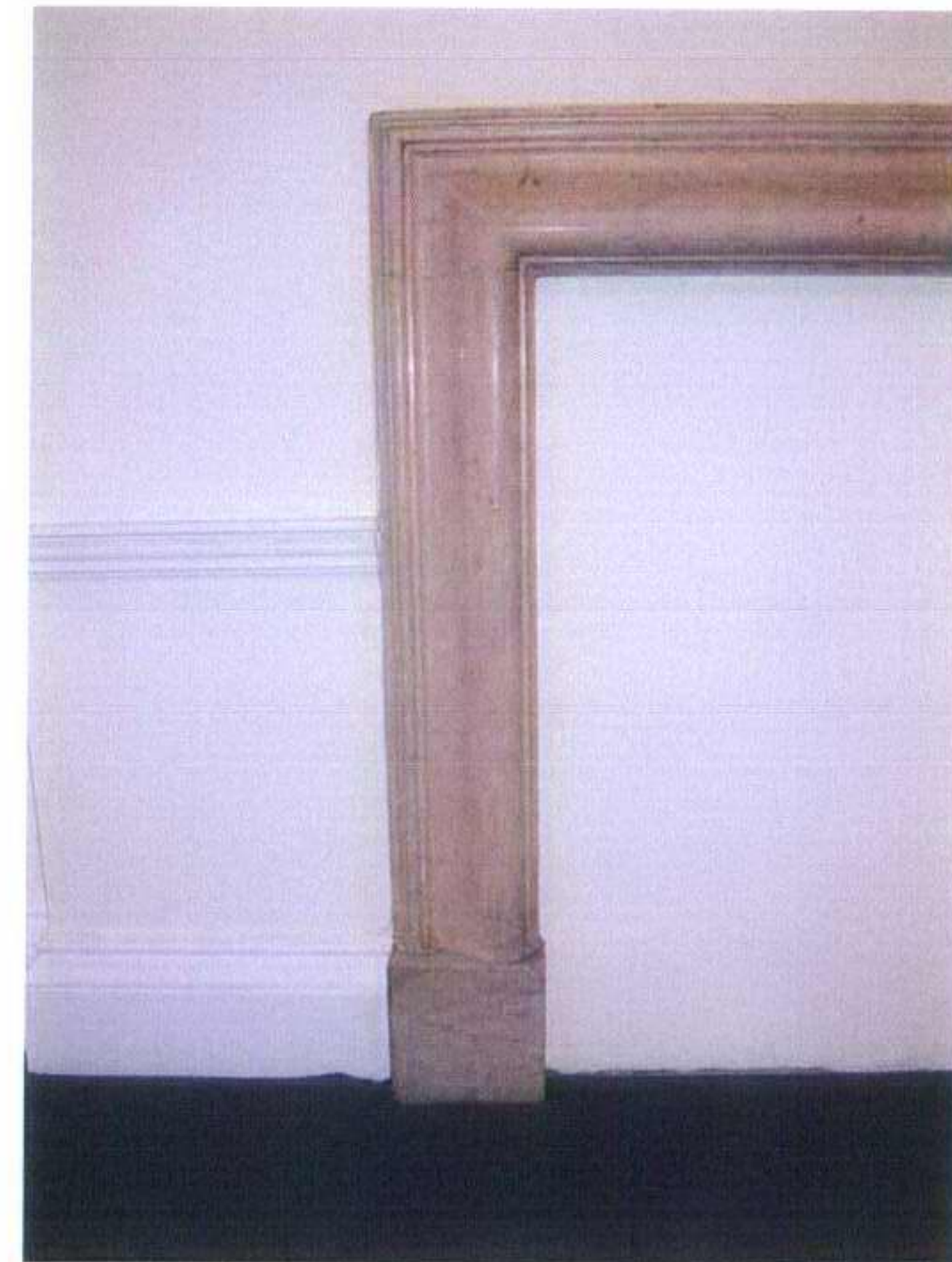
10 Existing fireplace ground floor front room No.52
