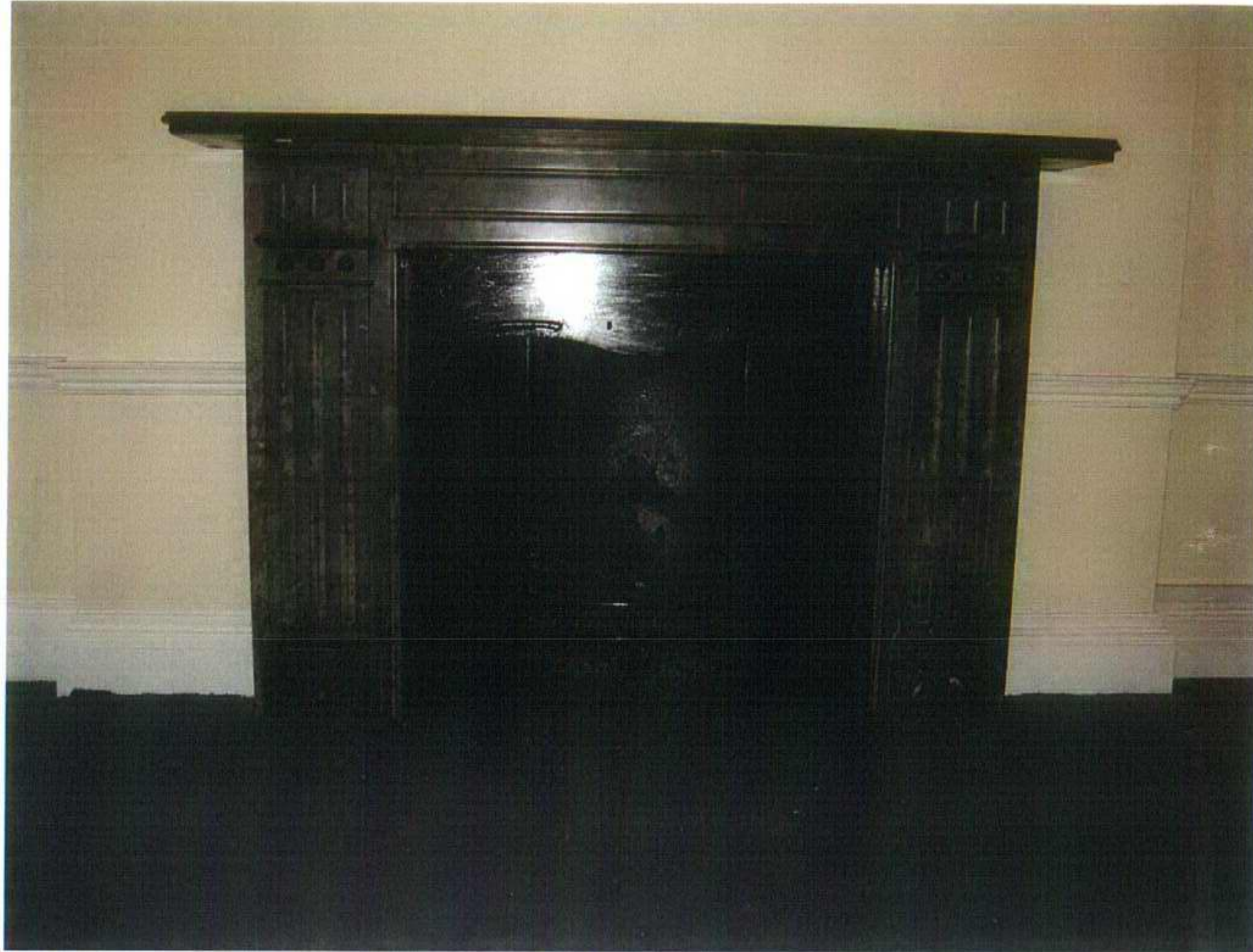
05 - Existing fireplace ground floor front room No.53
