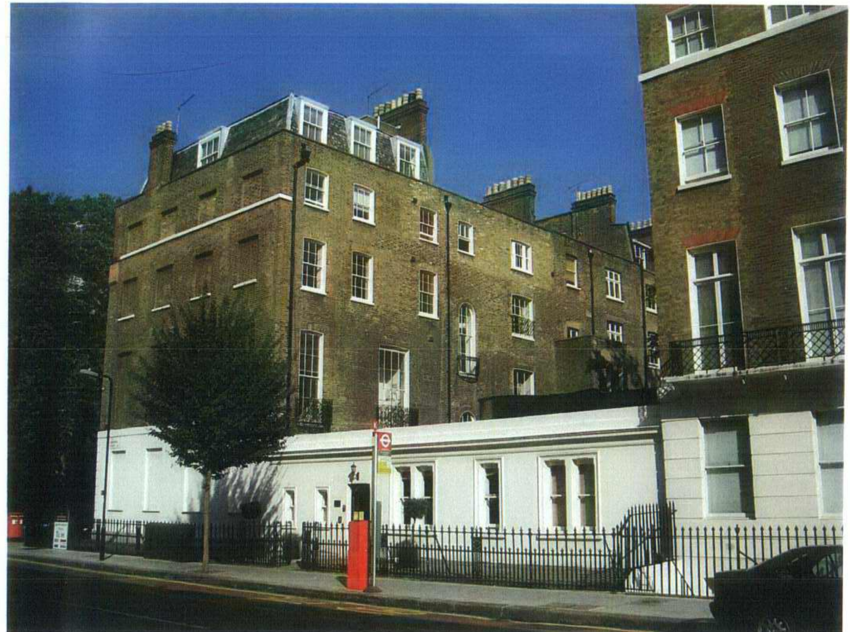
02 - Side elevation view from Bedford Place
