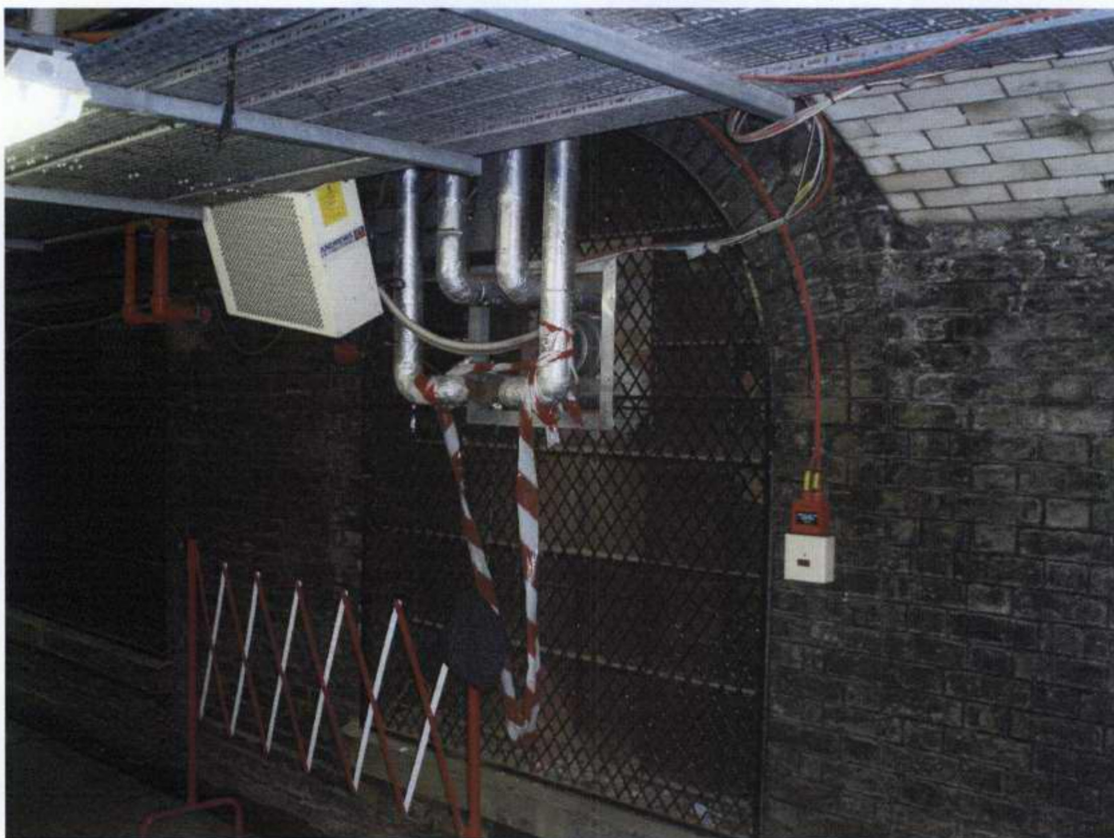
Existing Chilled Water Pipe Work
