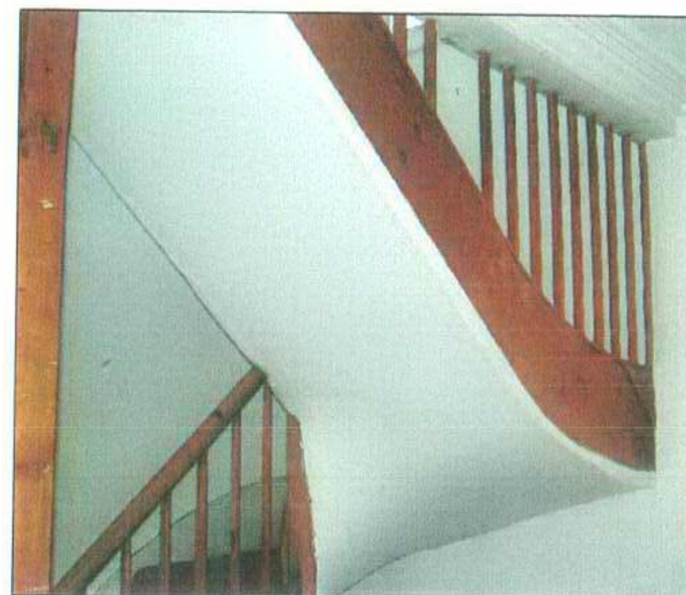
Ground floor stair to be rebuilt with flat half landing to allow access onto proposed roof terrace. Stair will be enclosed to comply with Building Regulations Part B.
