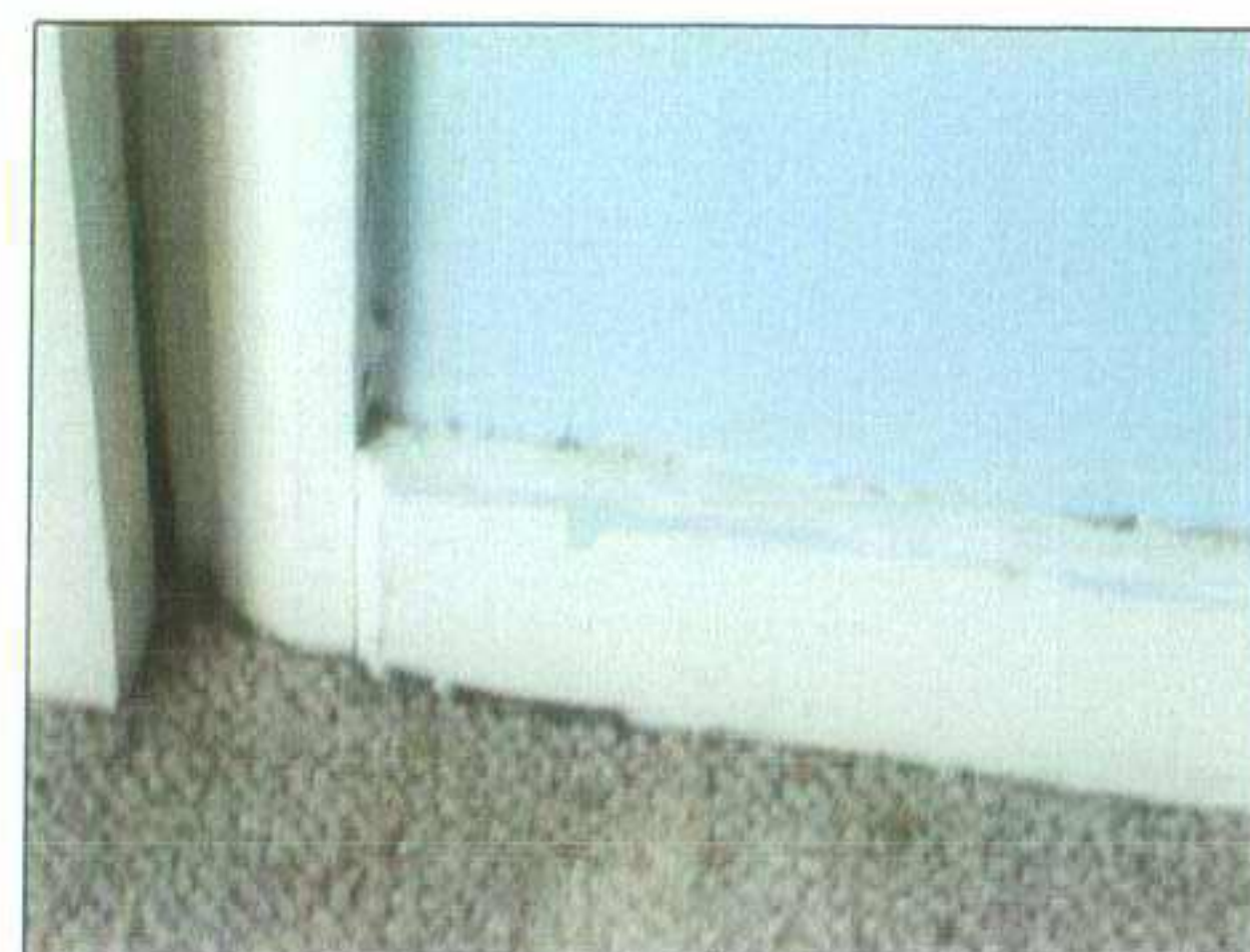
Existing skirting in basement to be replaced with square edge softwood skirting with 5mm chamfer
