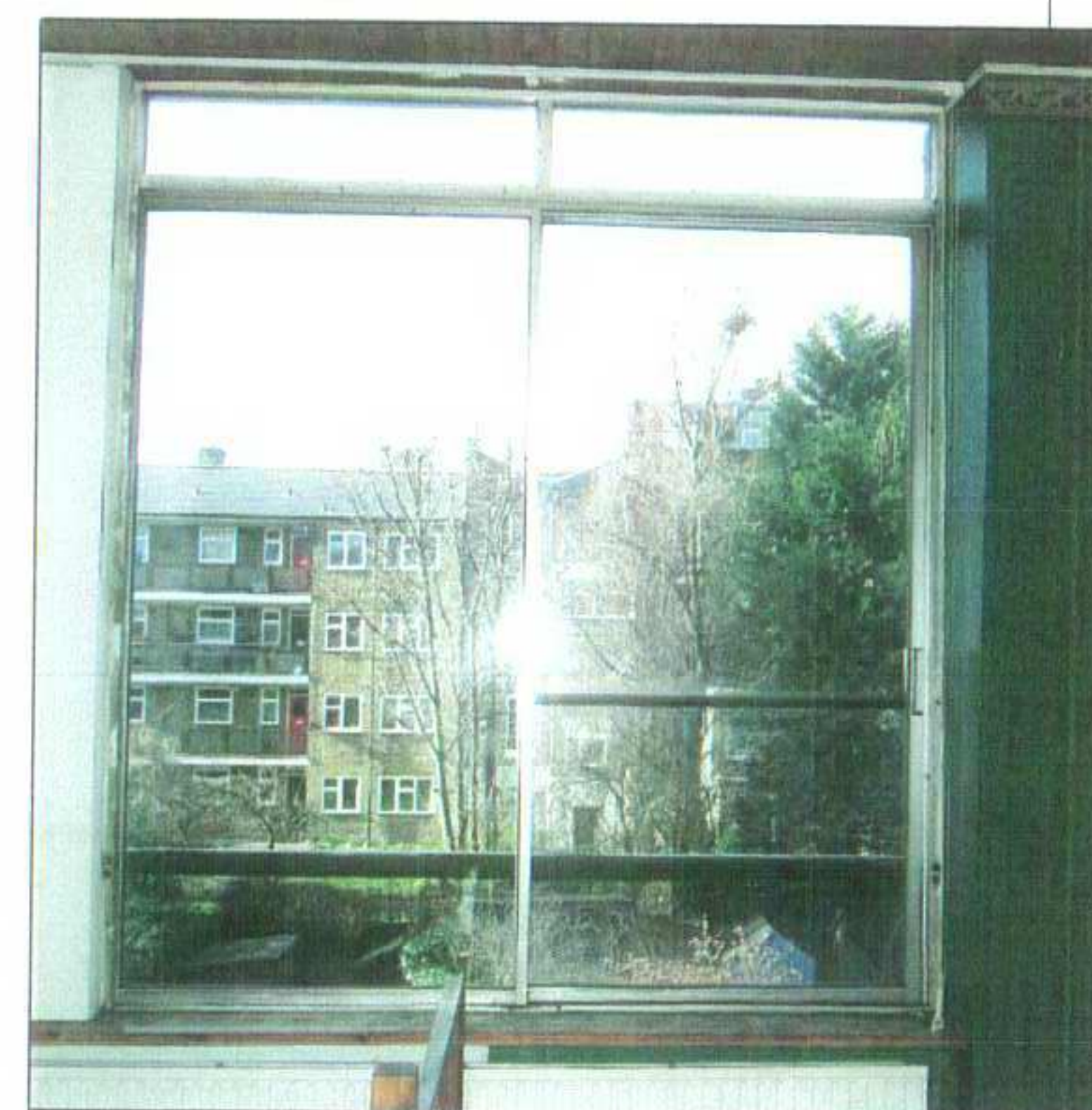
Large metal framed window to be replaced by two timber framed sliding sash windows to line up with windows below and to match existing. This is due to proposed new partitions within the space conflicting with the existing window. This will also enhance the aesthetic of the rear elevation.
