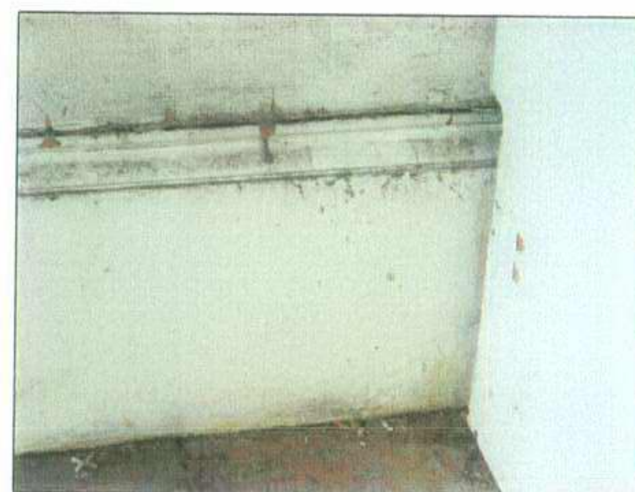
Skirting in existing ground floor kitchen to be replaced with square edge softwood skirting with 5mm chamfer
