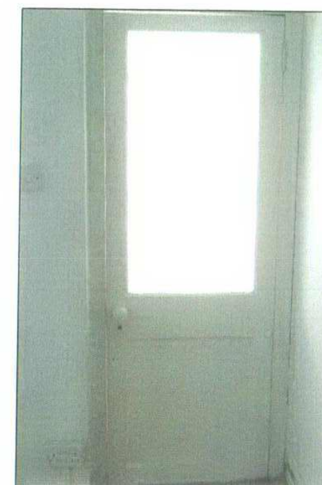
Existing door to basement WC to be replaced with standard door blank with painted finish and painted softwood standard architrave. Stainless steel door handles.
