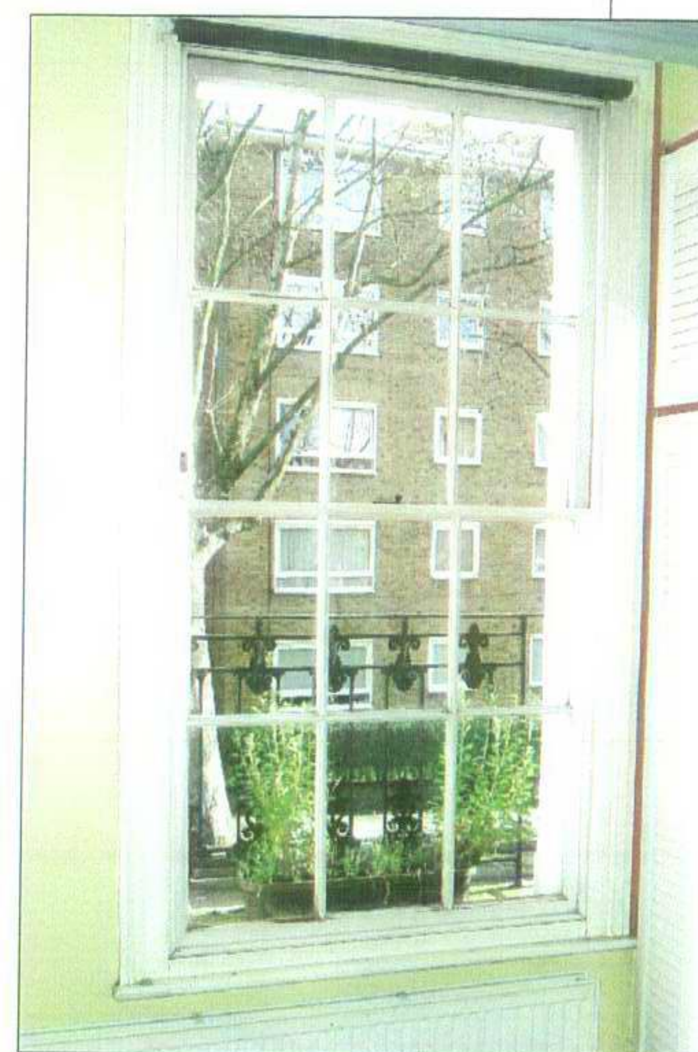
Windows to be replaced with new timber framed sliding sash windows to match existing. All to be double glazed
