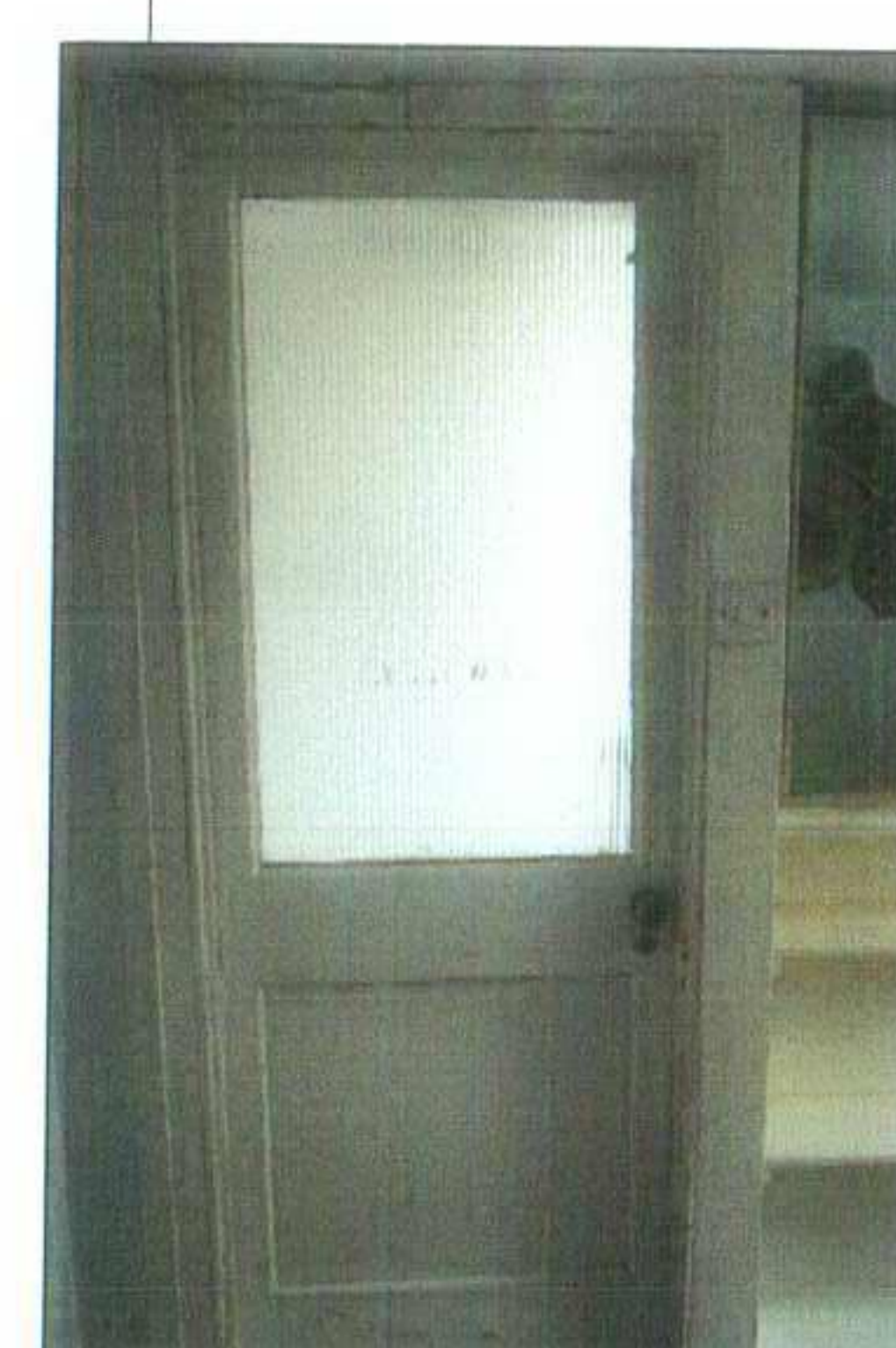
Existing door to basement WC to be replaced with standard door blank with painted finish and painted softwood standard architrave. Stainless steel door handles.
