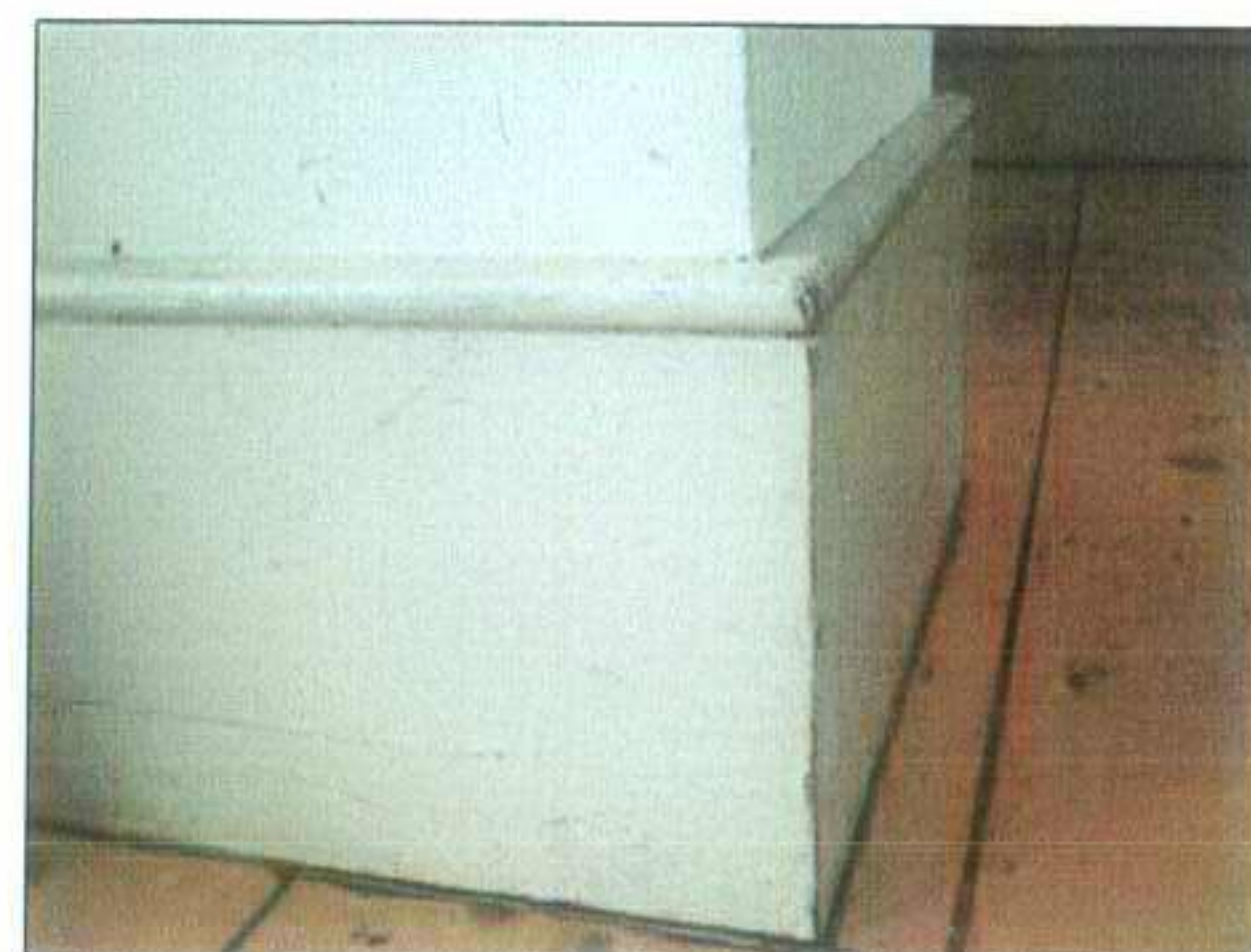
Skirting in existing ground floor dining to be replaced with square edge softwood skirting with 5mm chamfer
