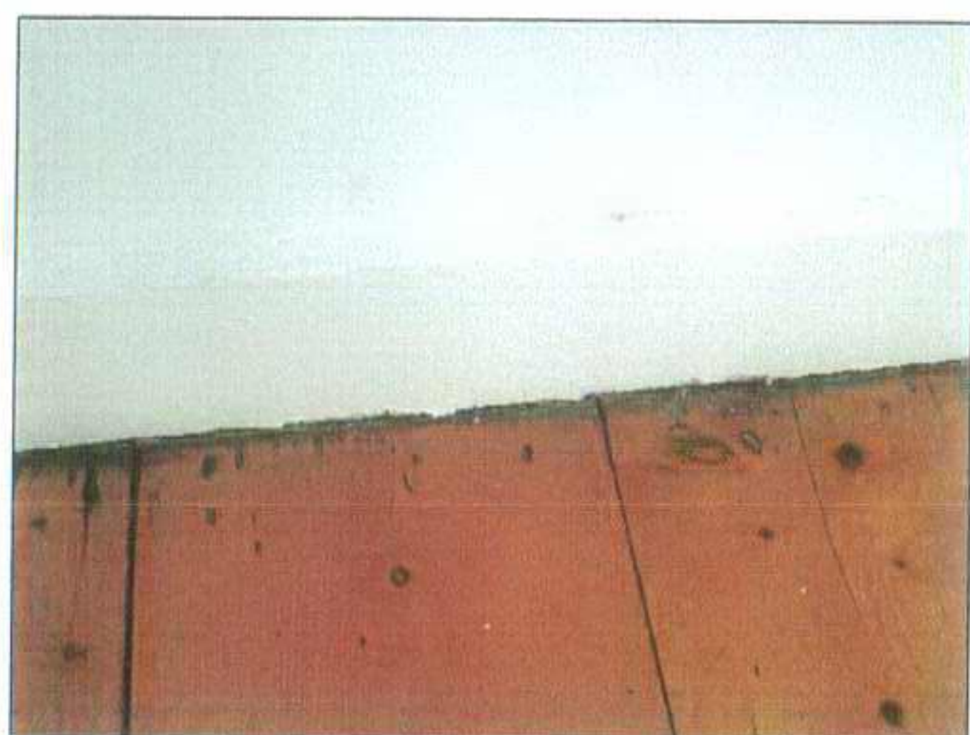
Existing skirting to be replaced with square edge softwood skirting with 5mm chamfer
