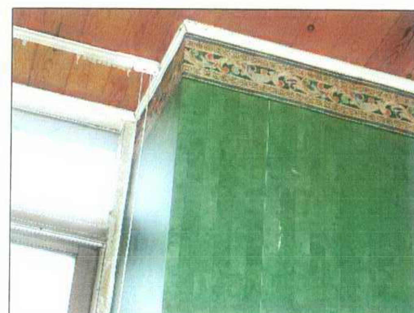
Cornicing to be removed as it conflicts with proposed new room layout and partitions
