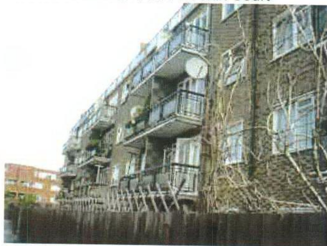
Rear Elevation to 1-39 Phoenix Court
