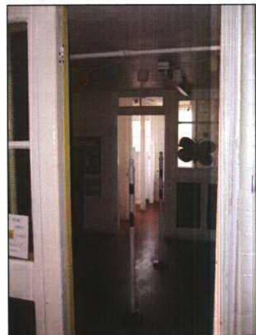
Toilet partition to be removed
