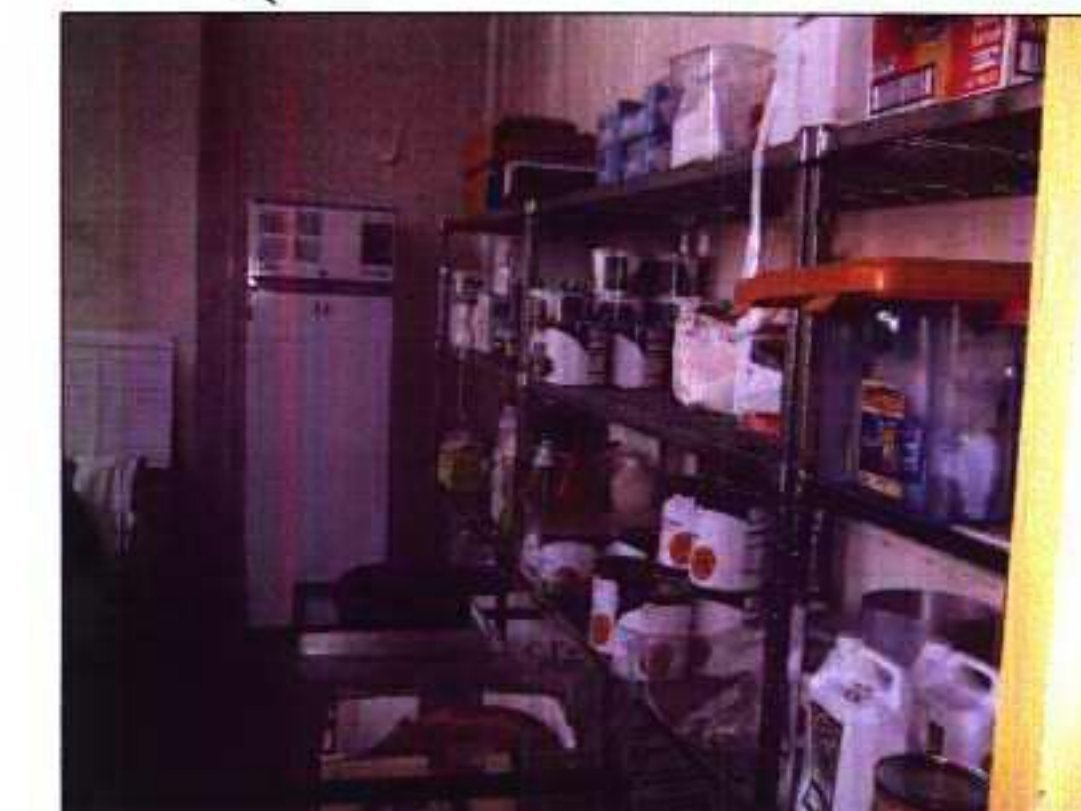
Modern partitions in Kitchen Store to be removed to make way for new Classroom
