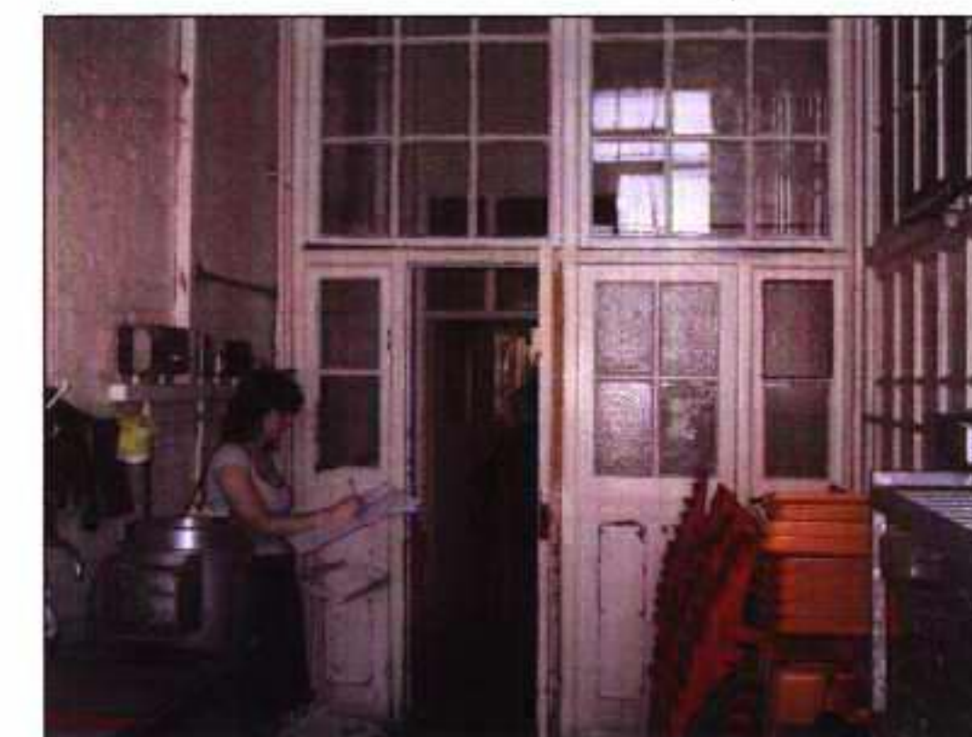
These screens to be removed to make way for new Classroom
