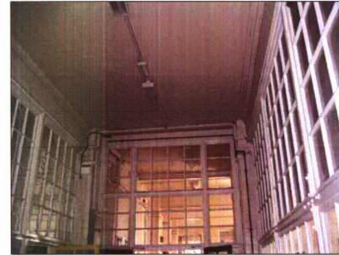
Door & screen between Corridor and Hall - new Lobby to be created here
