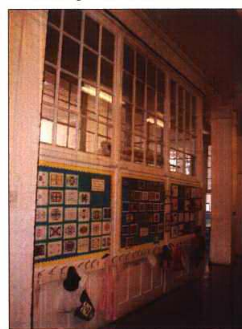
Store room glazed screen to be removed
