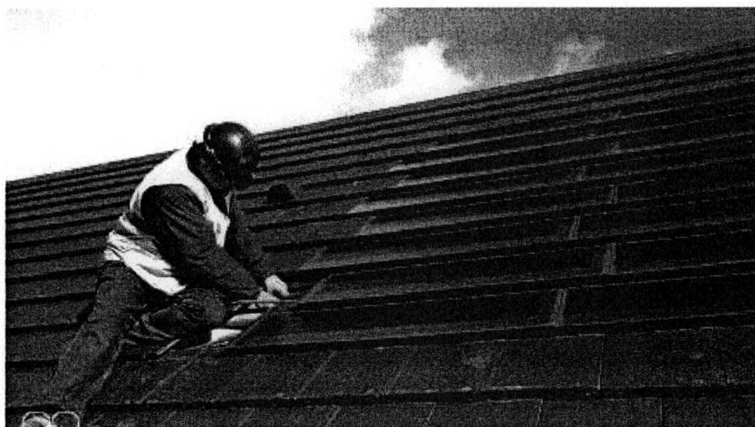
Figure 5.3 - Solar Tiles combining PV and Solar Hot Water.
