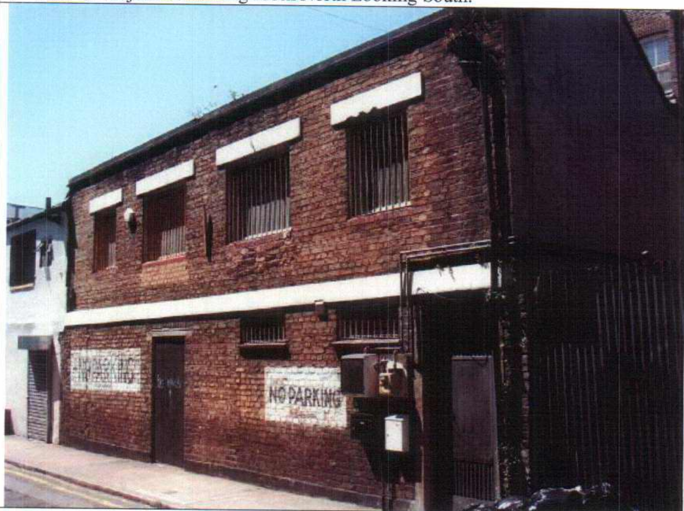
8- Front Face Of Adjacent Building Taken From Wolsey Mews.
