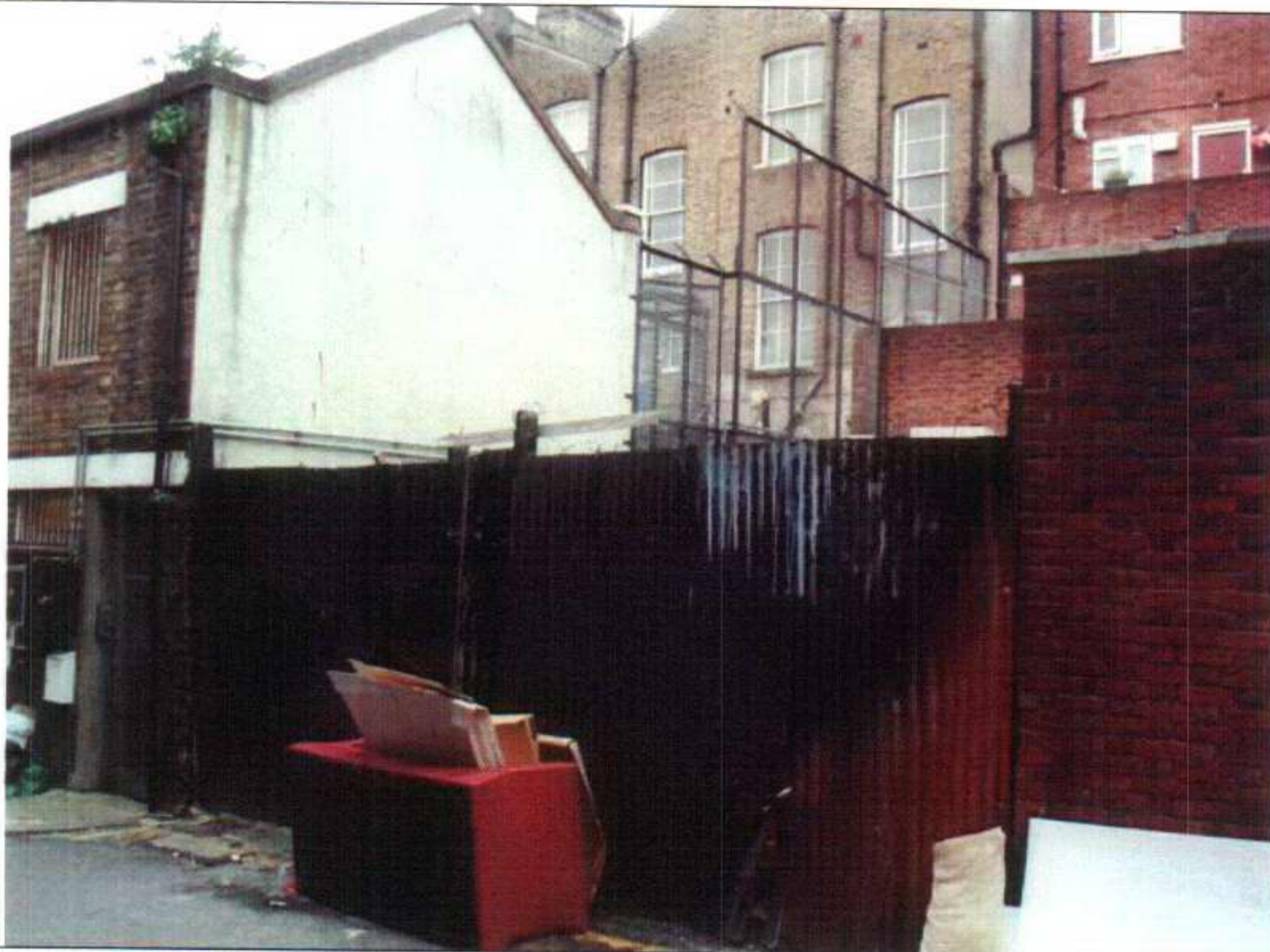
3- Front View Of Site With Adjacent Building Visible.
