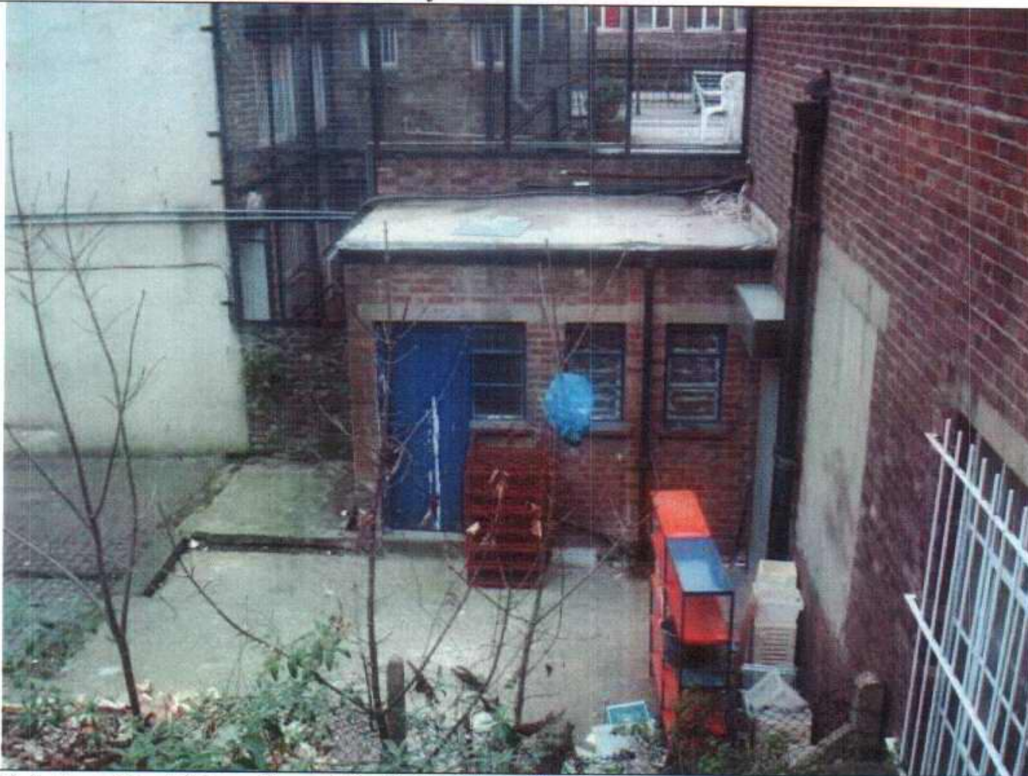
2- Existing Site Taken From North looking South.
