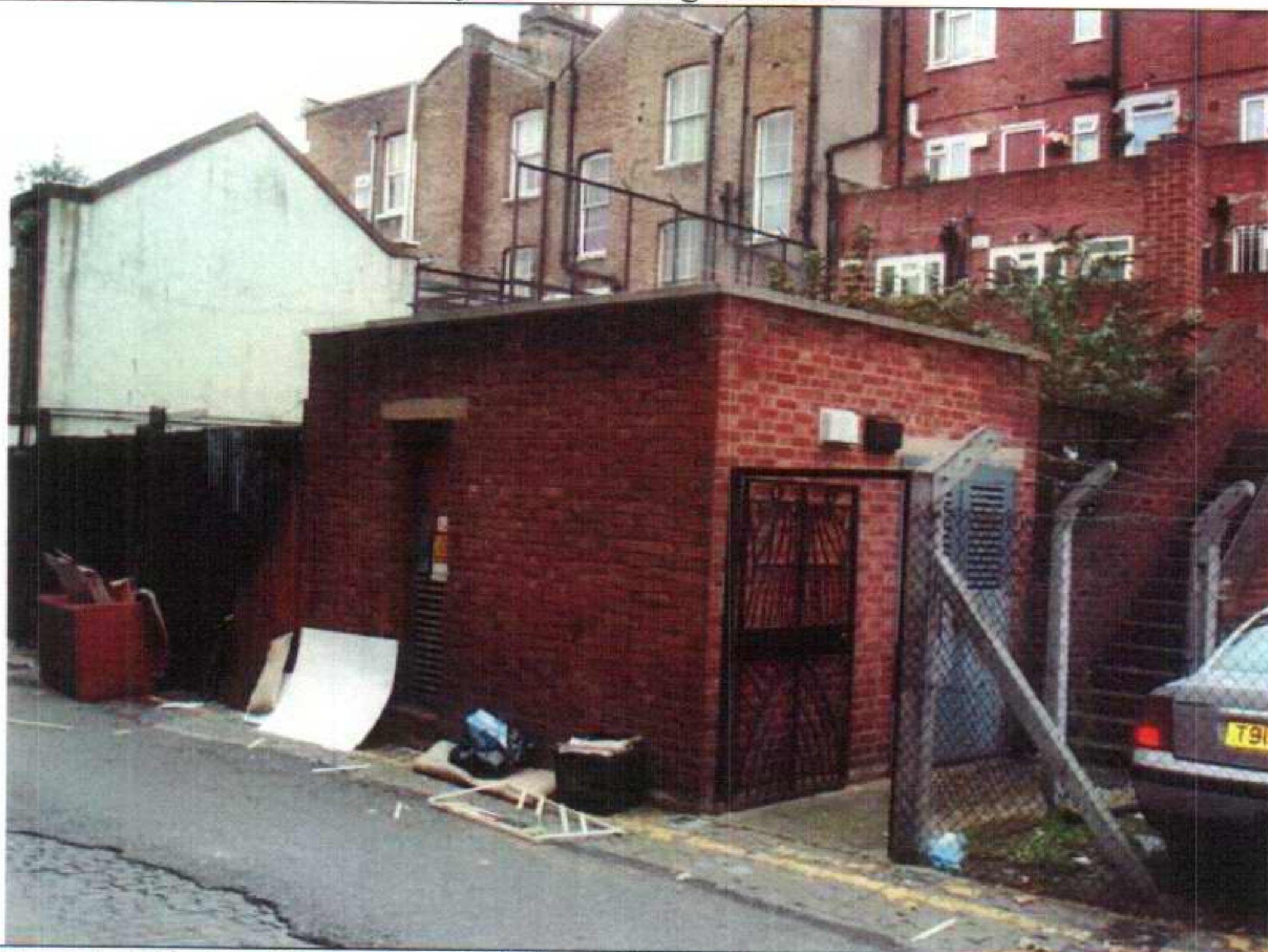
4- Electrical Substation on North Side of Site.
