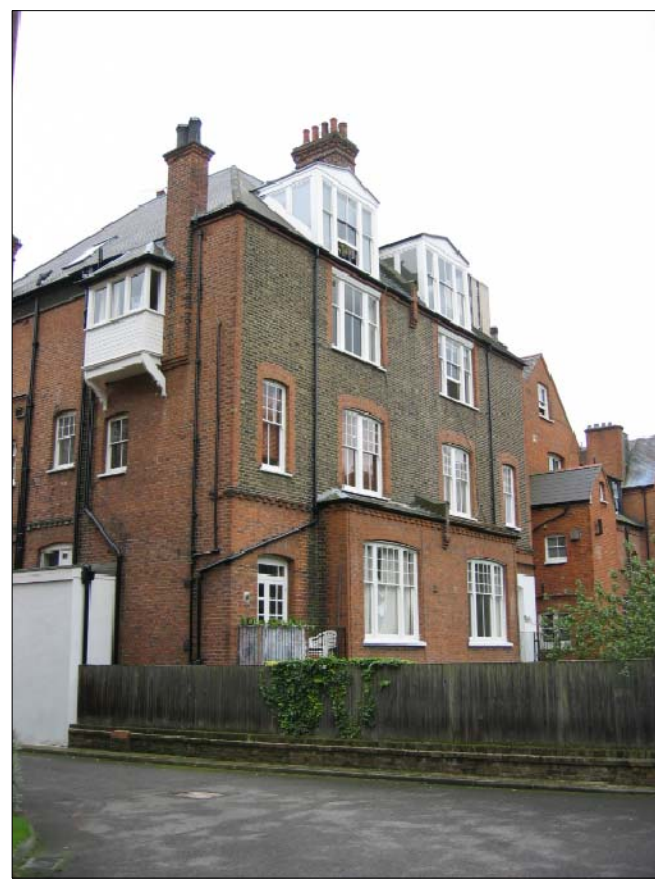
View to rear elevation
