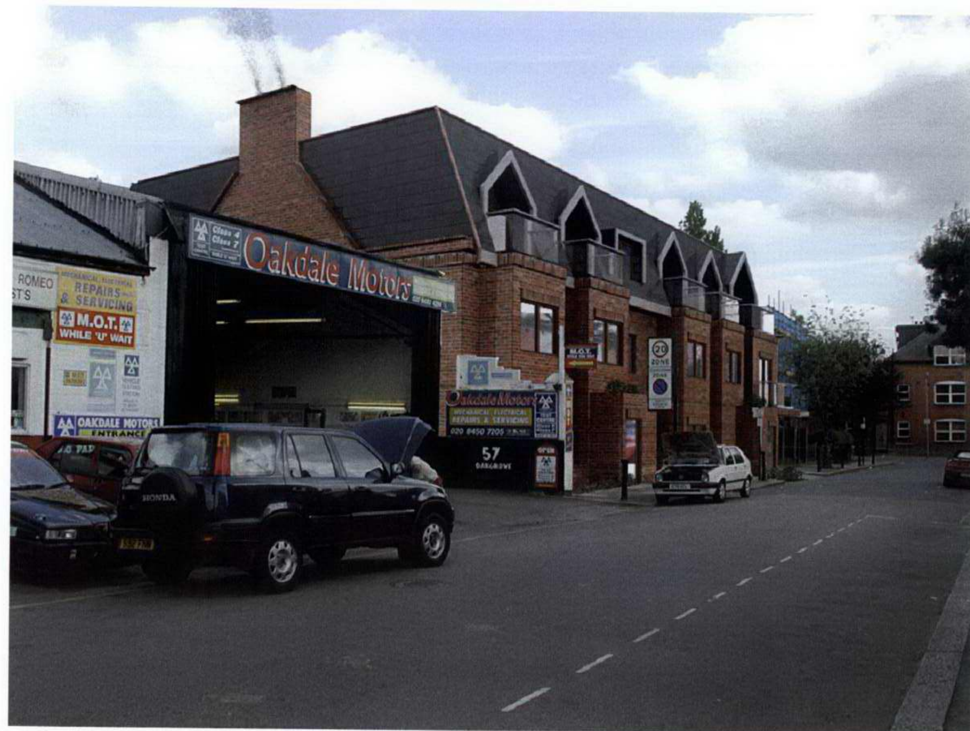
View from the West
