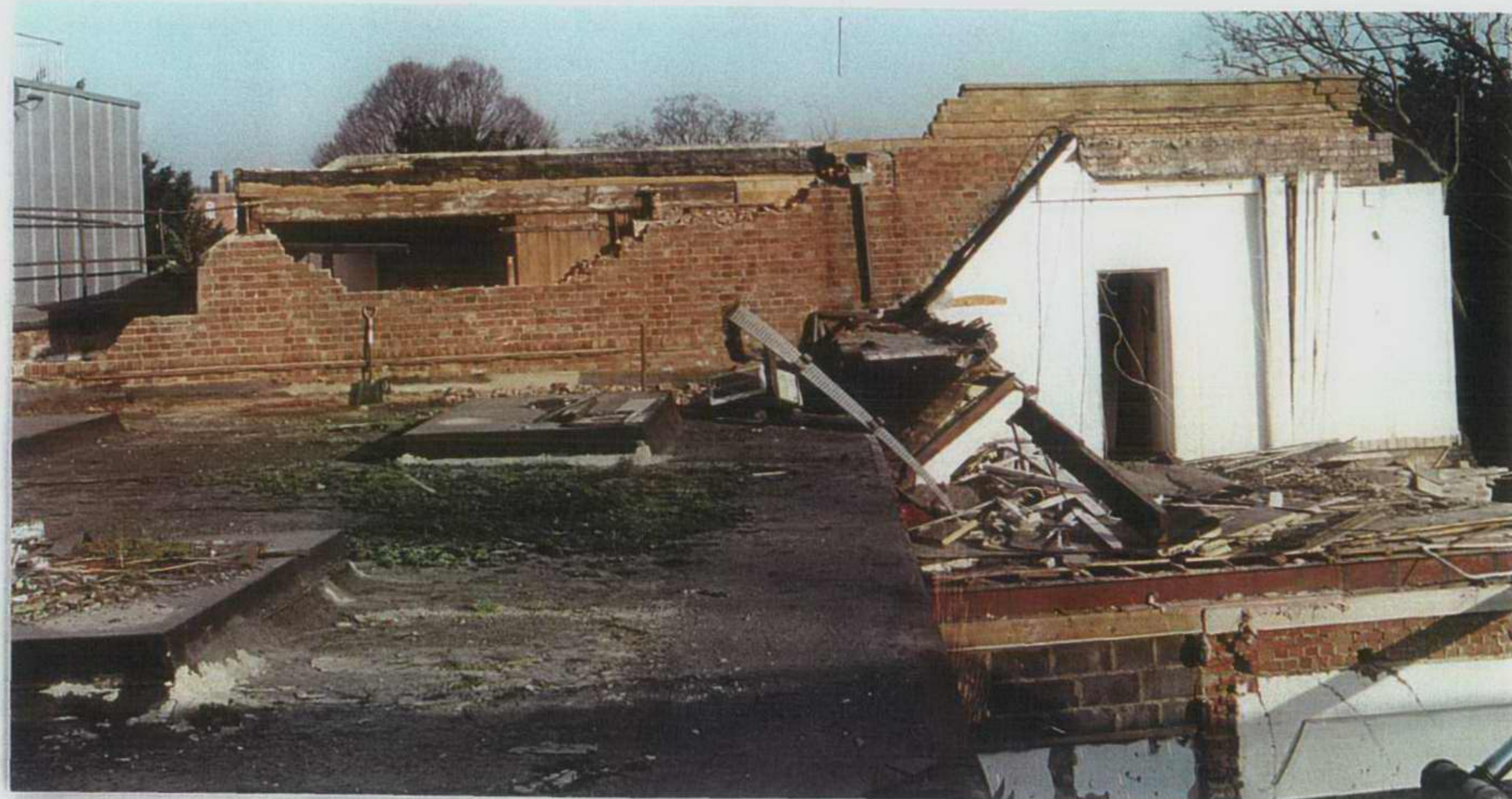
Rear of Property NO 1-2 Grangeway (Being demolished)
