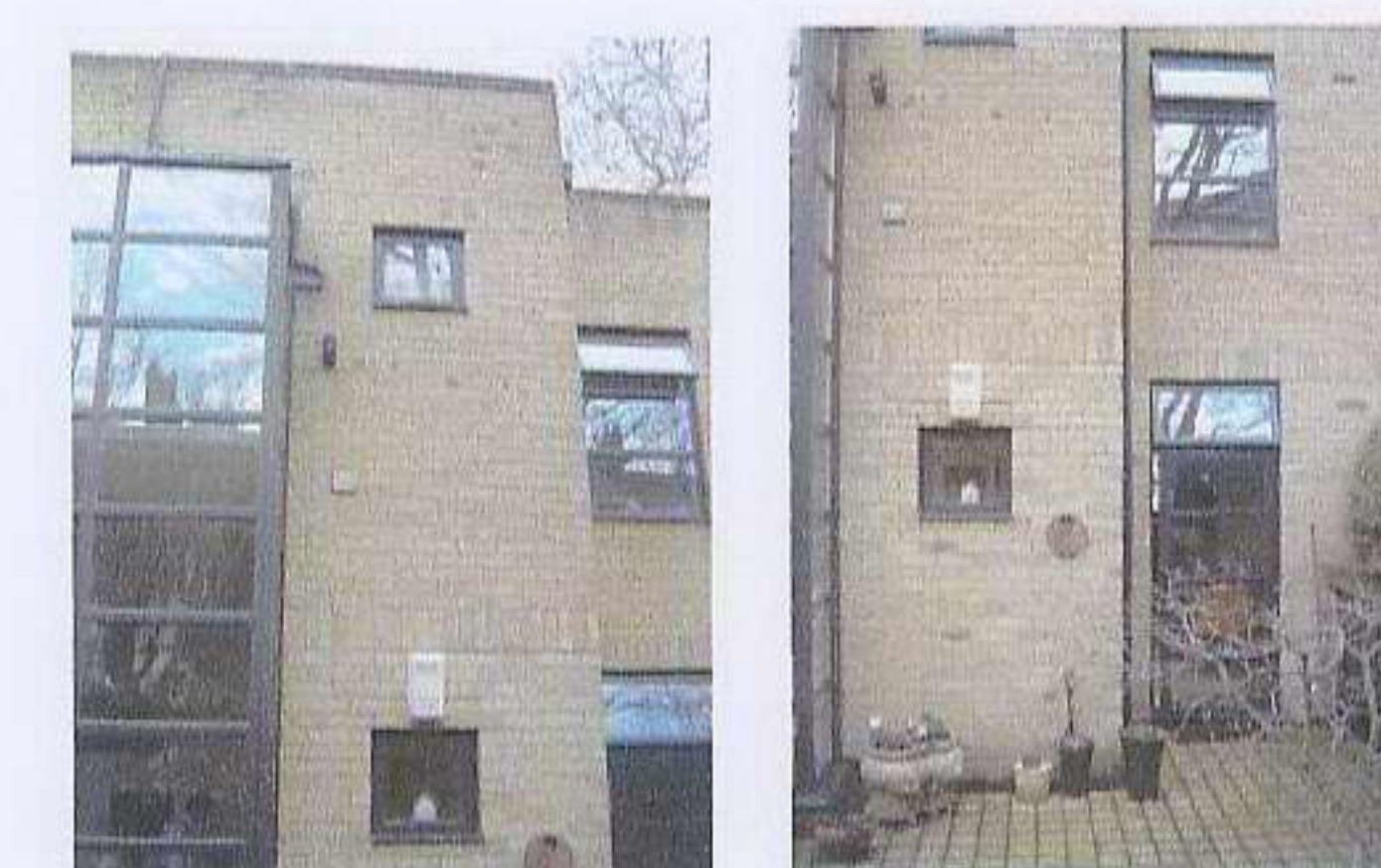
view of rear of property
