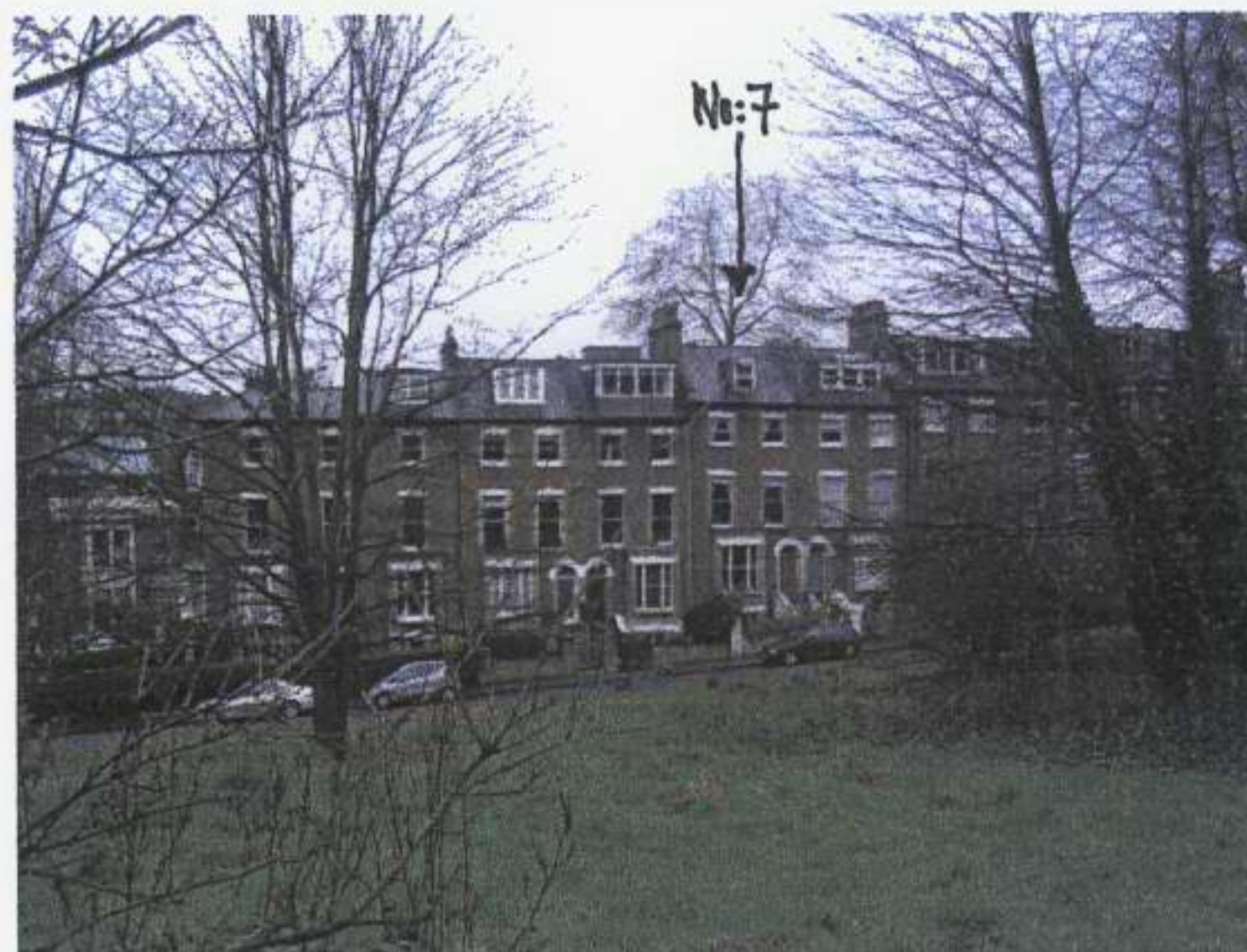
GENERAL VIEW FROM HAMPSHIRE HILL PHOTO 2
