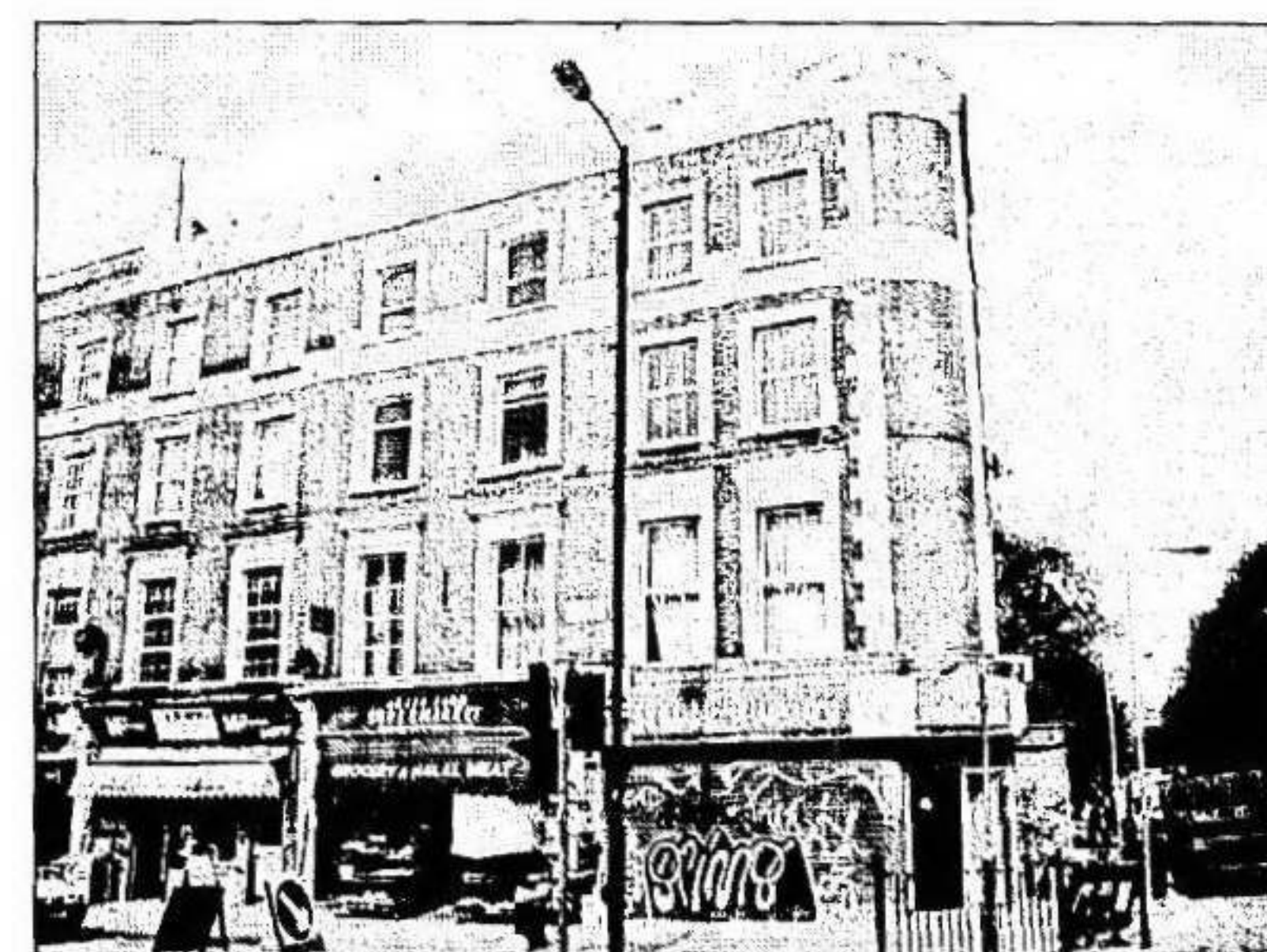
10. ADJACENT CORNER (YORK WAY)
