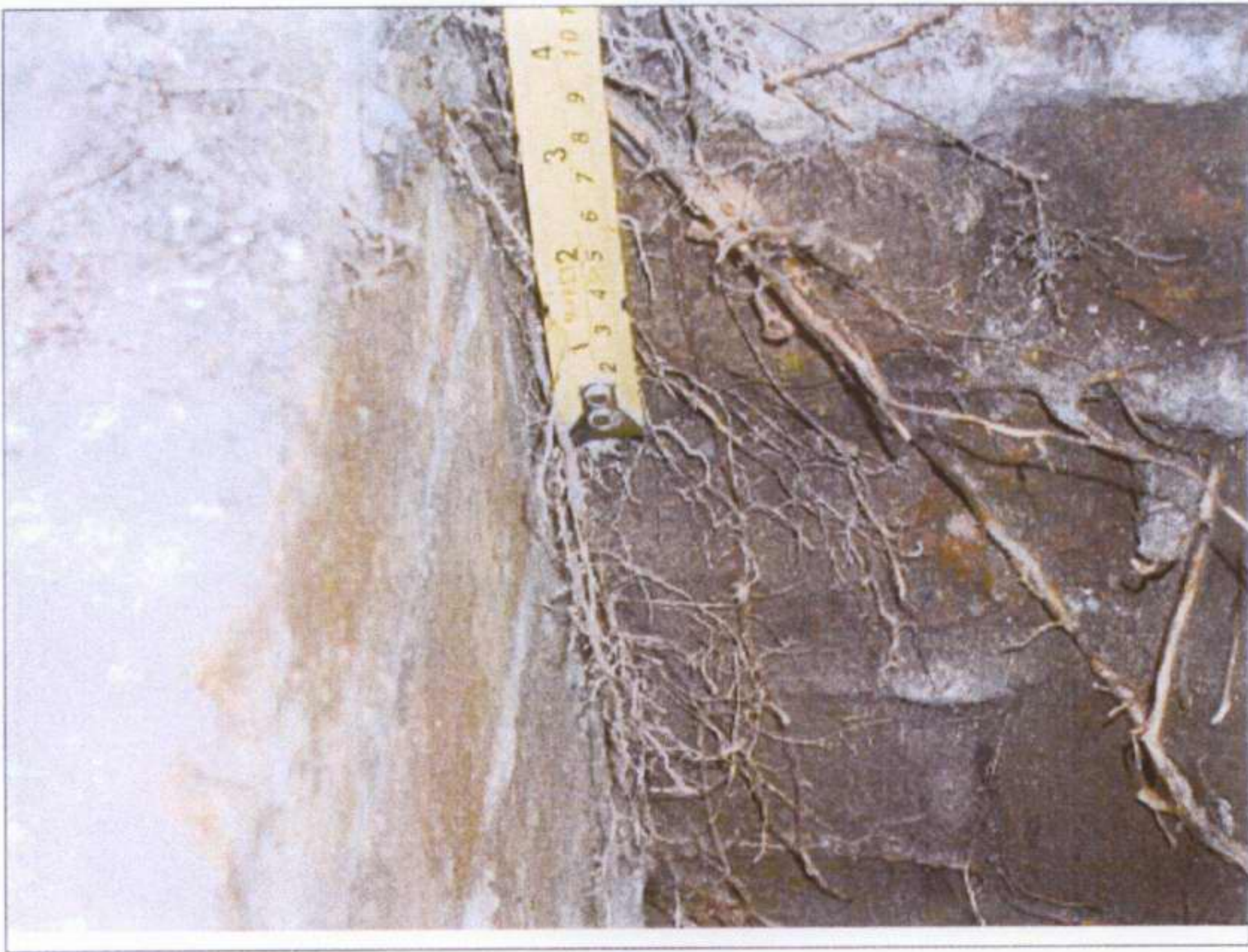
Figure 5 - Close up showing fibrous and woody roots up to a maximum of 6mm diameter.
