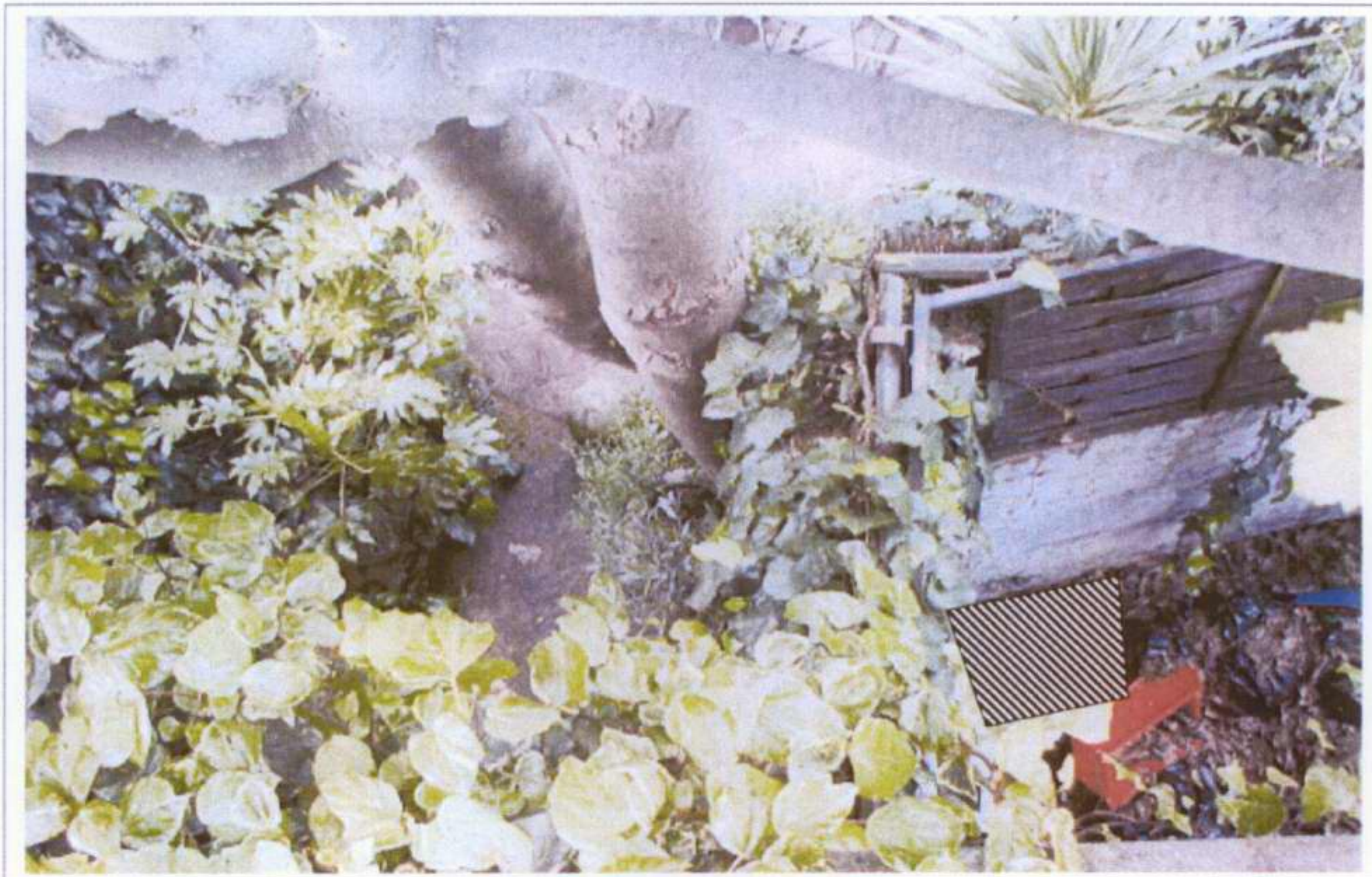
Figure 3 – Stem and base of tree looking down from roof of existing building. Stem of tree at 4.5 metres is 0.5 metres from wall. Trial pit is shown hatched.
