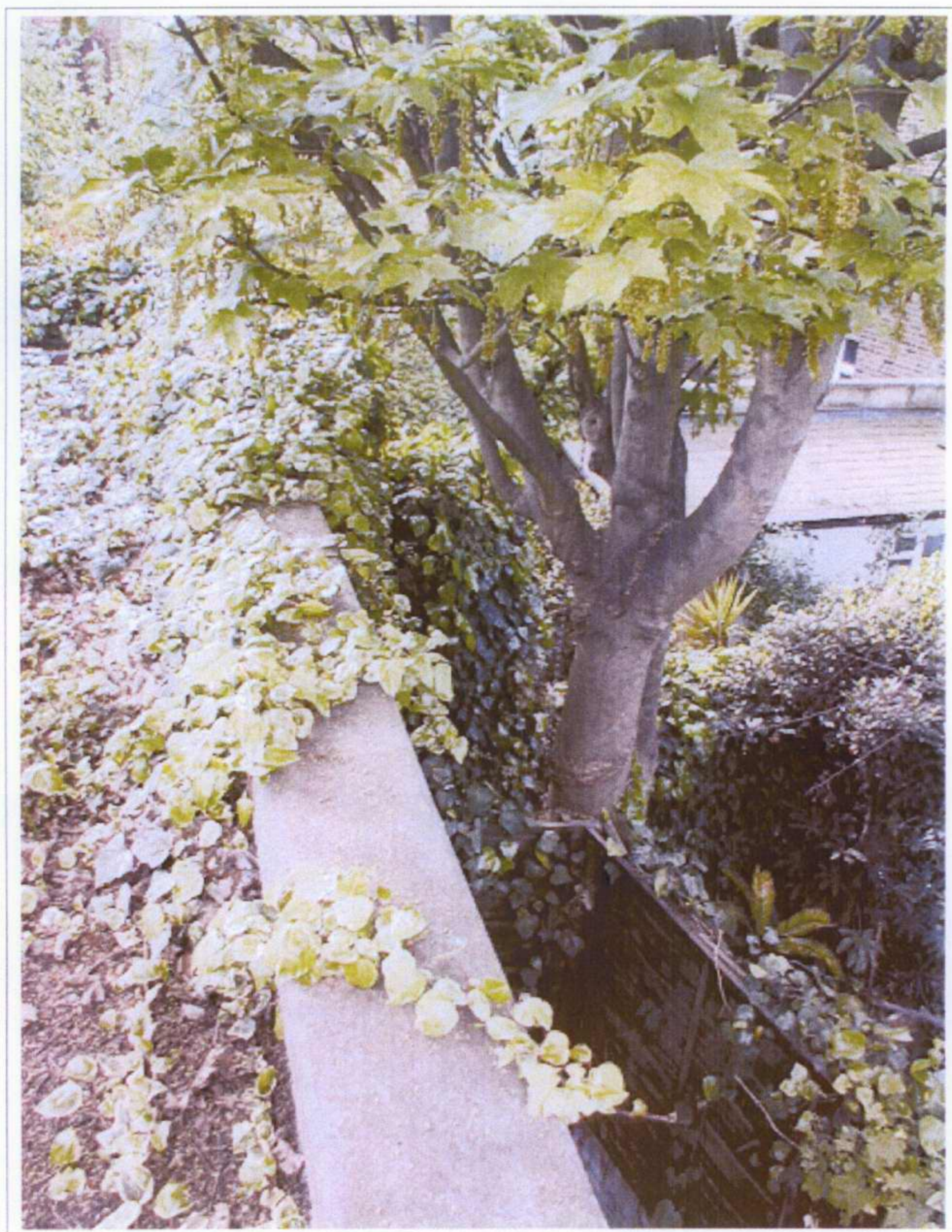
Figure 1 – Canopy overhangs site by 3.5m maximum but there is no direct contact with wall.
