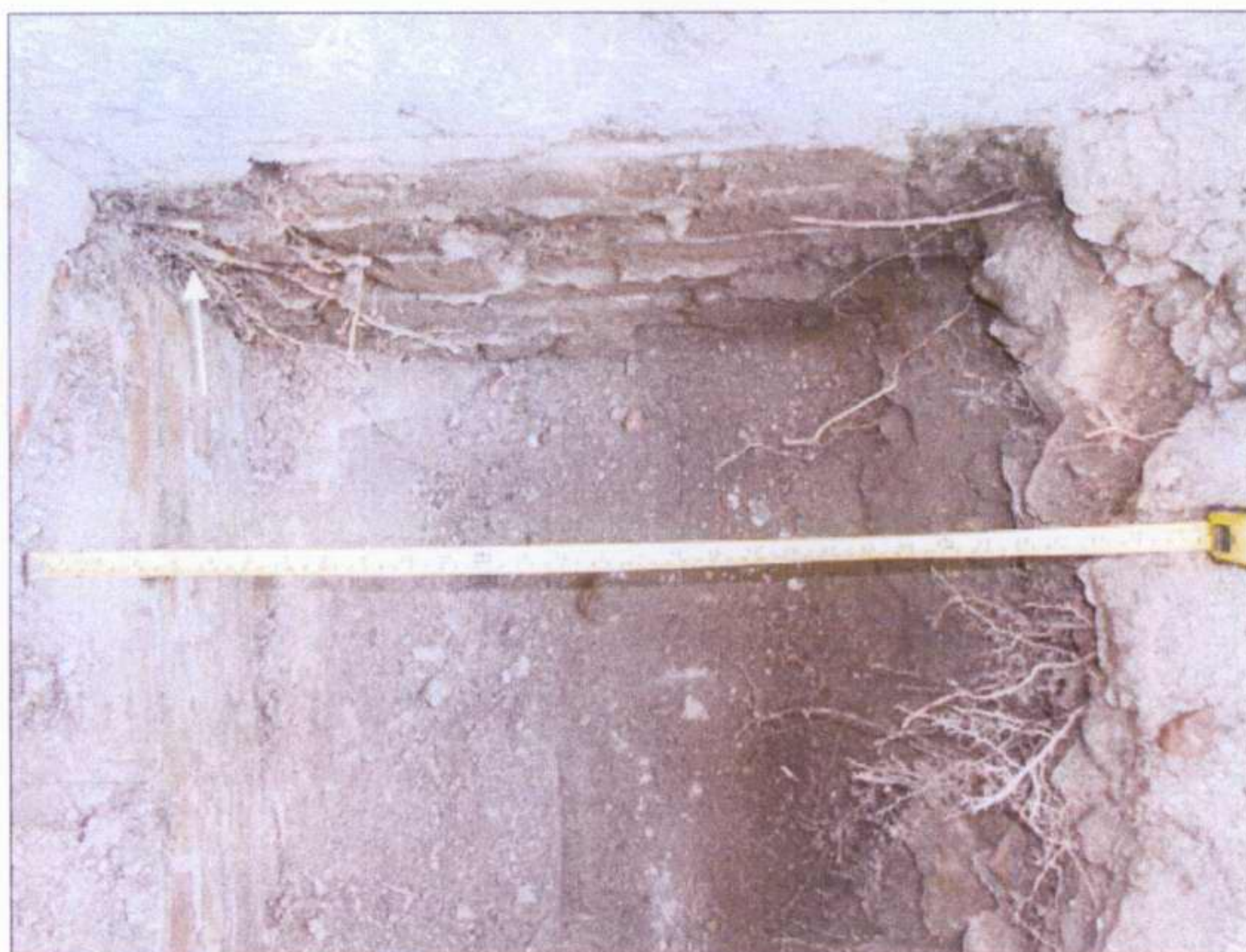
Figure 4 - Extent of root penetration limited to intersection of walls (arrowed)
