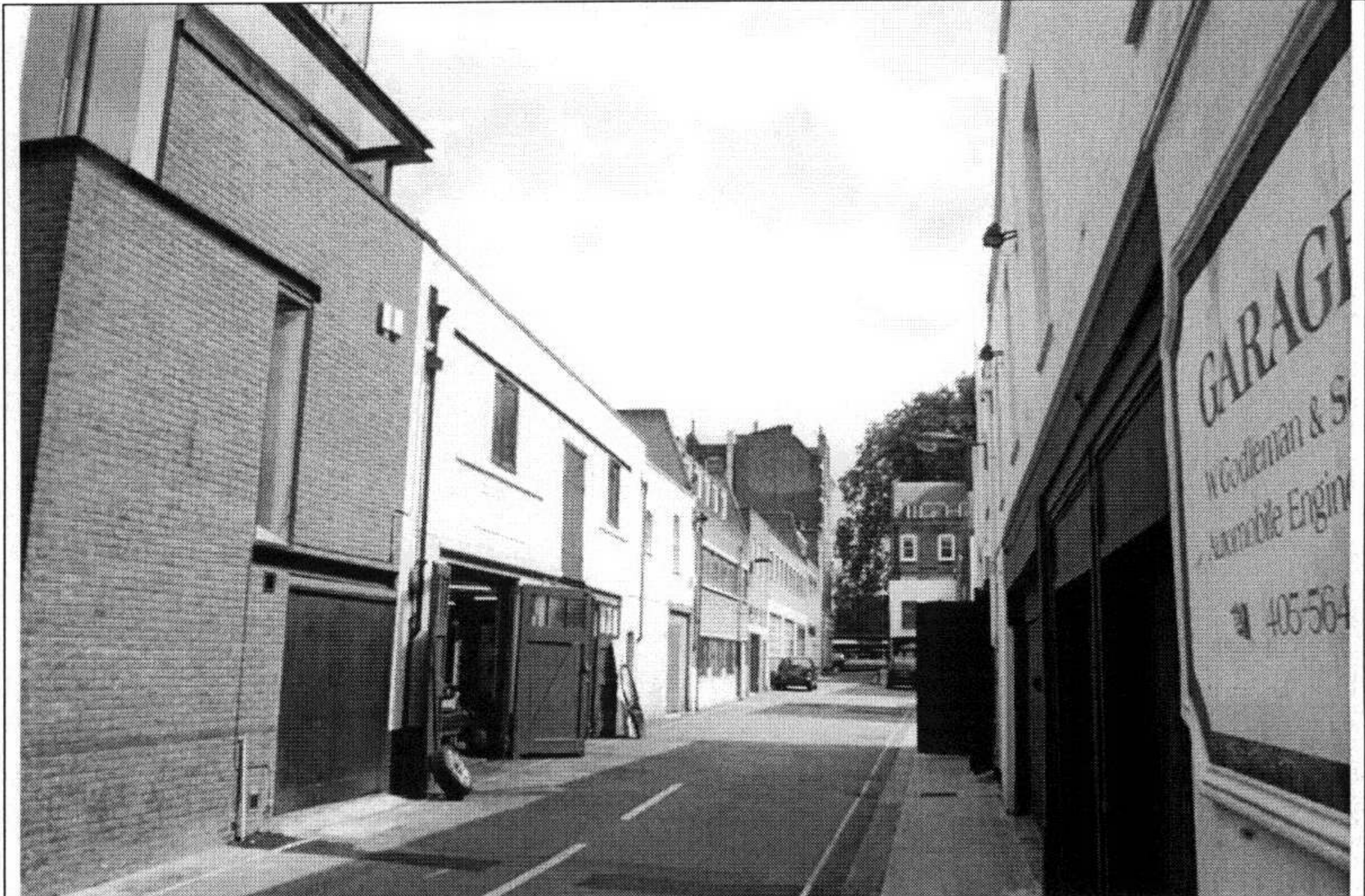
Existing view of 22-30 Kings Mews. View from north.
