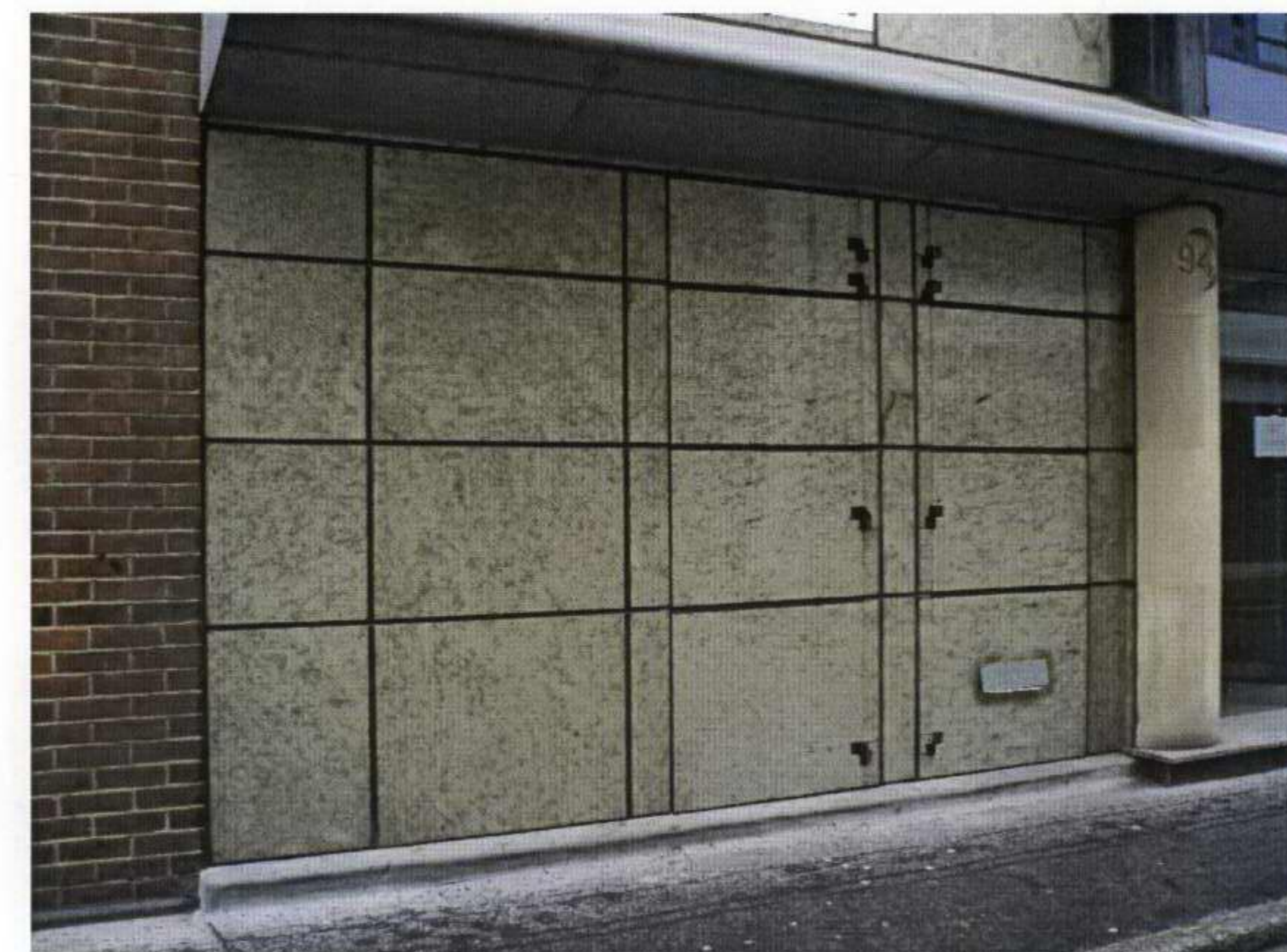
Cladding Adjacent to Saffron Hill Entrance
