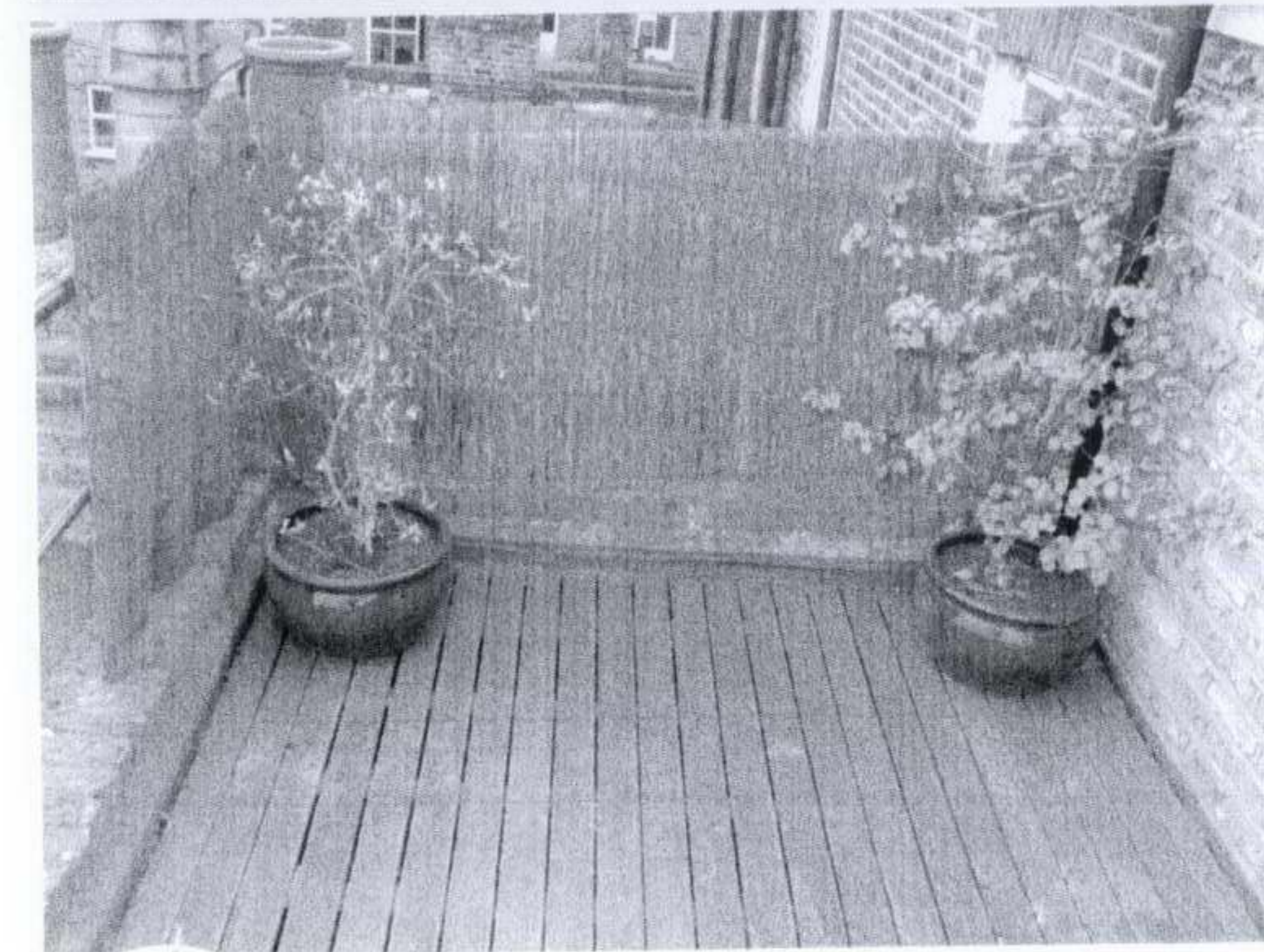
terrace 2 @ second floor level.
