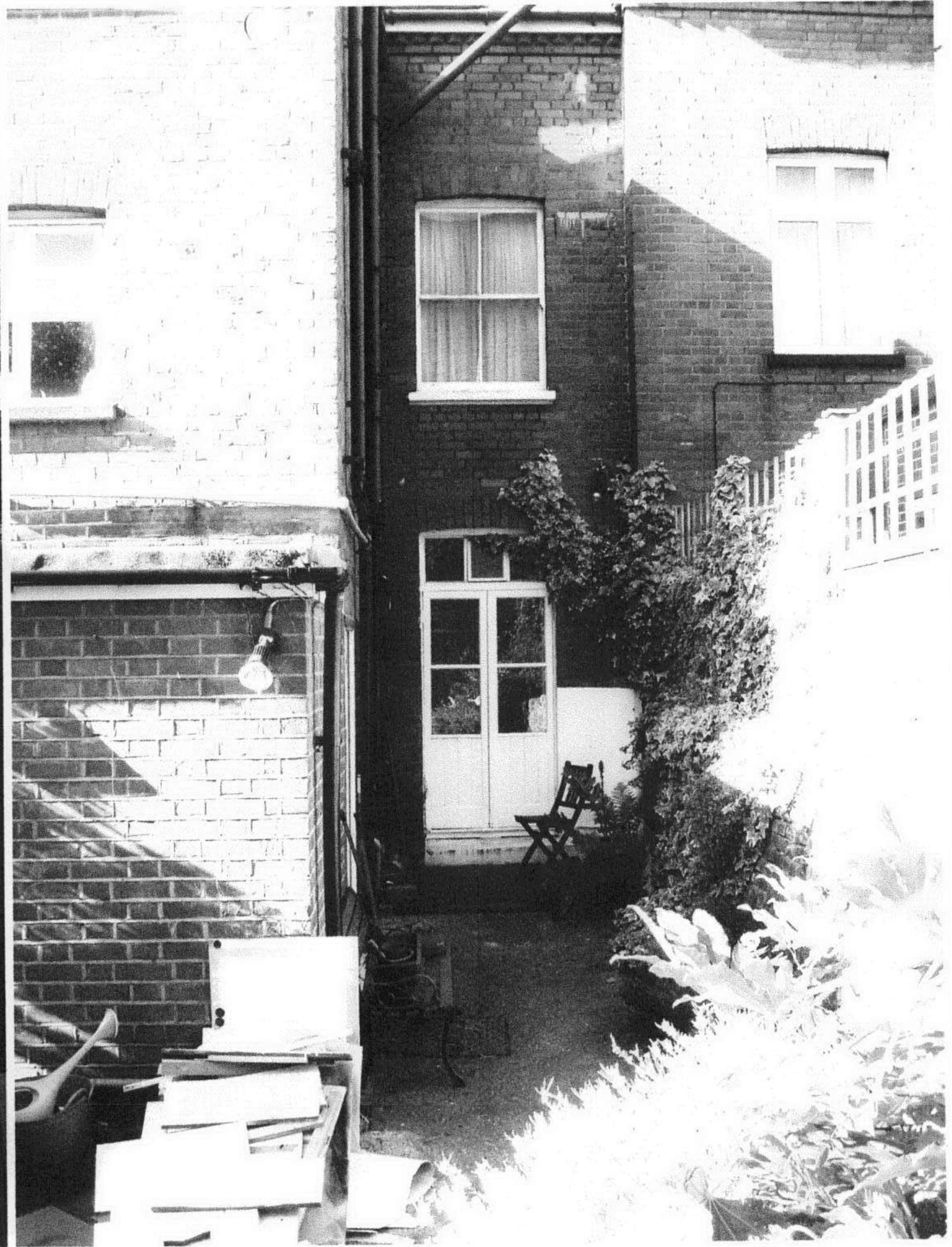
EXISTING REAR AREA
