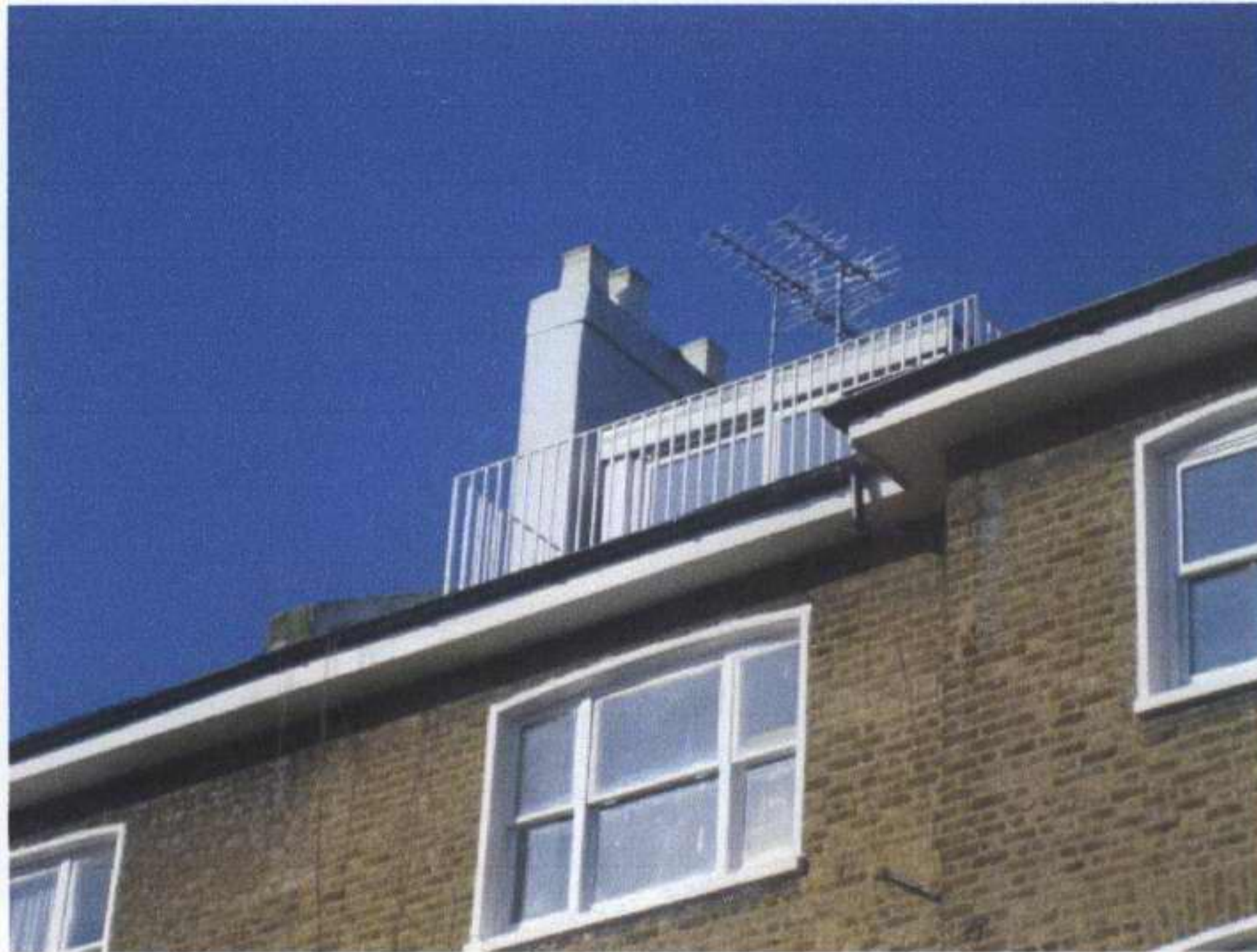
Rear dormer to no. 63 adjacent
