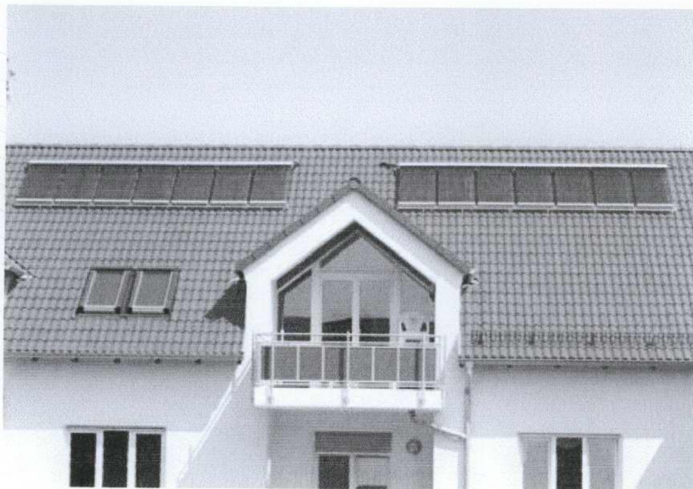
14 collectors for solar water heating and solar heating support for a multi-family apartment building.
