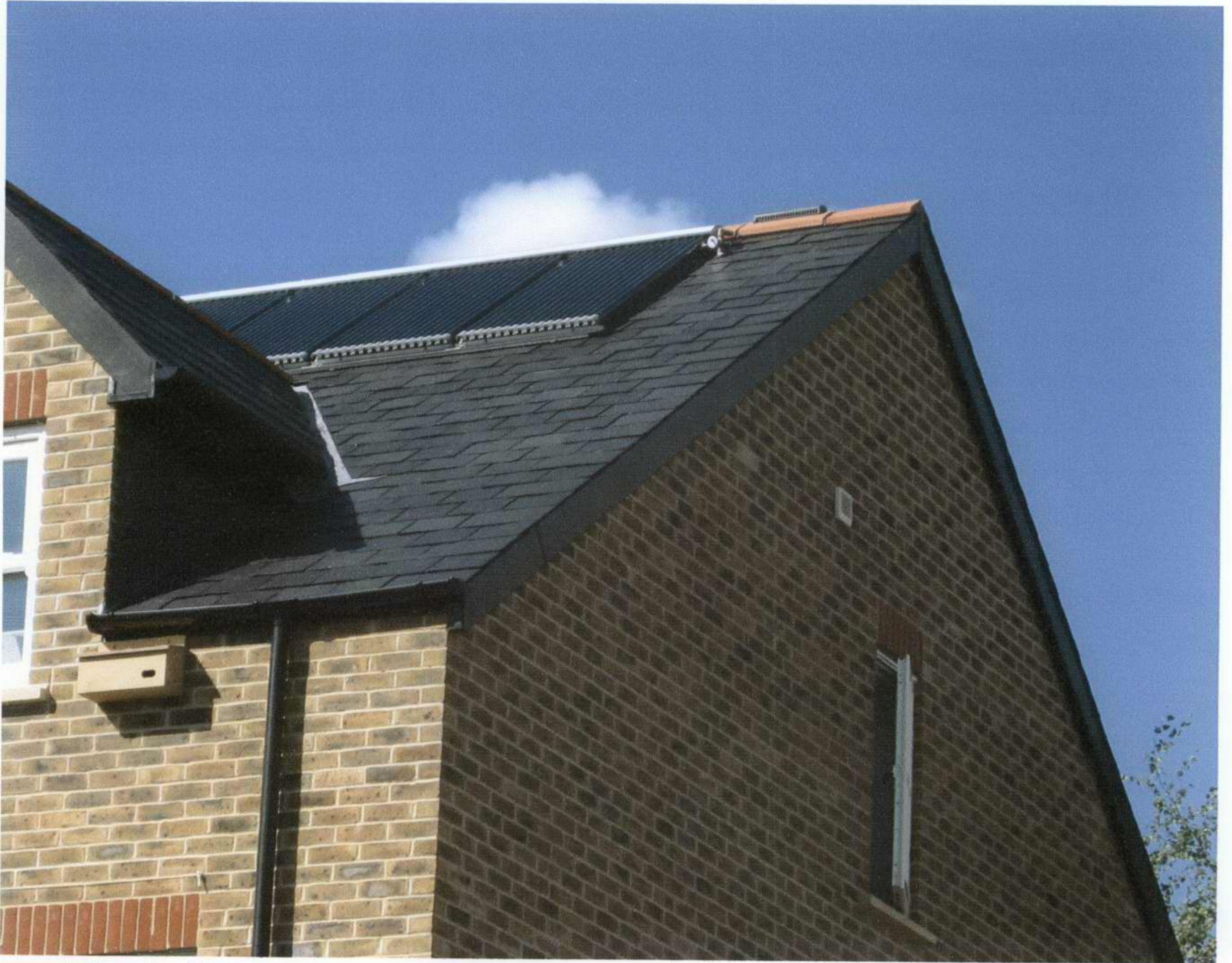
Image 5: Example of Schott Solar Thermal panels installed.
