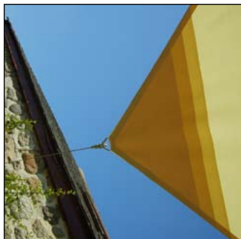
Tensioned wire with rigging screw & corner detail.
