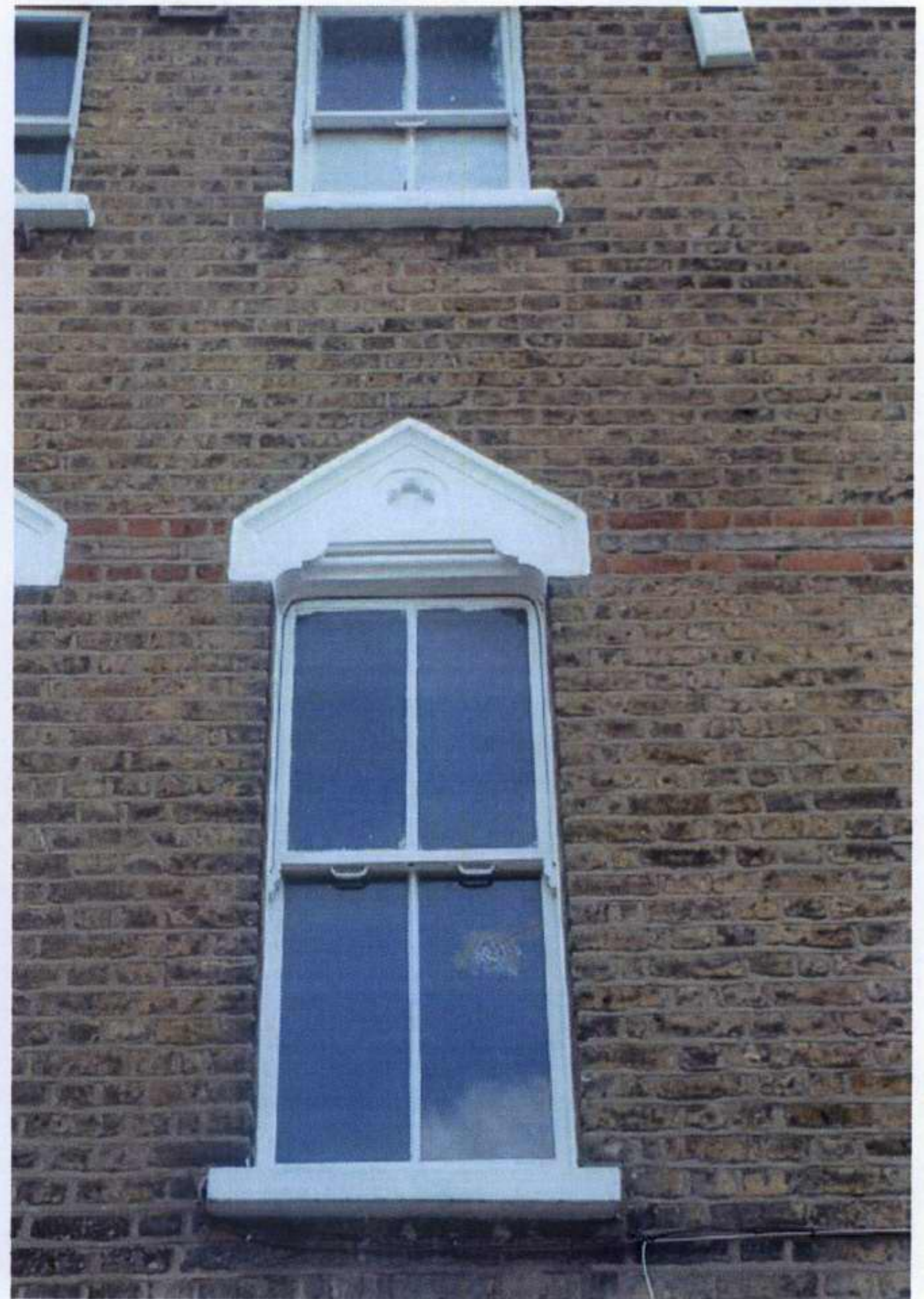
Photo 2: First Floor Window - Front Elevation
