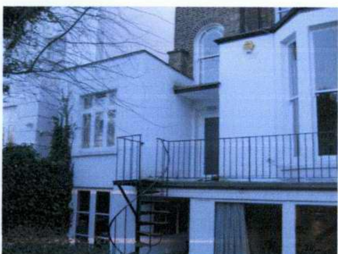
Rear return and basement level extension.
