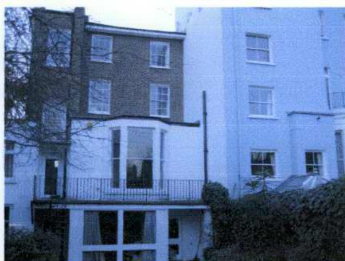
Historic bay window to hall floor level
