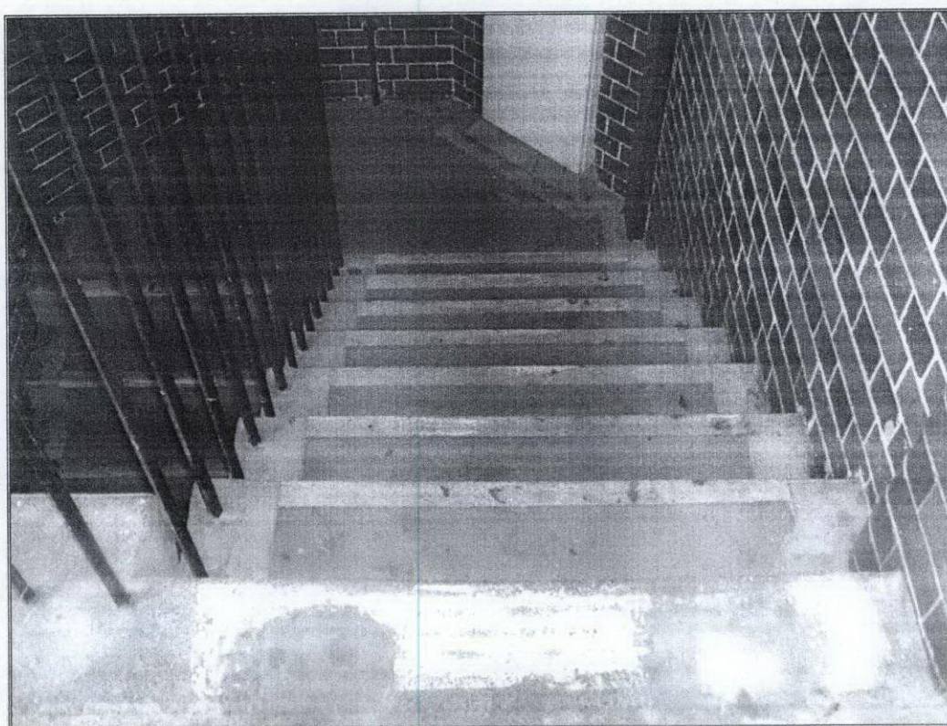
Photo 2 – Typical example of the existing 'Tor' coating to the treads within the staircases.
