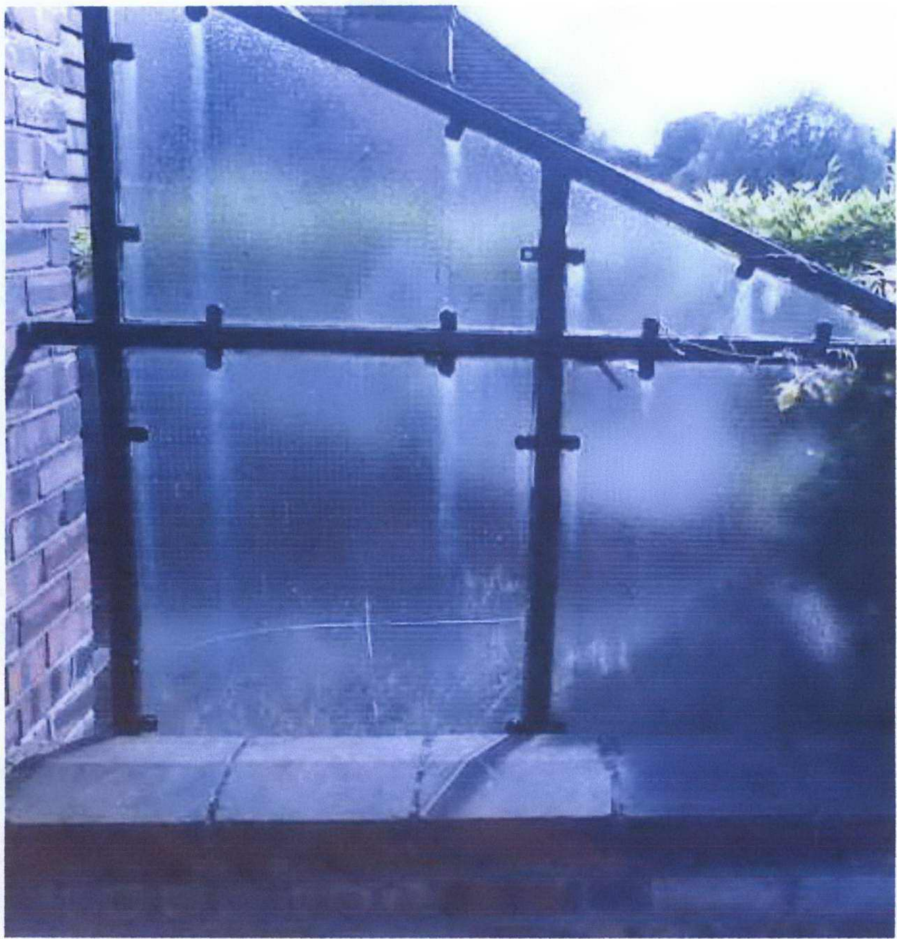
PARTY WALL & SIDE OF NEXT DOOR NEIGHBOURS ROOF TERRACE (NO. 30) PHOTO TAKEN FROM MY FLAT ROOF (31)
