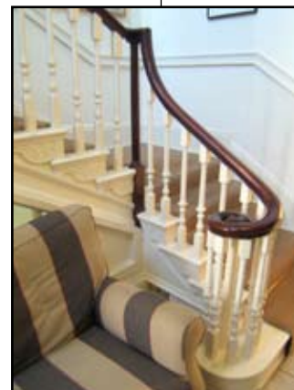
Original stairtreads and balusters
