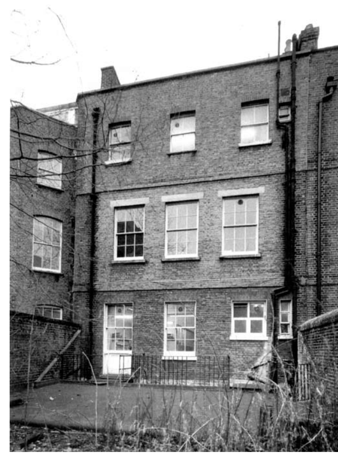
Photo from 1973, showing the 3rd floor of No. 34 rebuilt, left. No. 35 has stone or concrete lintels on the first floor, and a much altered ground floor.
