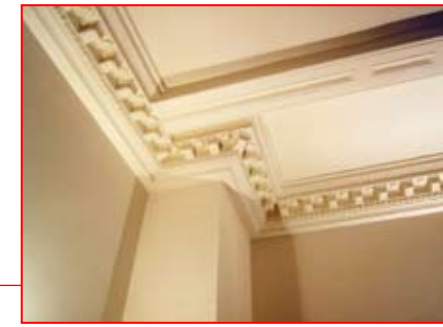
Modern cornice (copy) routed around services box
