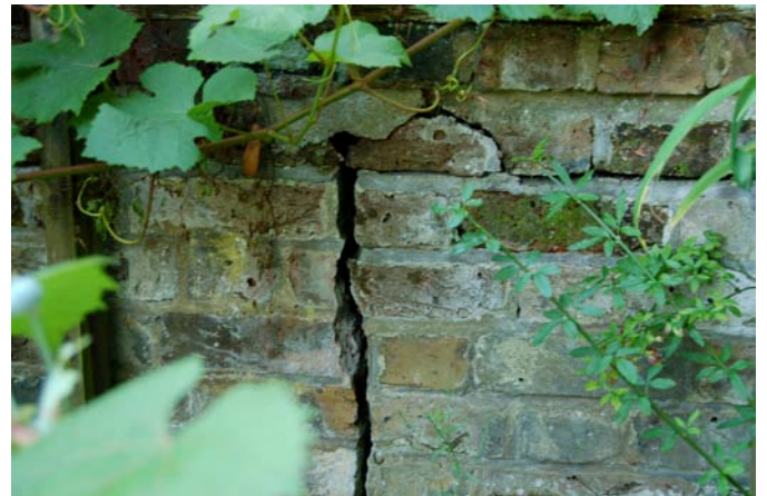
5. cracking caused by subsidence to garden terrace
