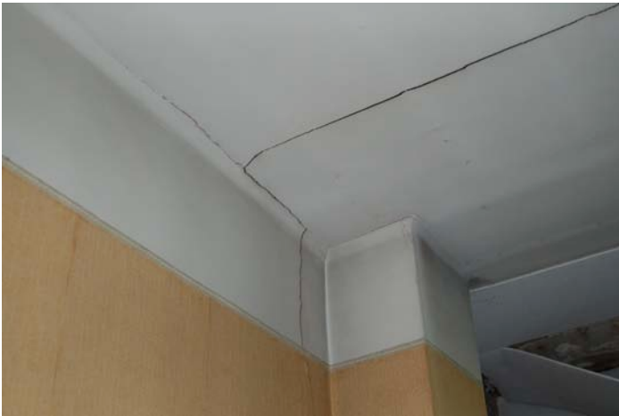
1. cracking caused by subsidence to rear ground floor
