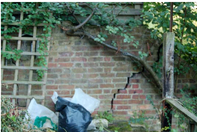
4. cracking caused by subsidence to garden terrace
