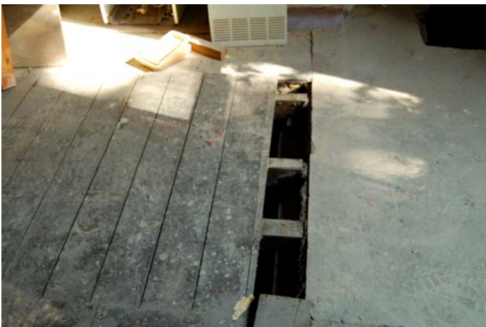
3. heave caused by subsidence to front basement
