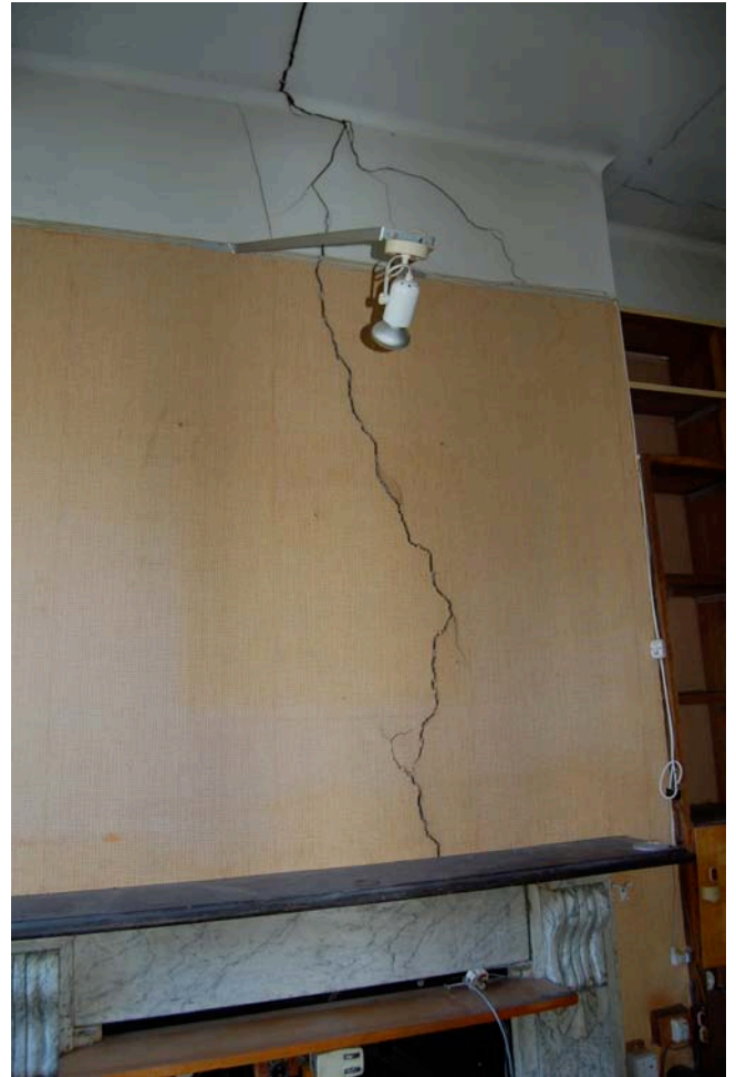
2. cracking caused by subsidence to rear ground floor
