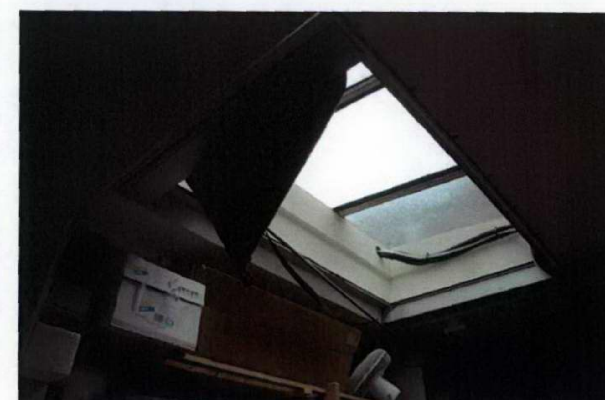
9. Roof light rear room
