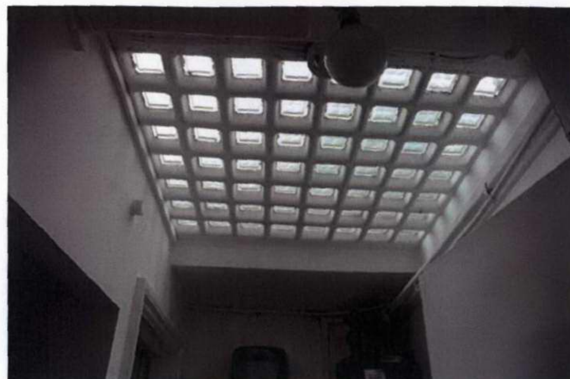
1. Under entrance pavement vaults
