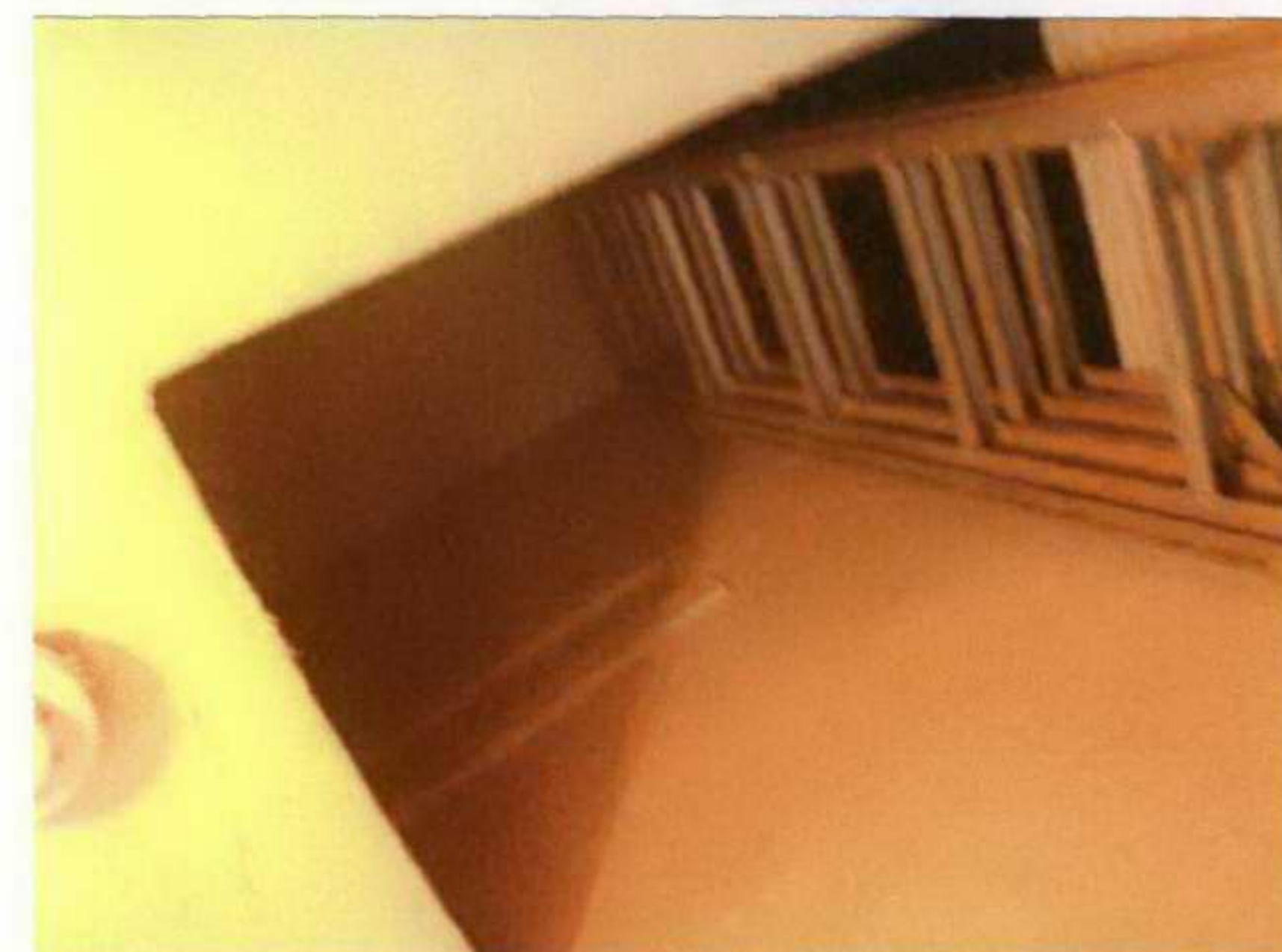
8. Access hatch to roof
