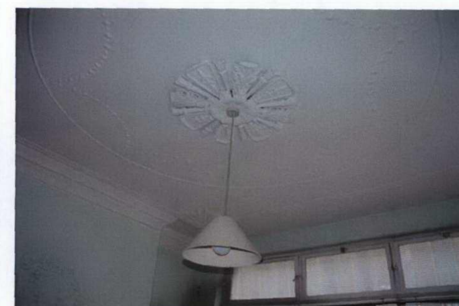
6. Front room ceiling
