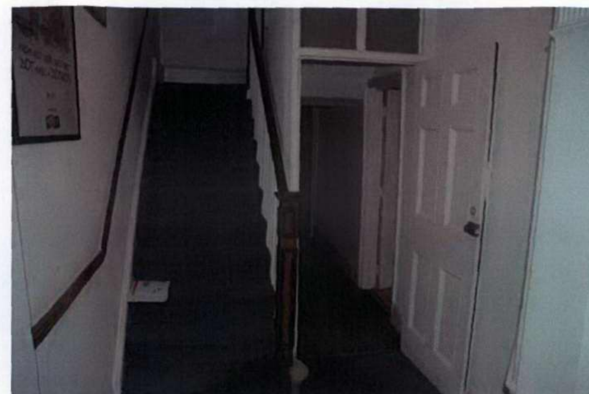
2. Stair to first floor
