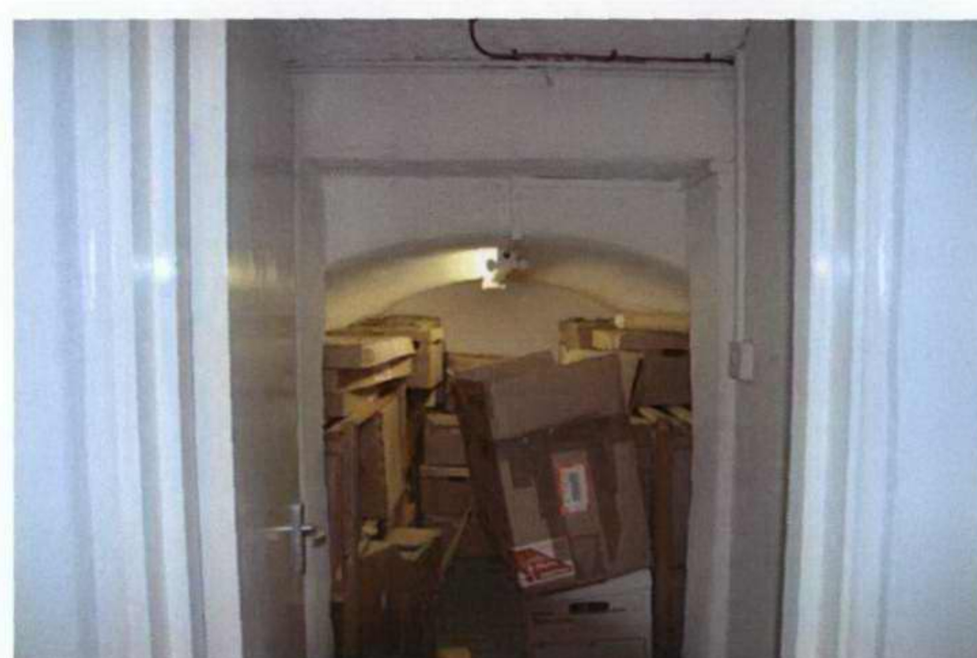
4. Vaults to rear
