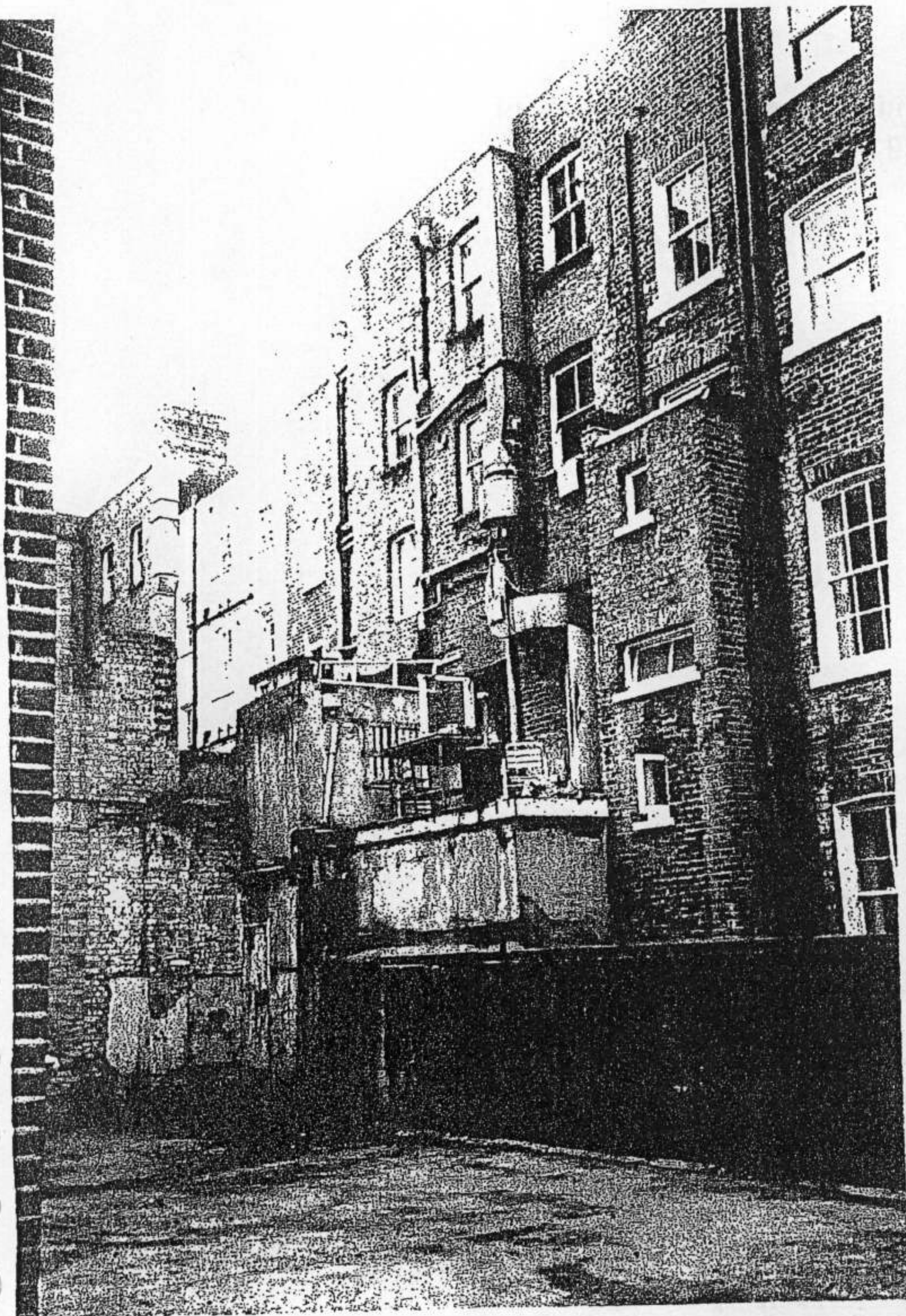
Plate 2 View of the rear of Nos. 22 and 24 Charlotte Street from the rear yard of Nos.7-15 Whitfield Street.
