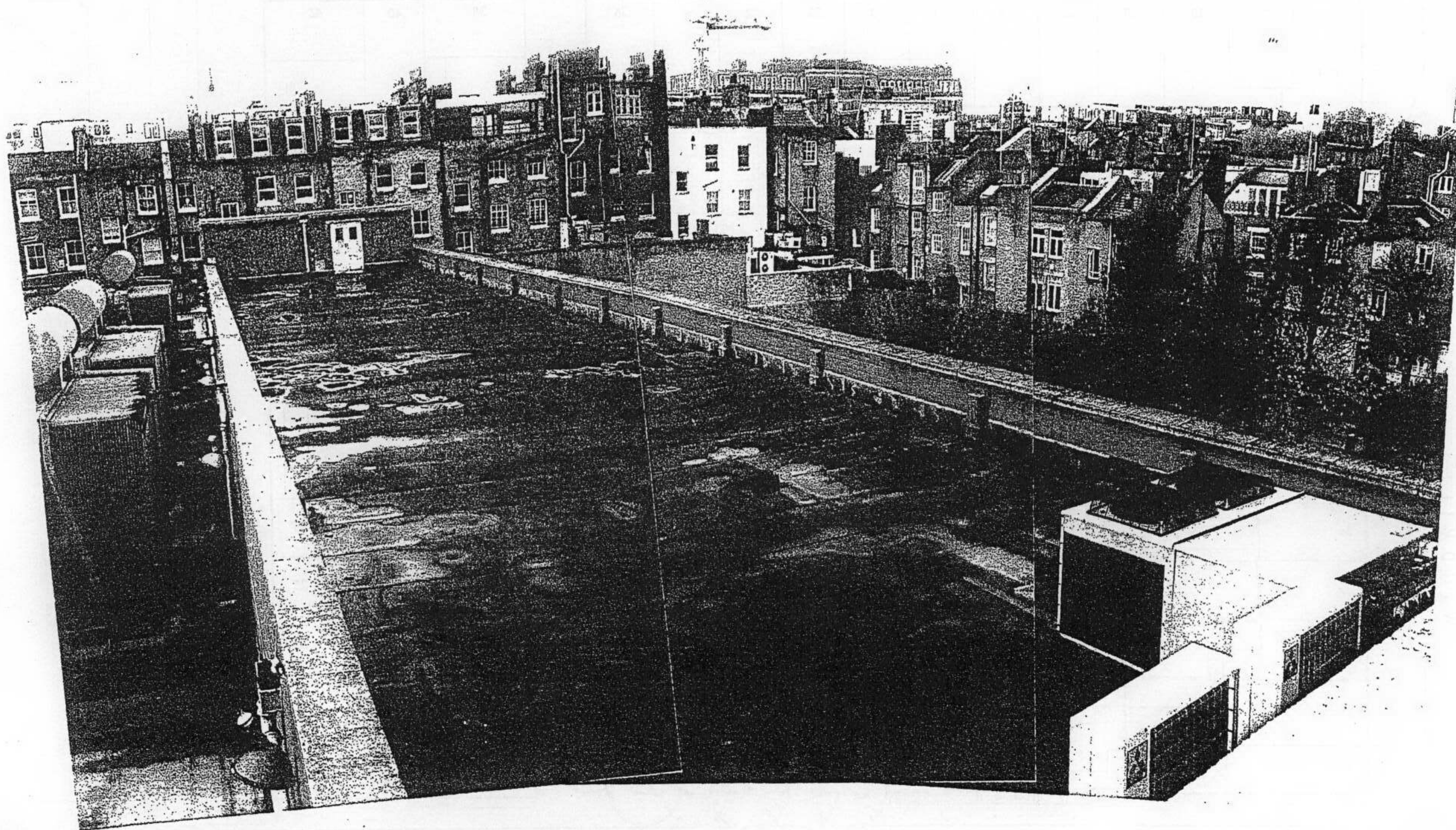
Plate 5 View of the buildings on Charlotte Street and Colville Place from the roof of the existing Whitfield Street building
