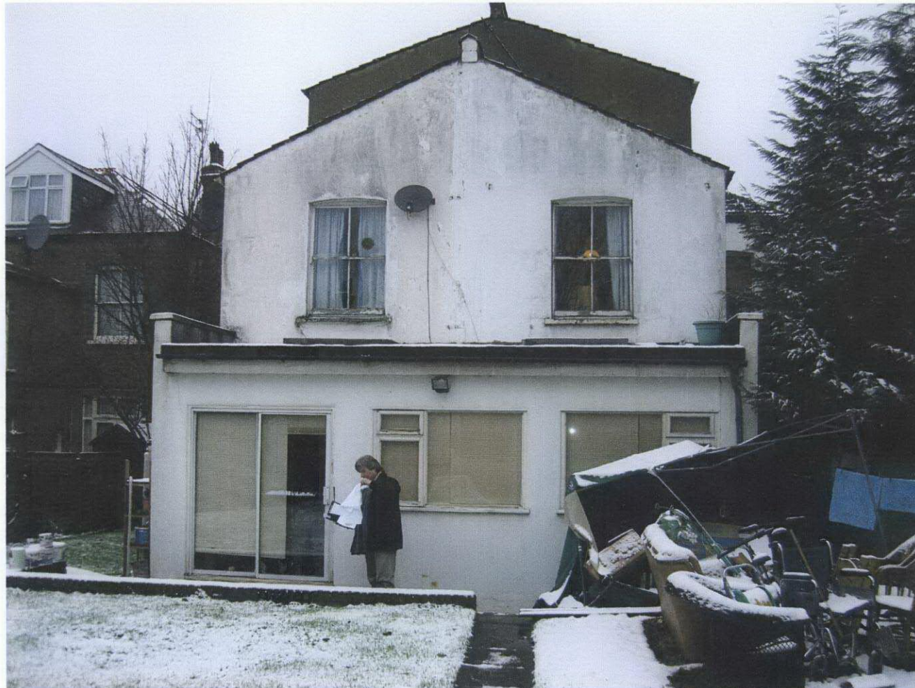
Rear Elevation of 13-15 Skardu Road
