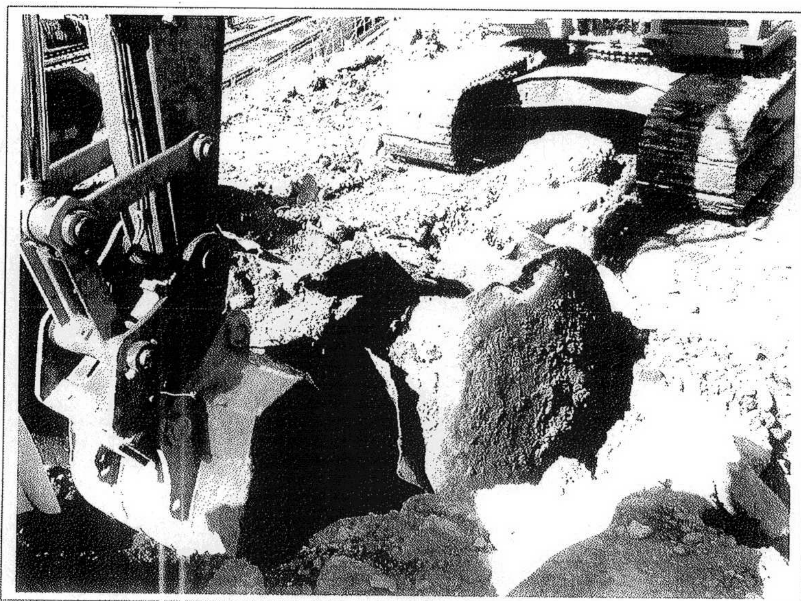
Photo 4: Removal of tank 3.
