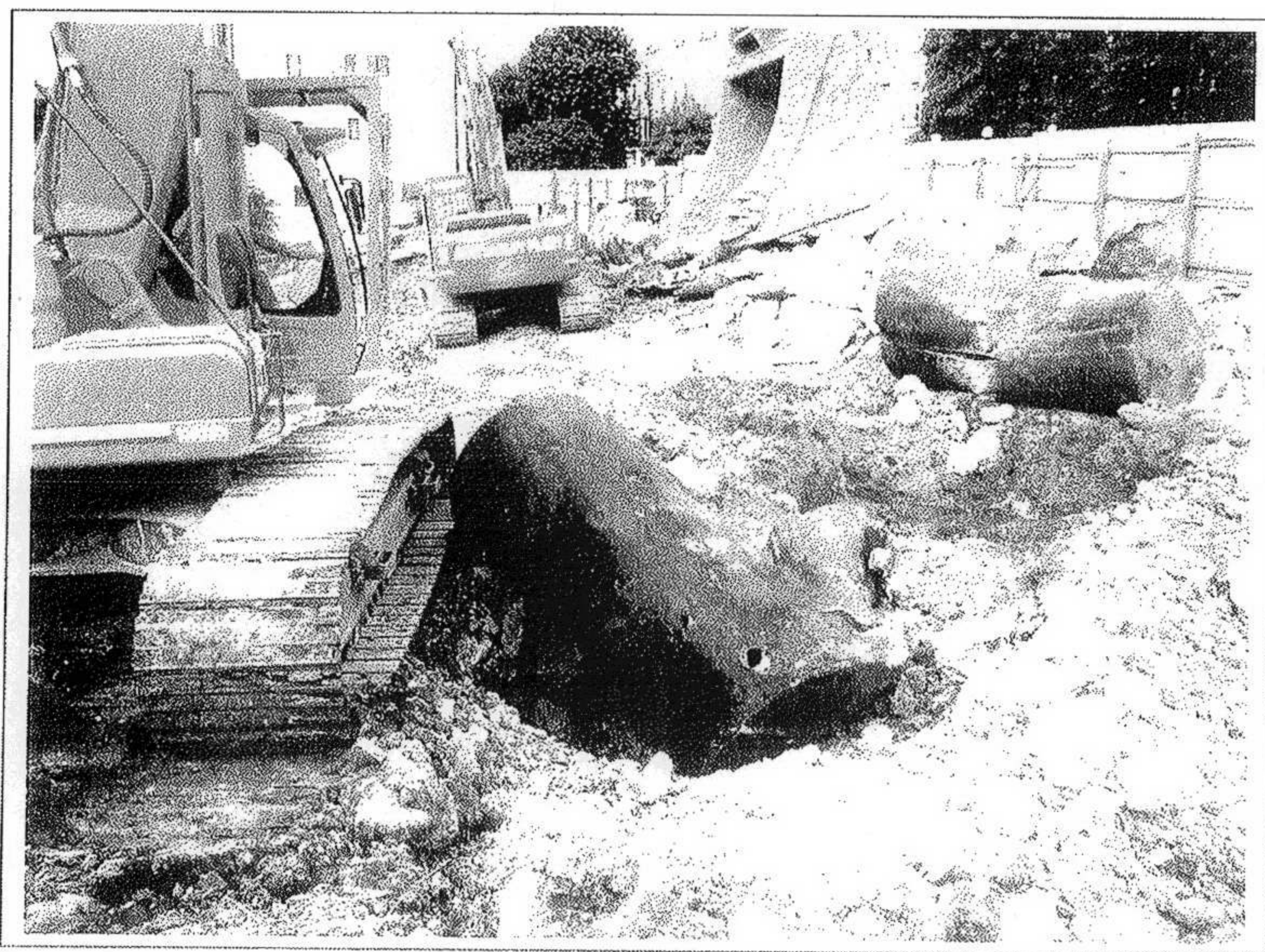
Photo 6: Removal of tank 8.
