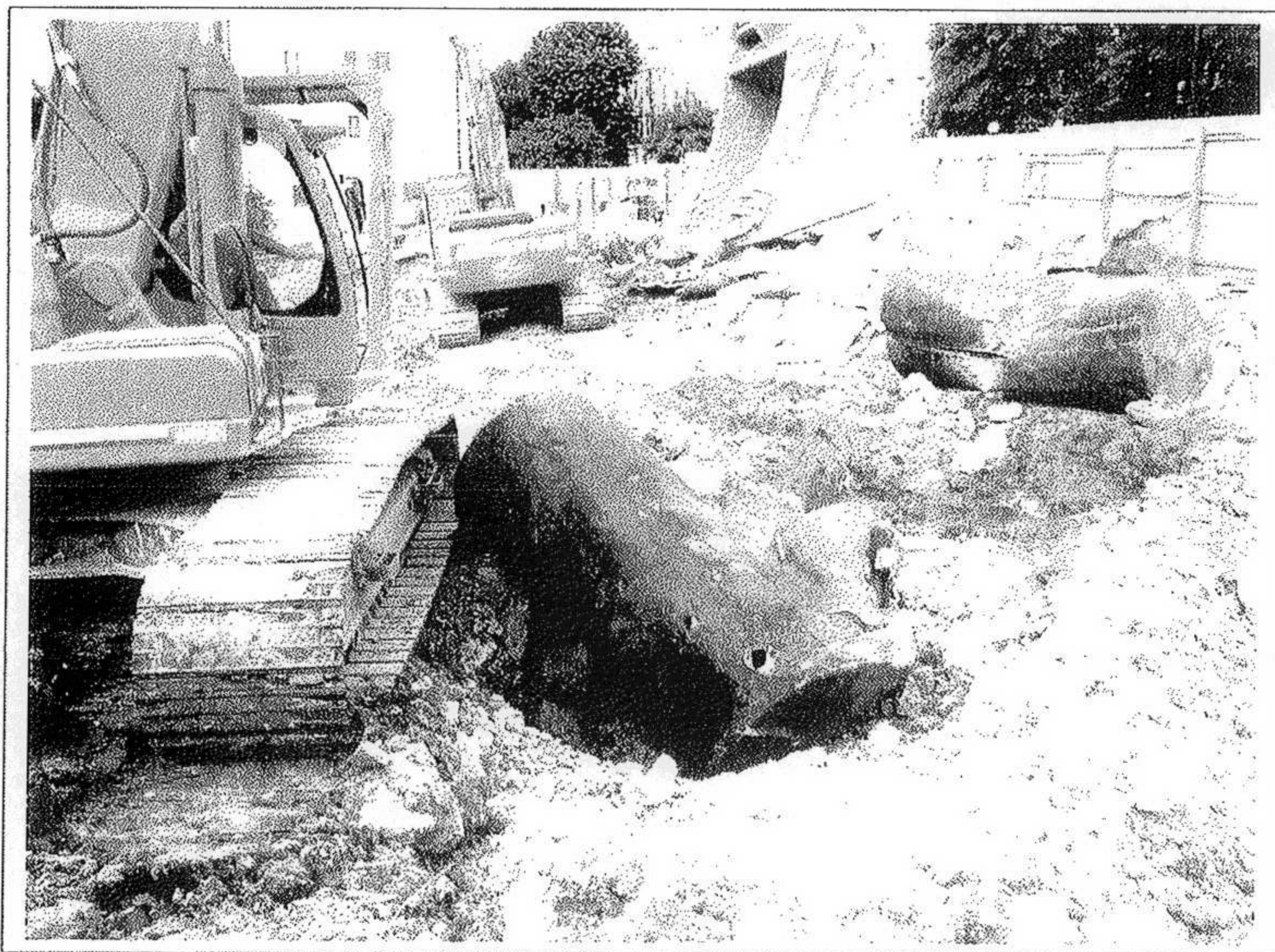
Photo 6: Removal of tank 8.
