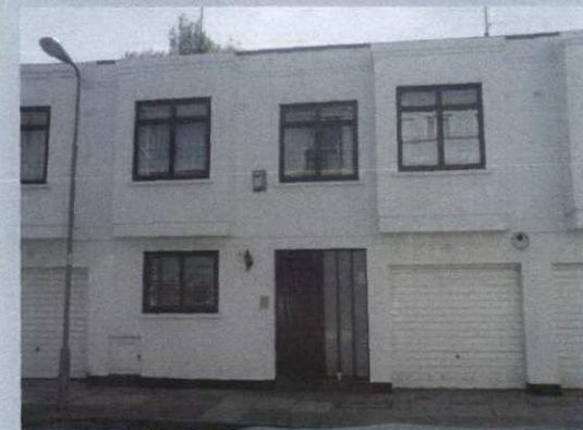
The existing front elevation of 53 Belsize Lane
