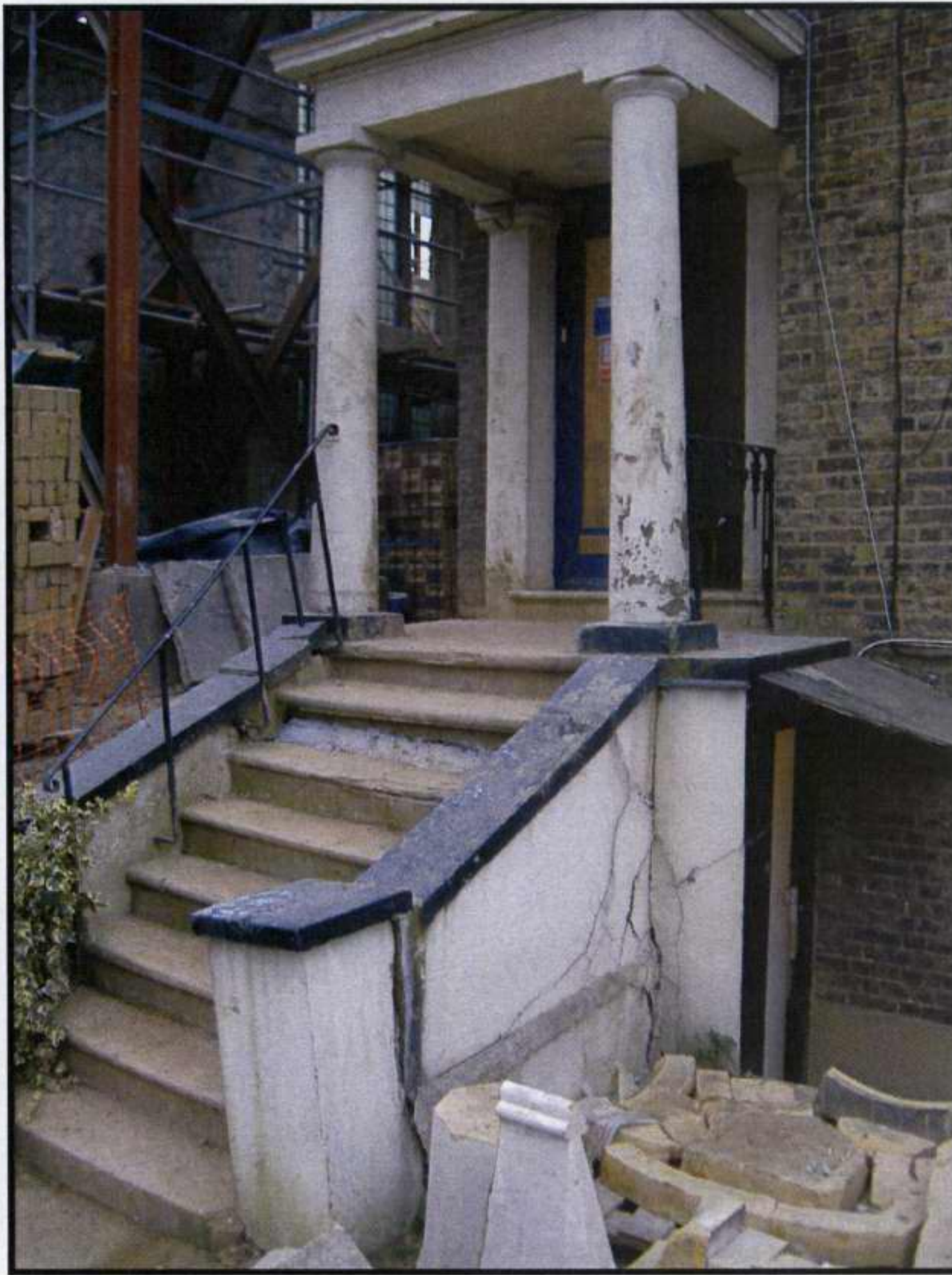
4. Collapsing pier and unstable steps and portico to front (west) elevation.
