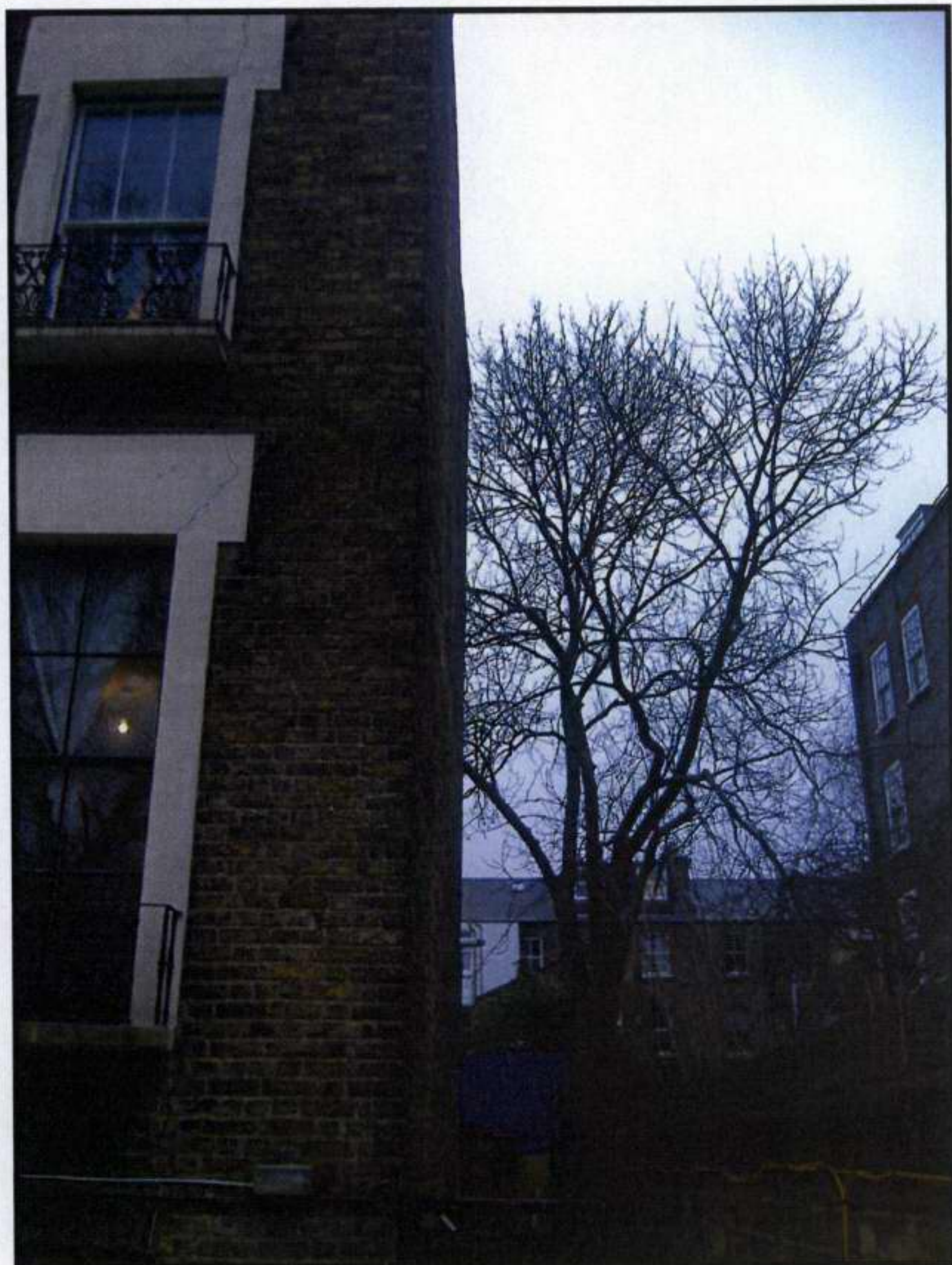
1. Severe bowing/belly to south flank elevation.
