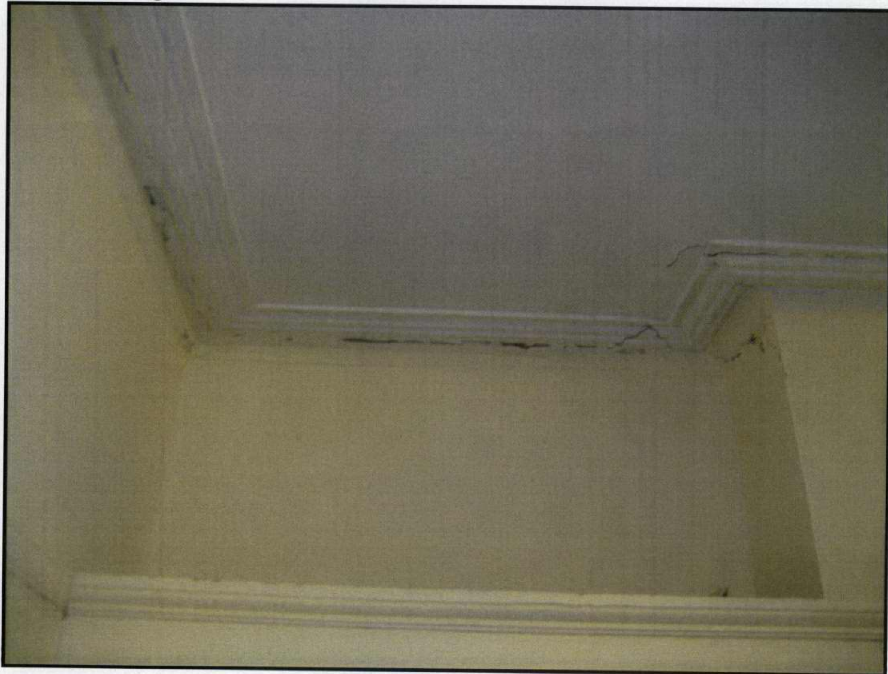
11. Severe fracture to first floor cornice to south elevation.
