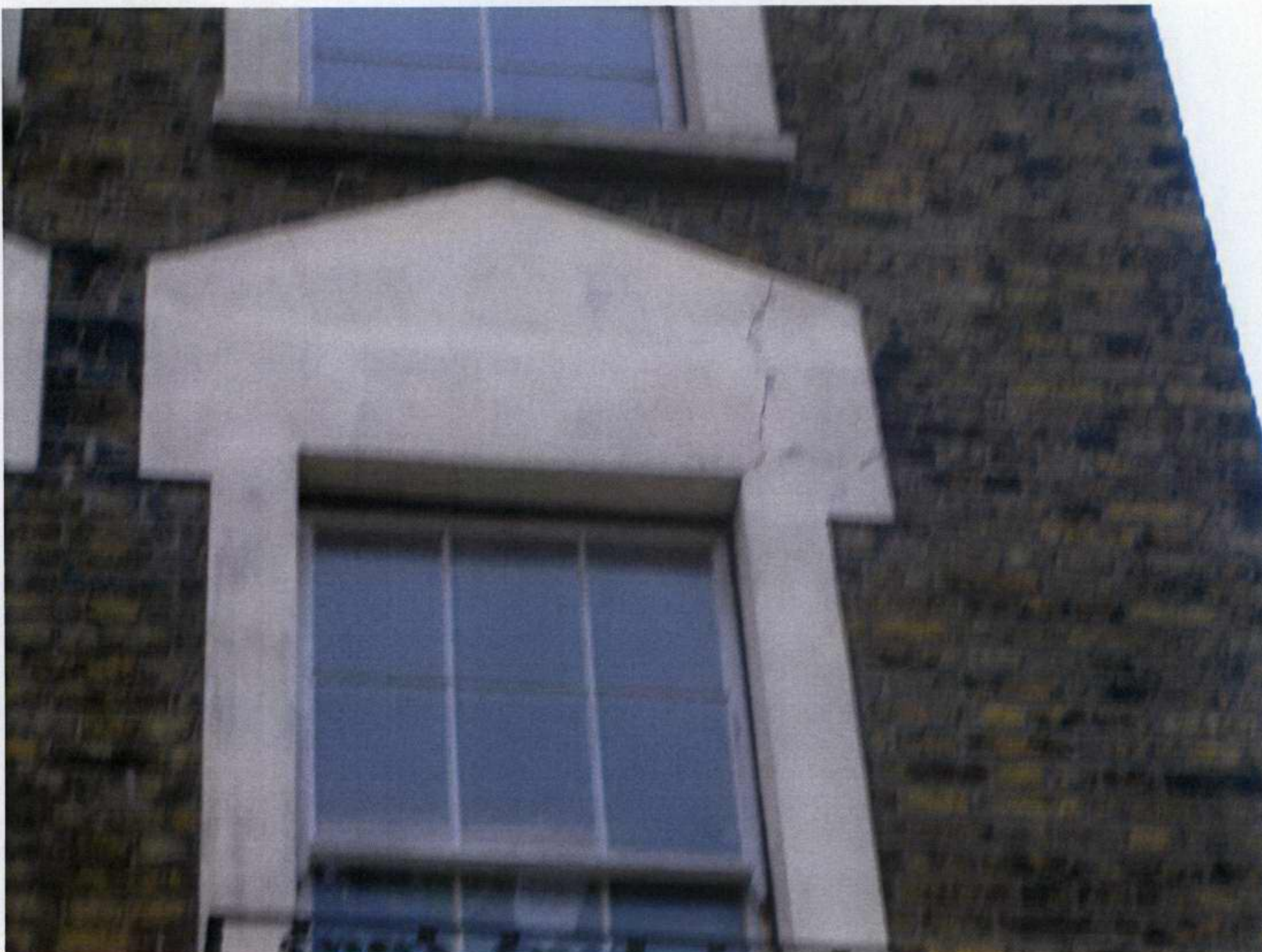
7. Severe vertical fracture to first floor lintel where south wall is separating from building.
