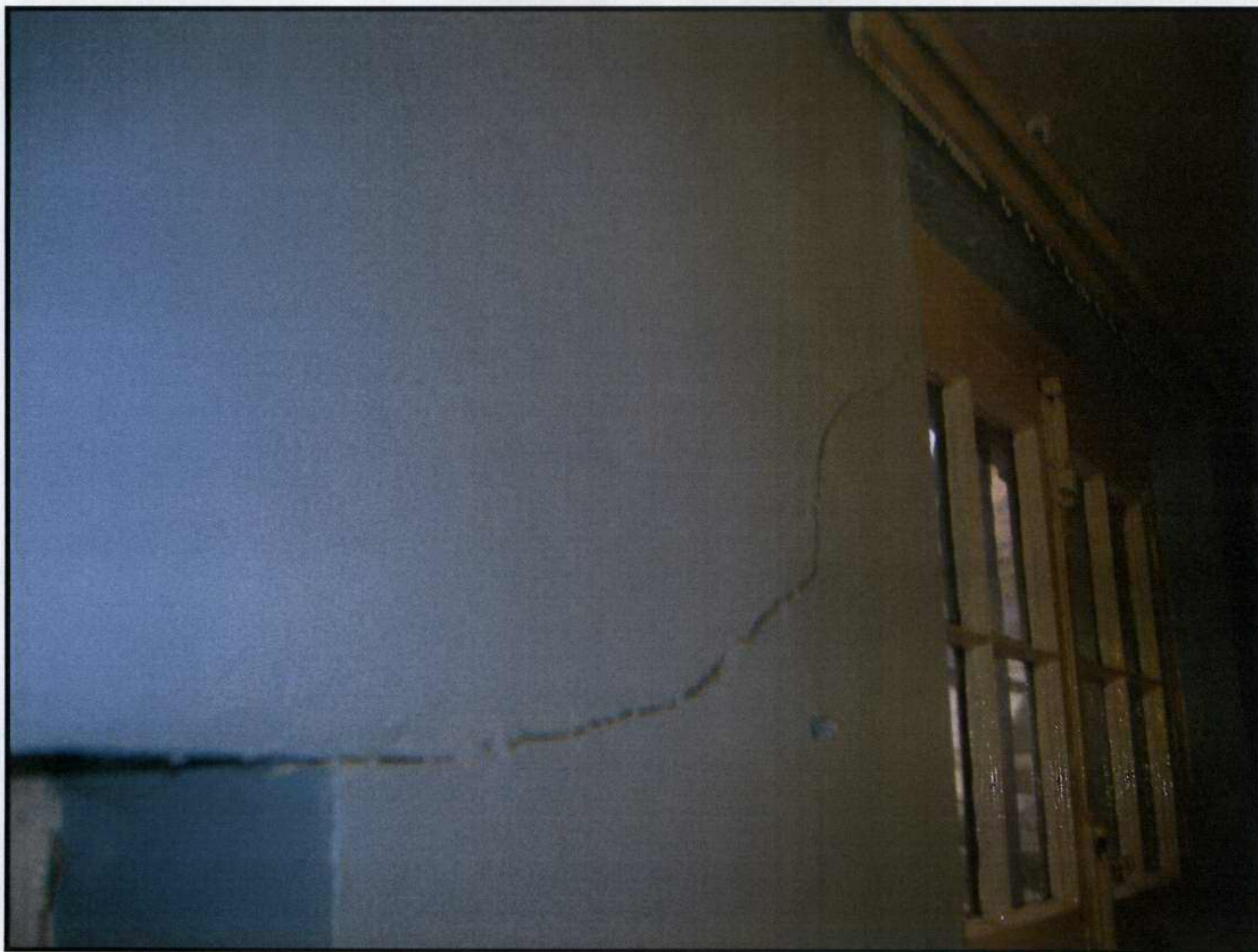
13. Severe horizontal fracture to rear outrigger at basement level caused by drain blockage from tree roots and rotation of outriggers.
