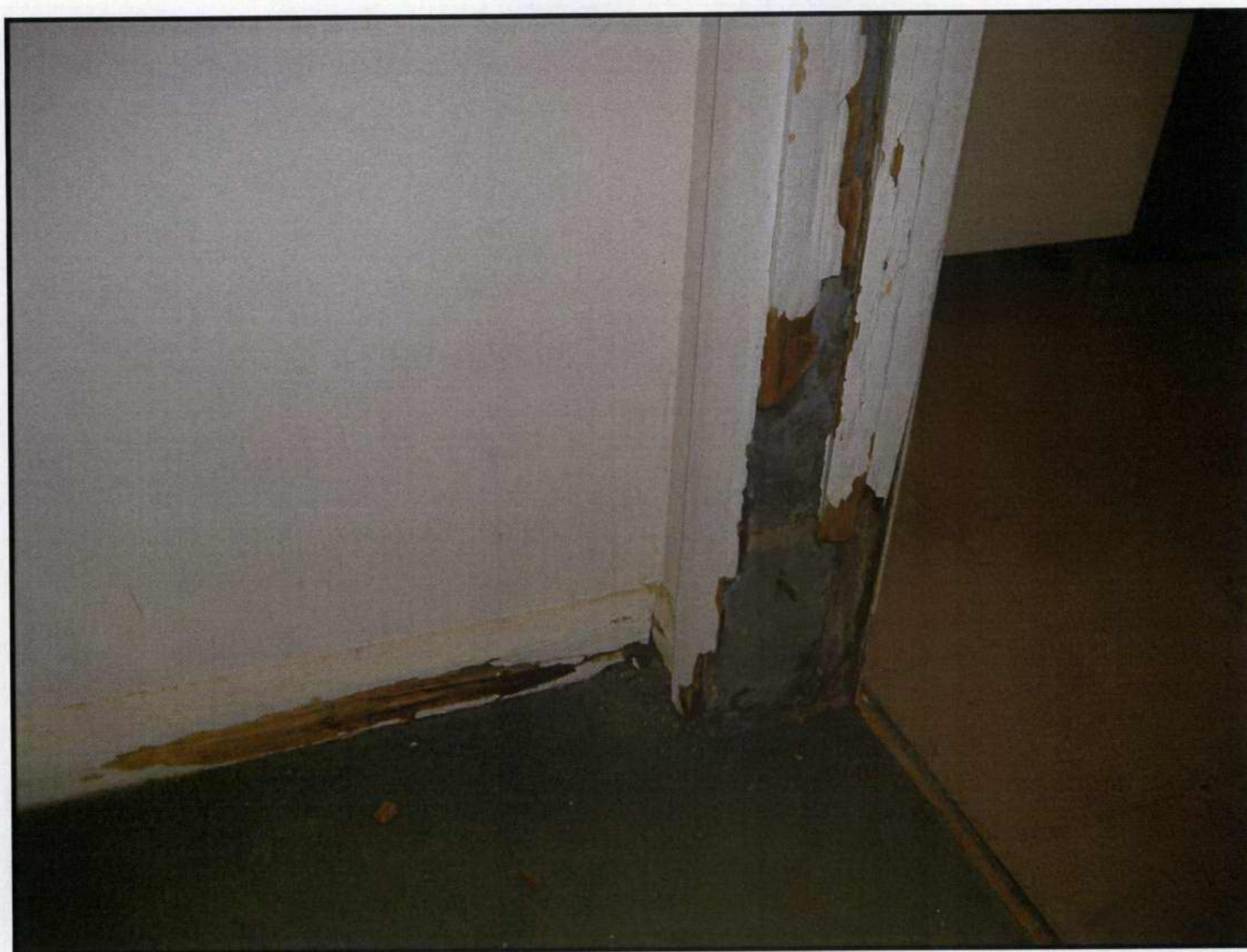
16. Extensive dry rot to timber skirtings and door lining.
