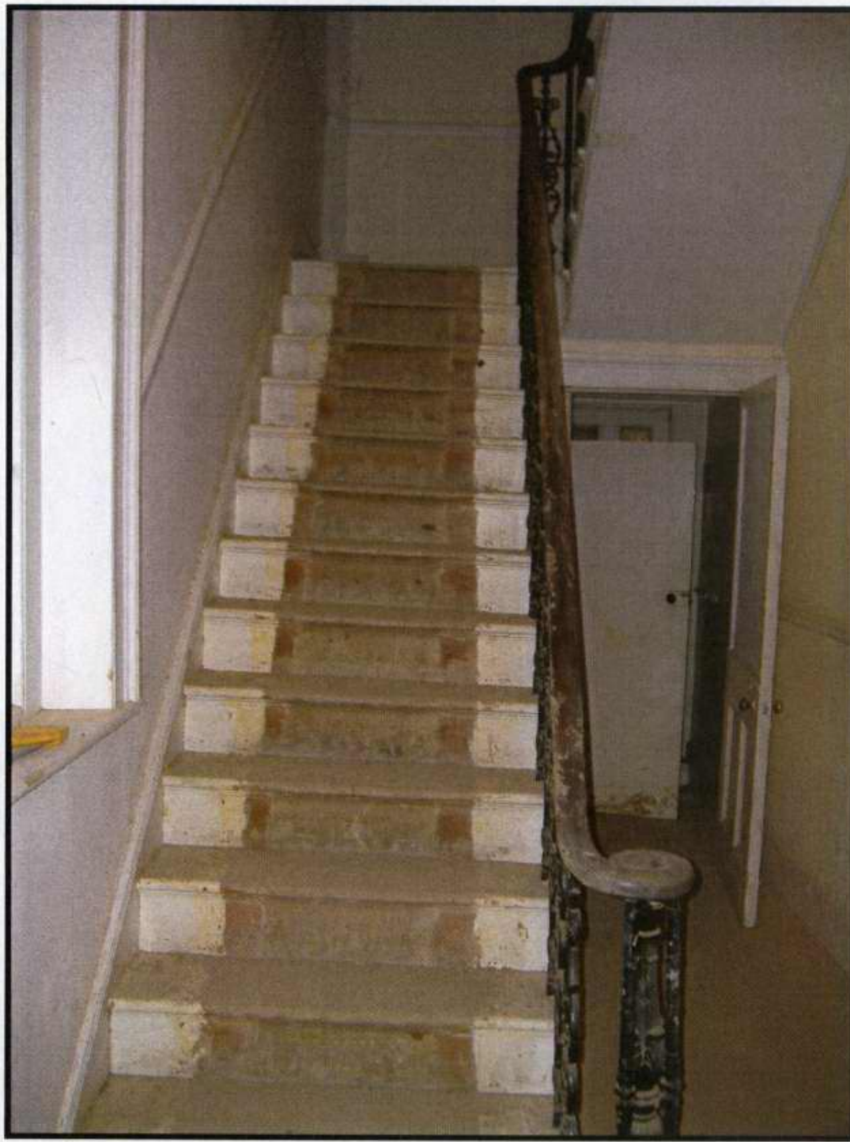
14. Severe deflection to staircase at first floor.
