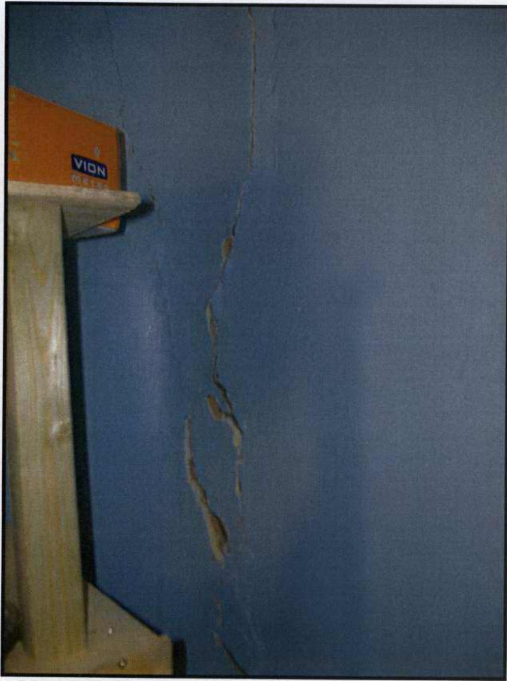
10. 20mm fracture internally at basement level where south wall is separating from the building.
