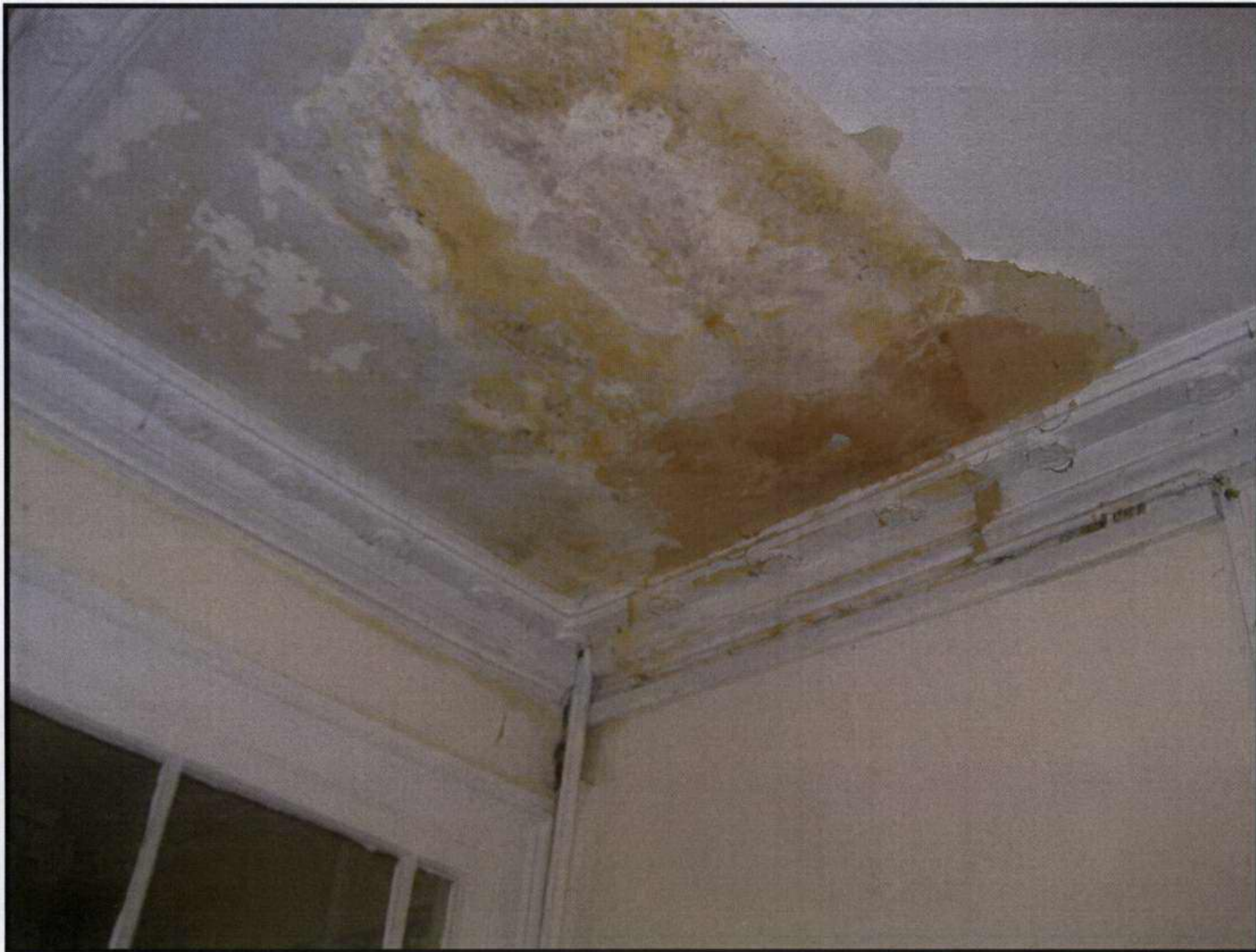
12. Water ingress and dry rot possibility to first floor ceiling.
