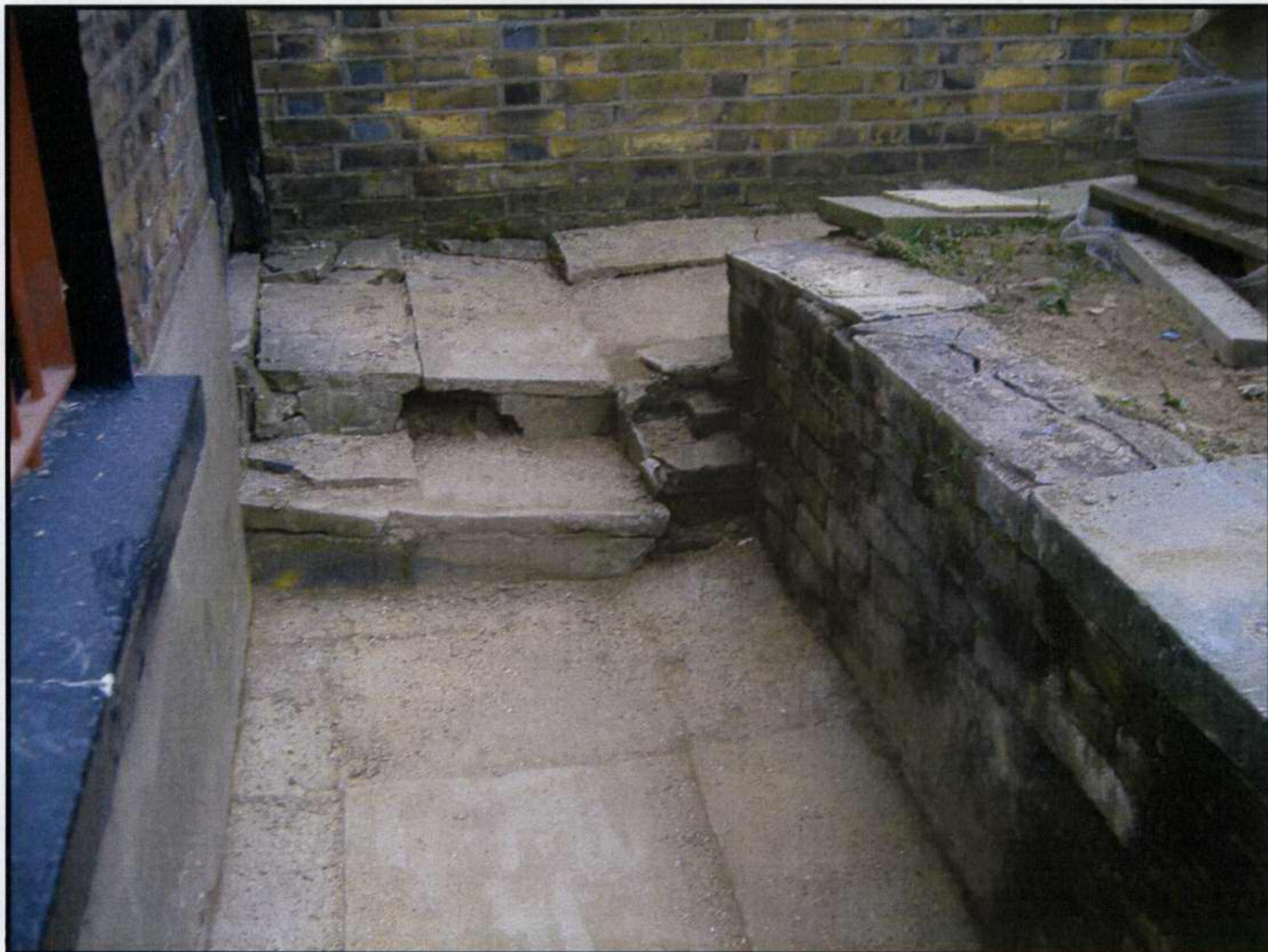
5. Settlement to steps and unstable retaining wall.
