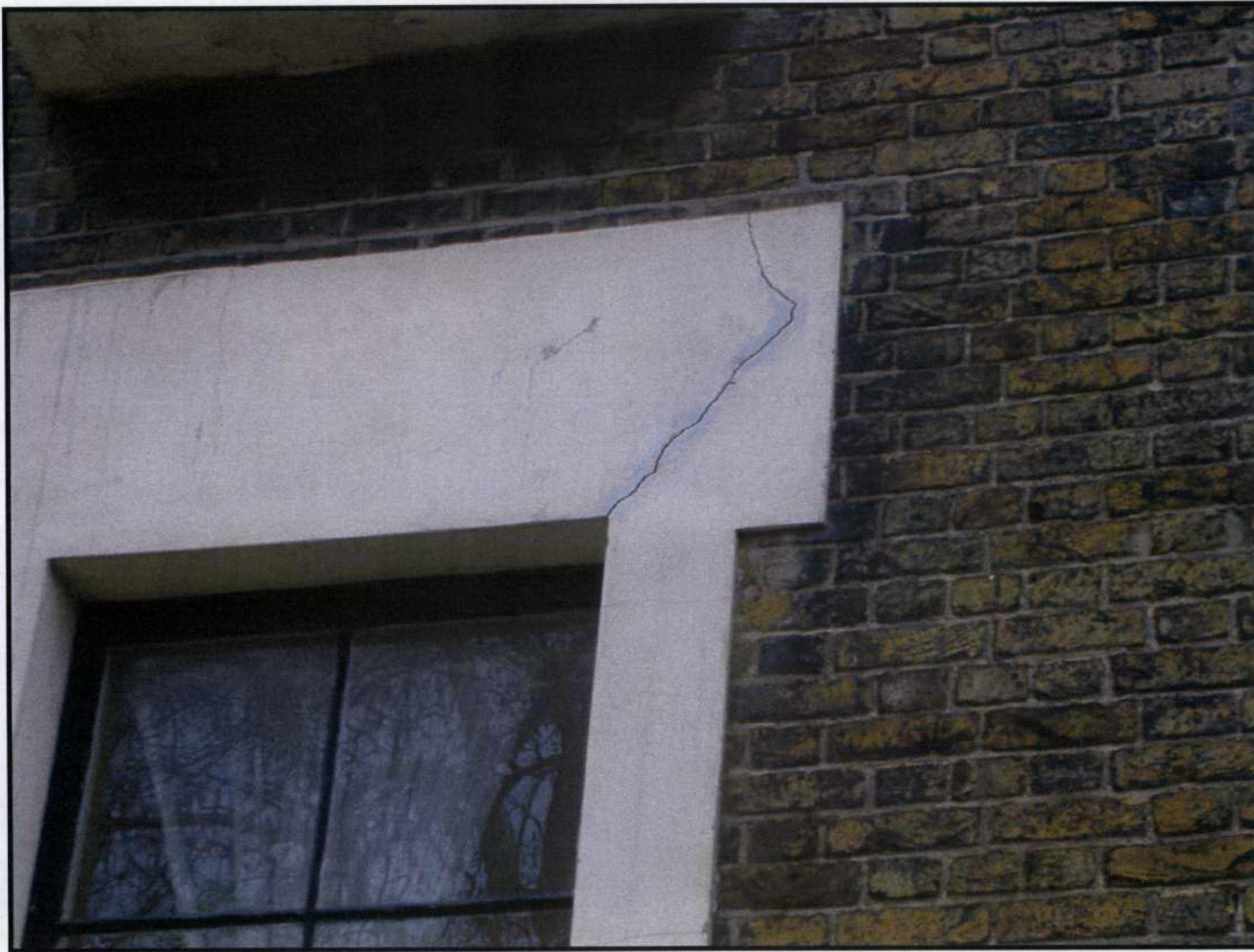
6. Severe diagonal fracture to lintel to Ground floor window.
