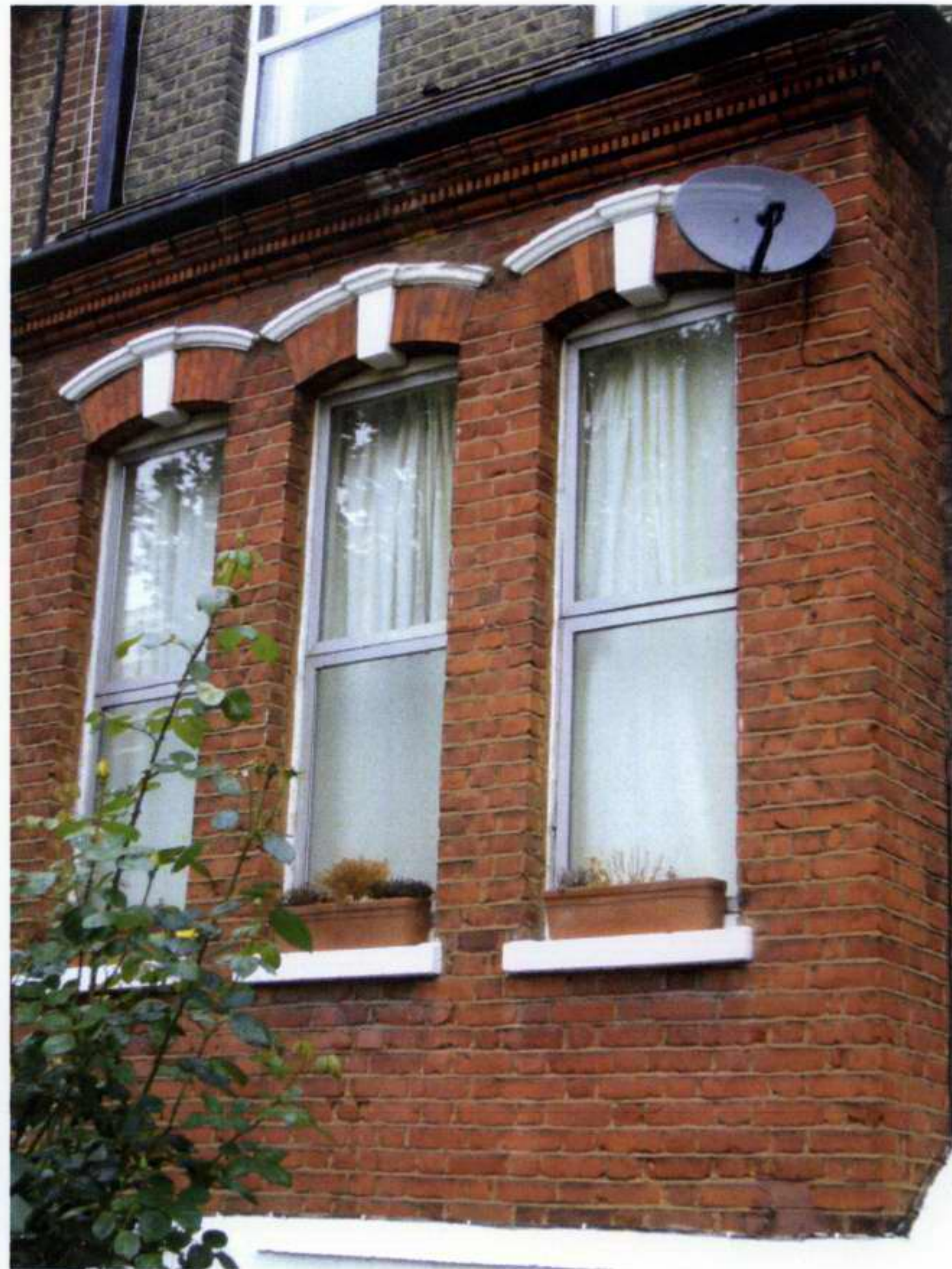
Front Windows - Upper Ground Floor
