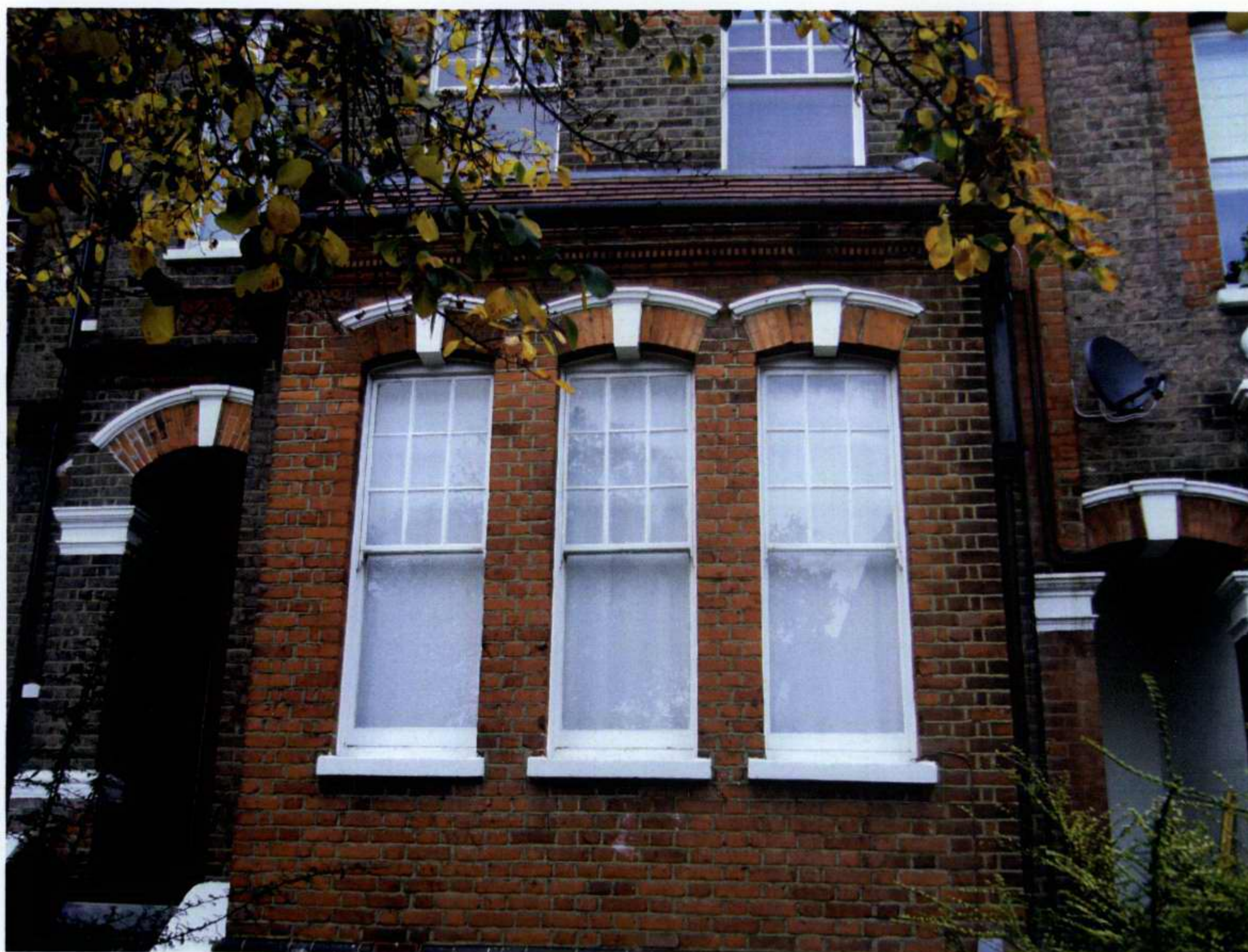
FRONT OF NUMBER 14 (situated on the right hand side of 16 Dennington Park Road)
