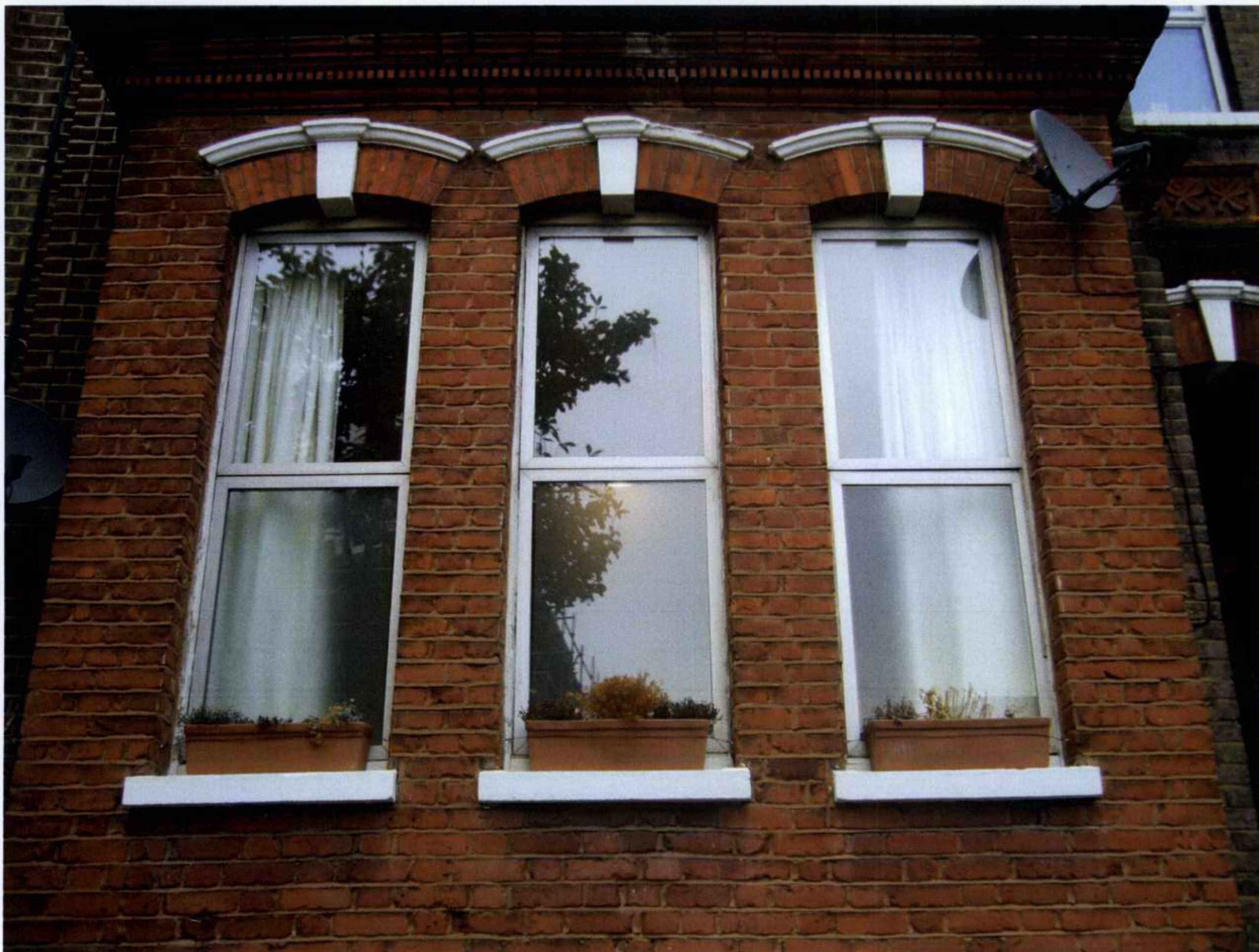
Front Windows – Upper Ground Floor
