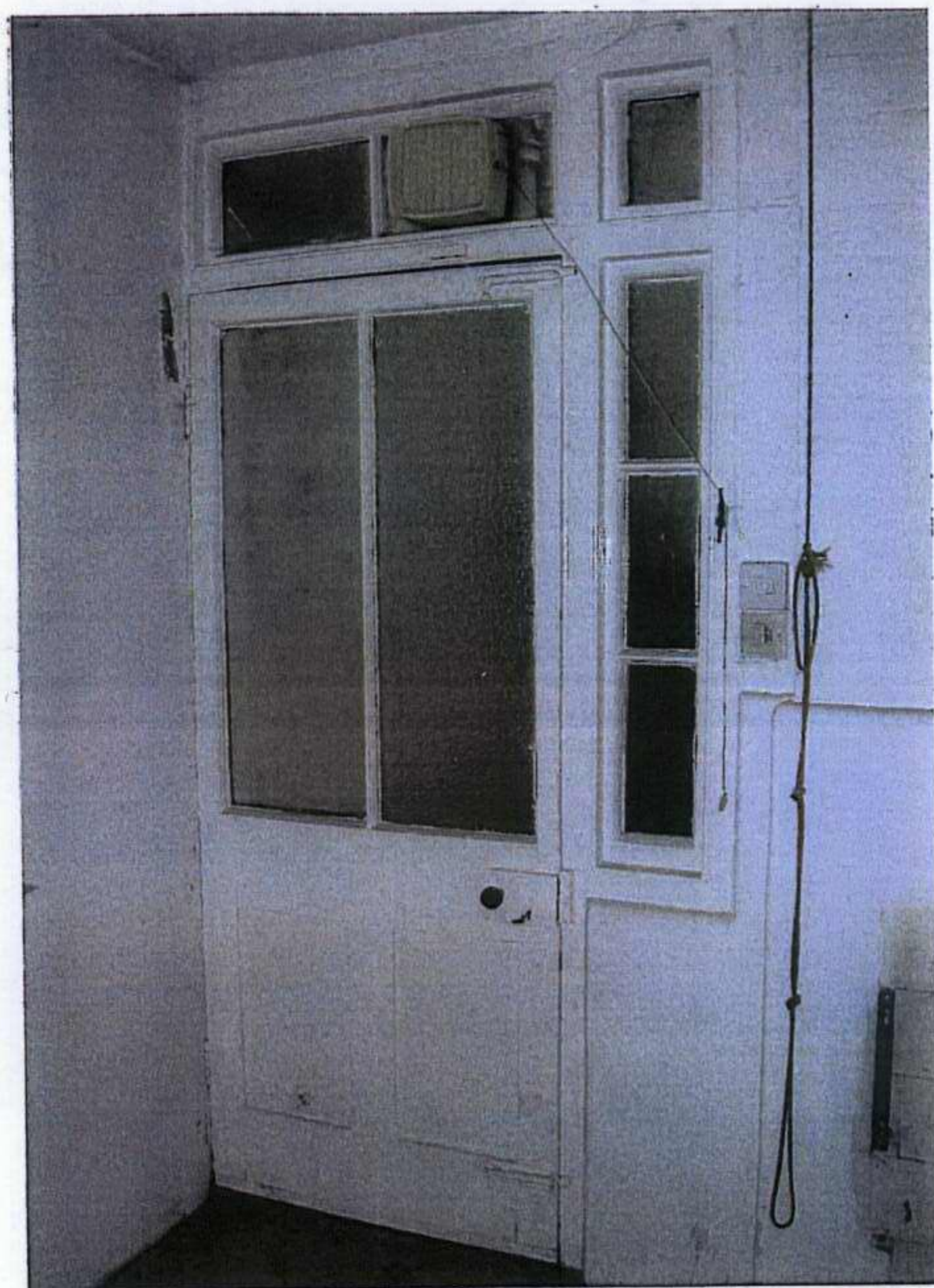
VIEW A EXISTING DOOR TO BE RETAINED.
