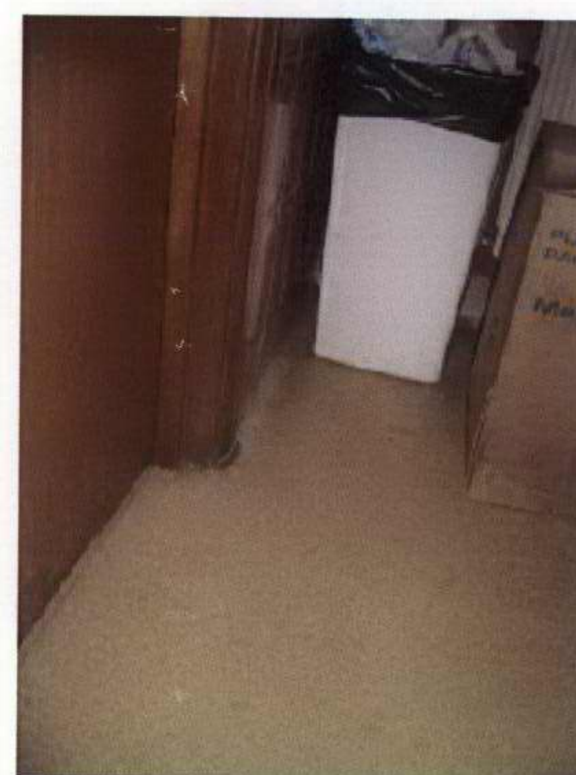
62. Second floor bathroom ES3
