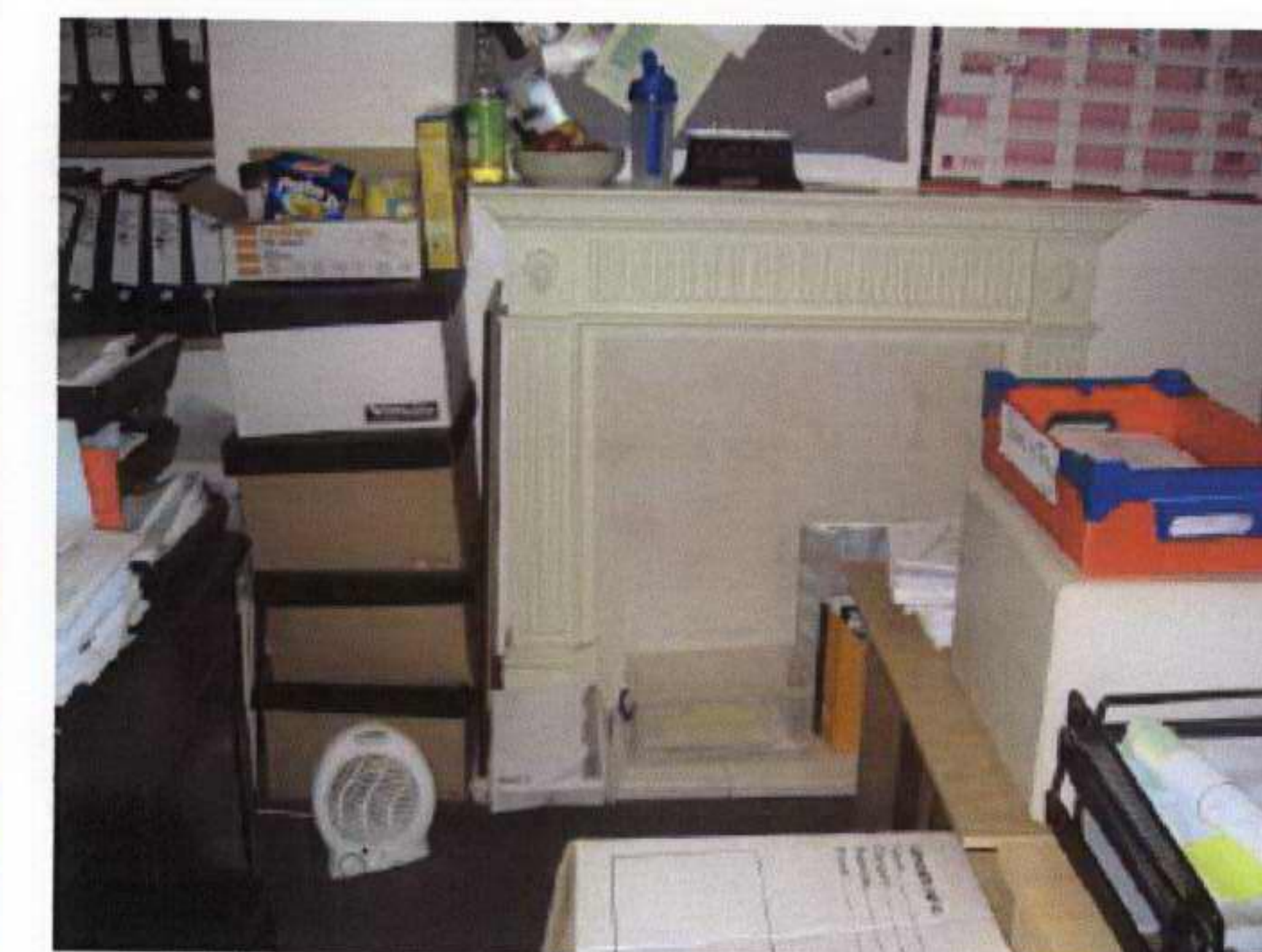
64. Second floor front office ES1
