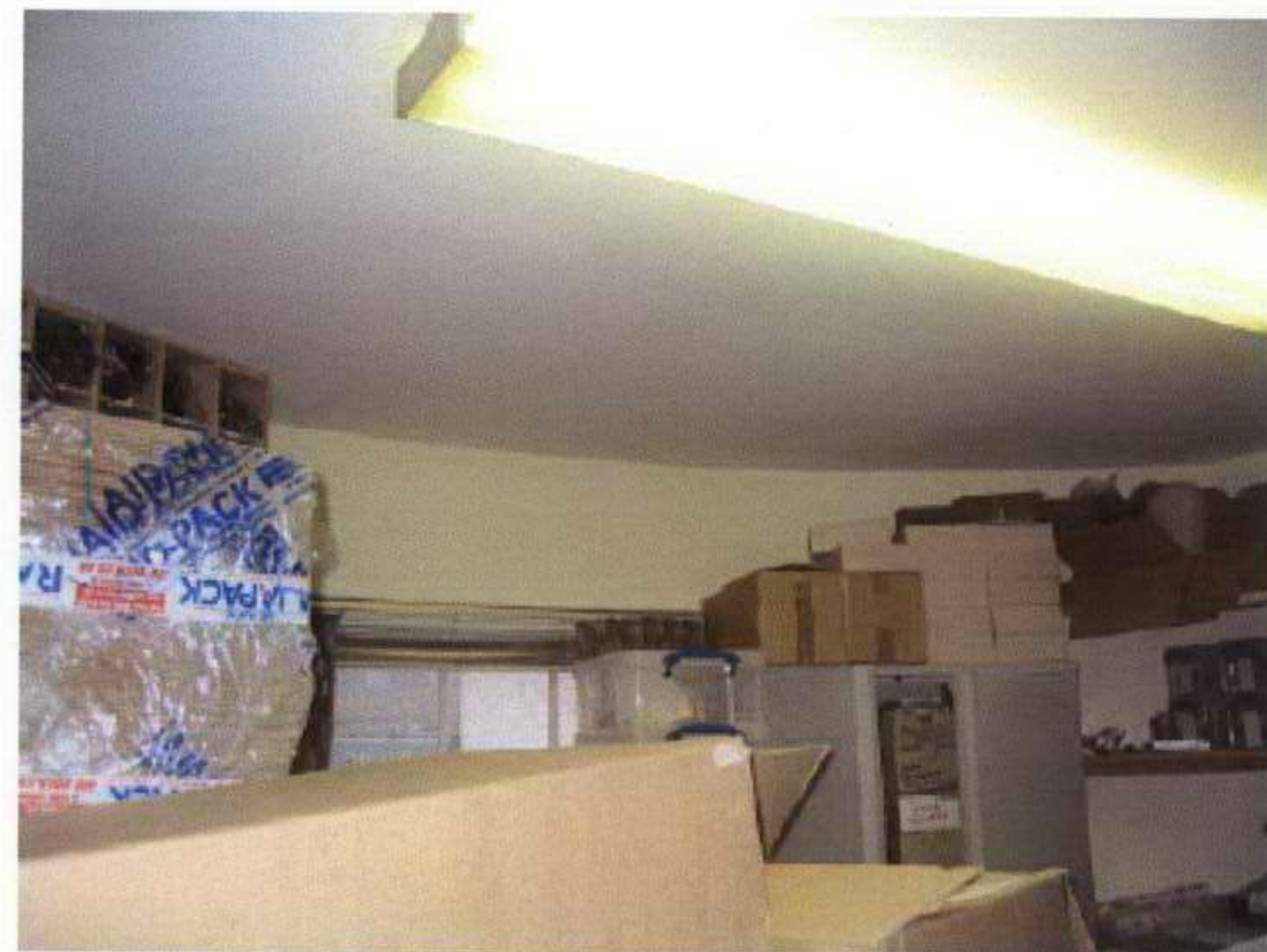
77. Third floor rear office ET3
