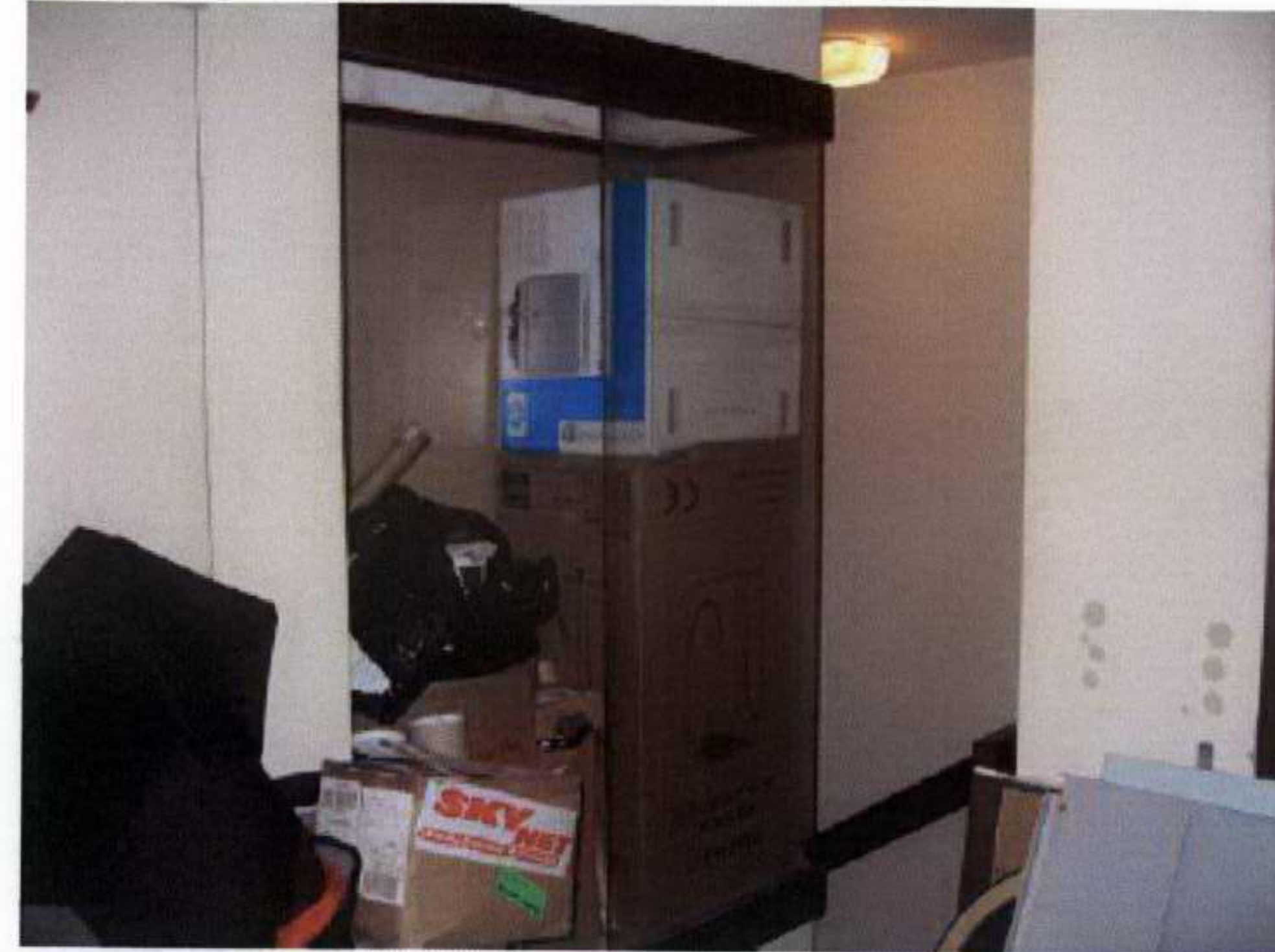
74. Third floor light well ET7
