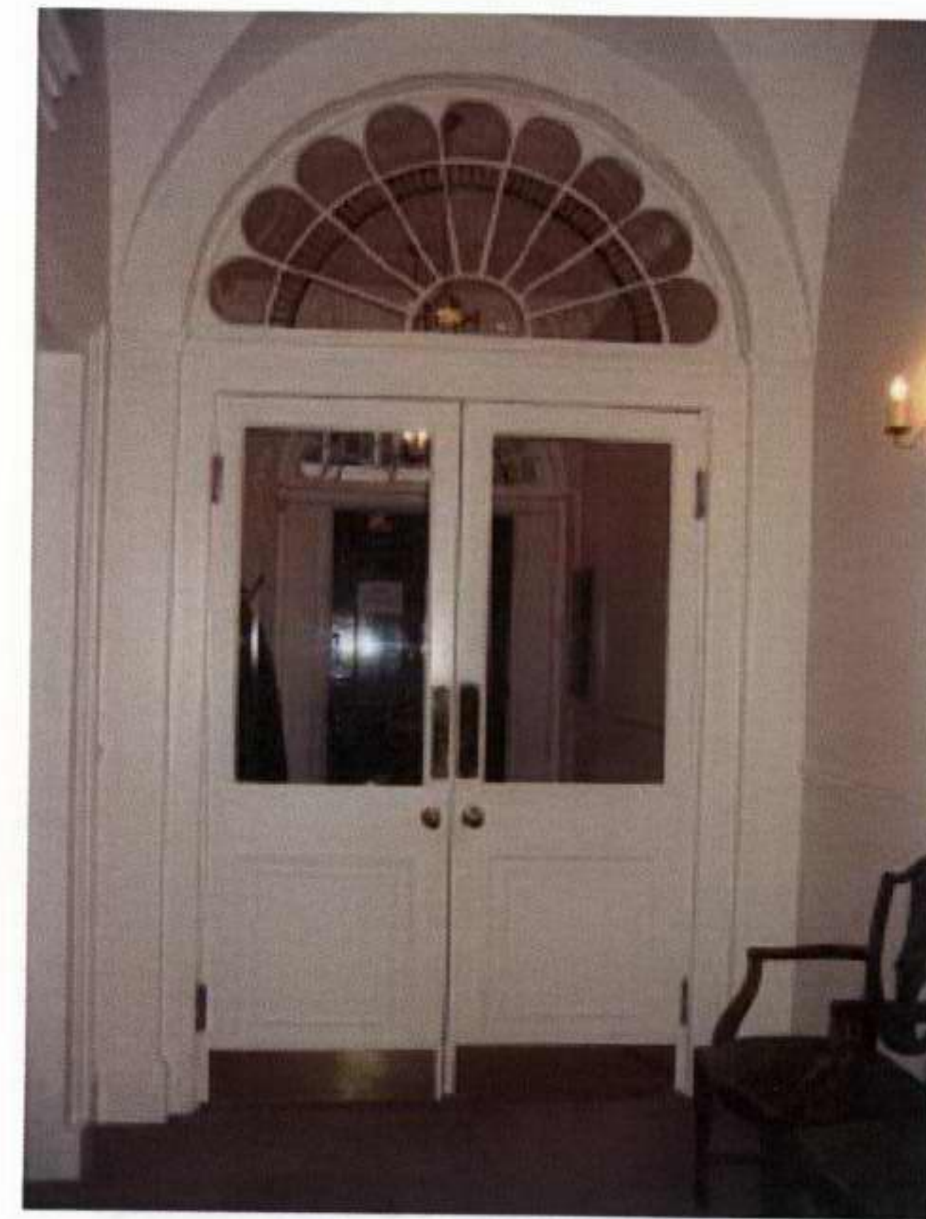
98. No 10 Fitzroy Square ground floor lobby G02
