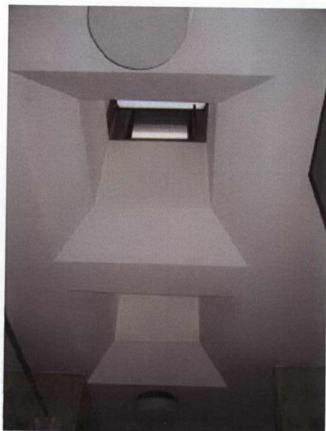
87. Third floor bathroom rooflights ET4
