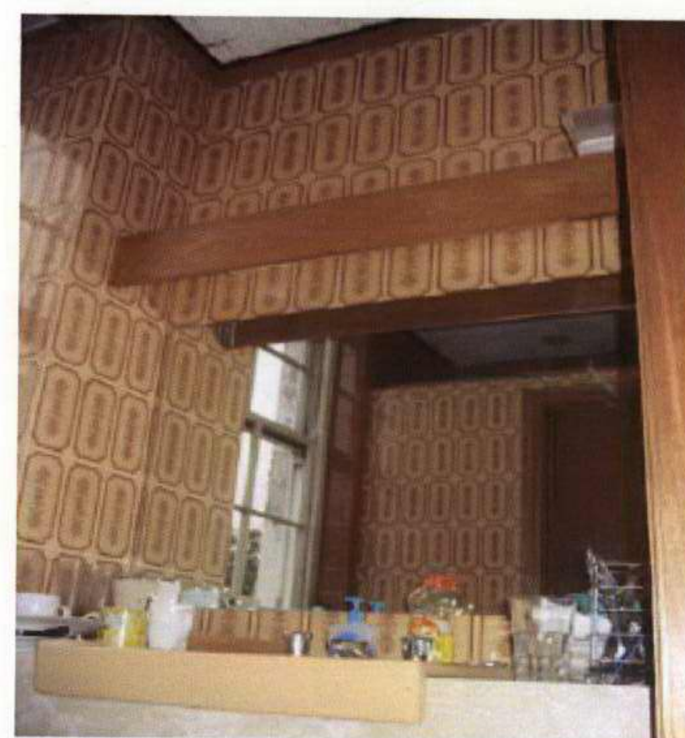
61. Second floor bathroom ES3
