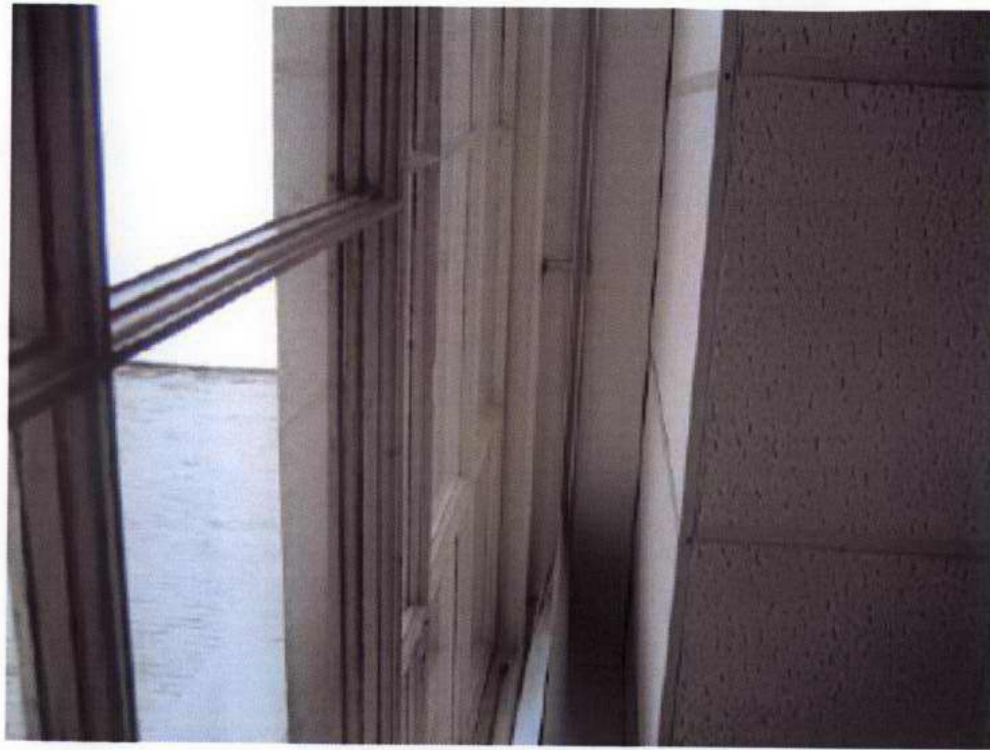
51. First floor rear office suspended ceiling EF3
