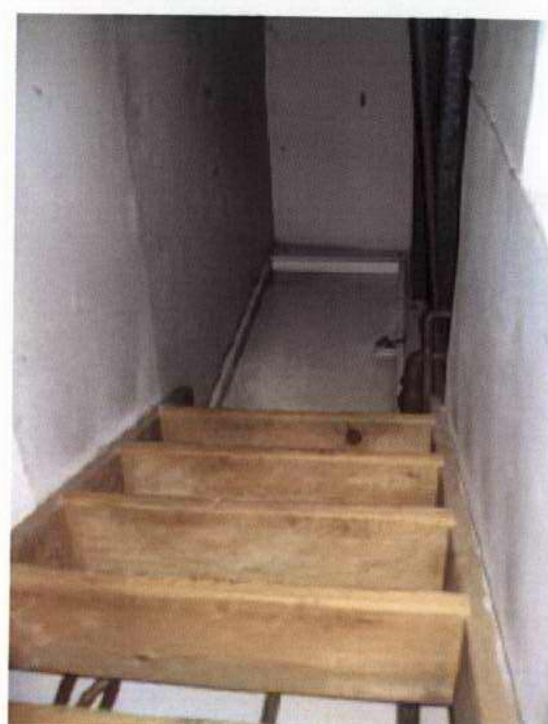
92. Third floor roof access ET5
