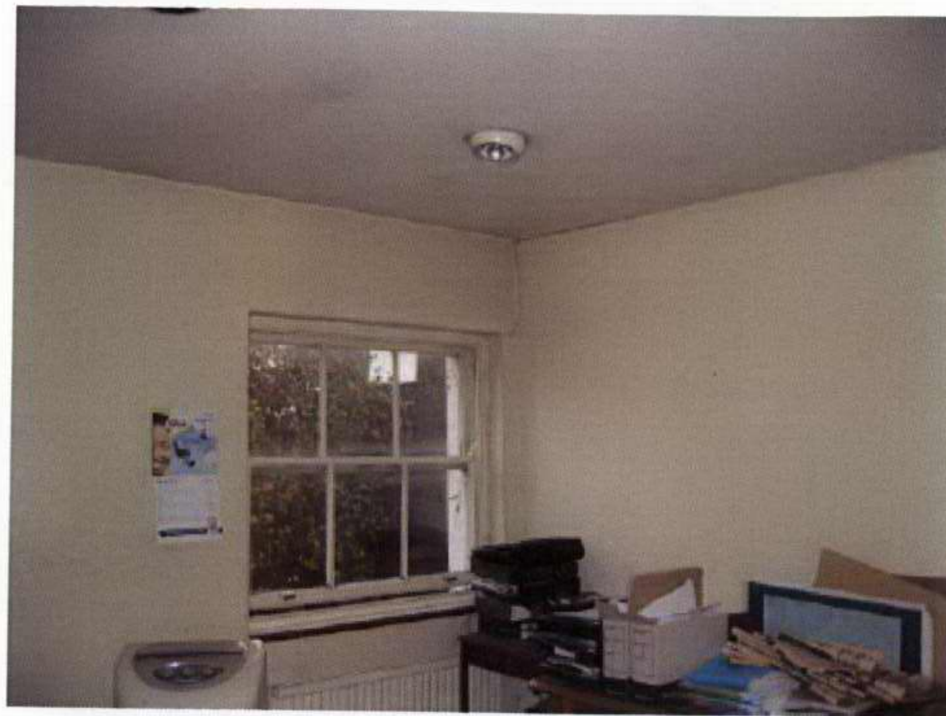
83. Third floor front office ET1
