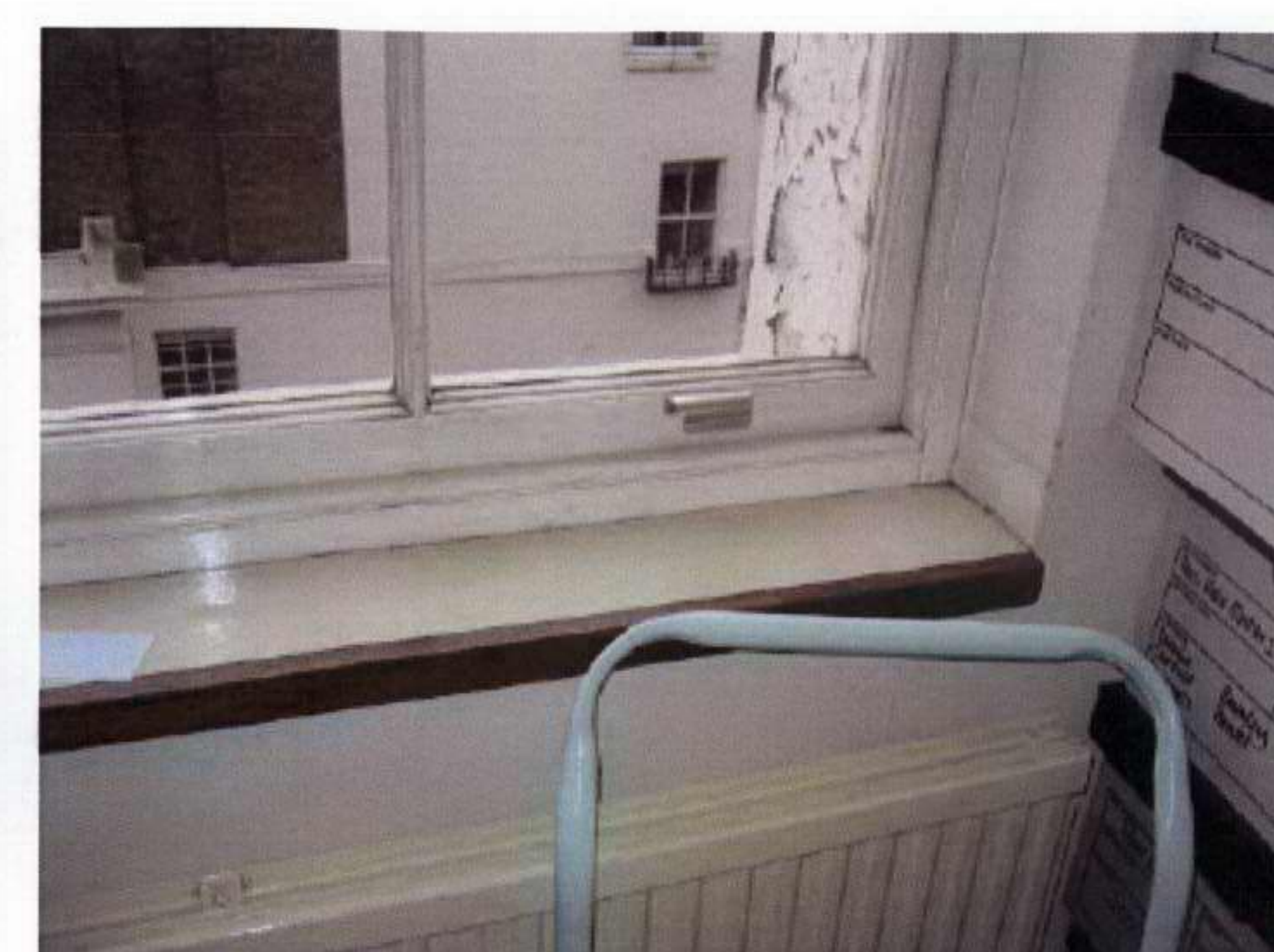
71. Second floor rear office window ES2
