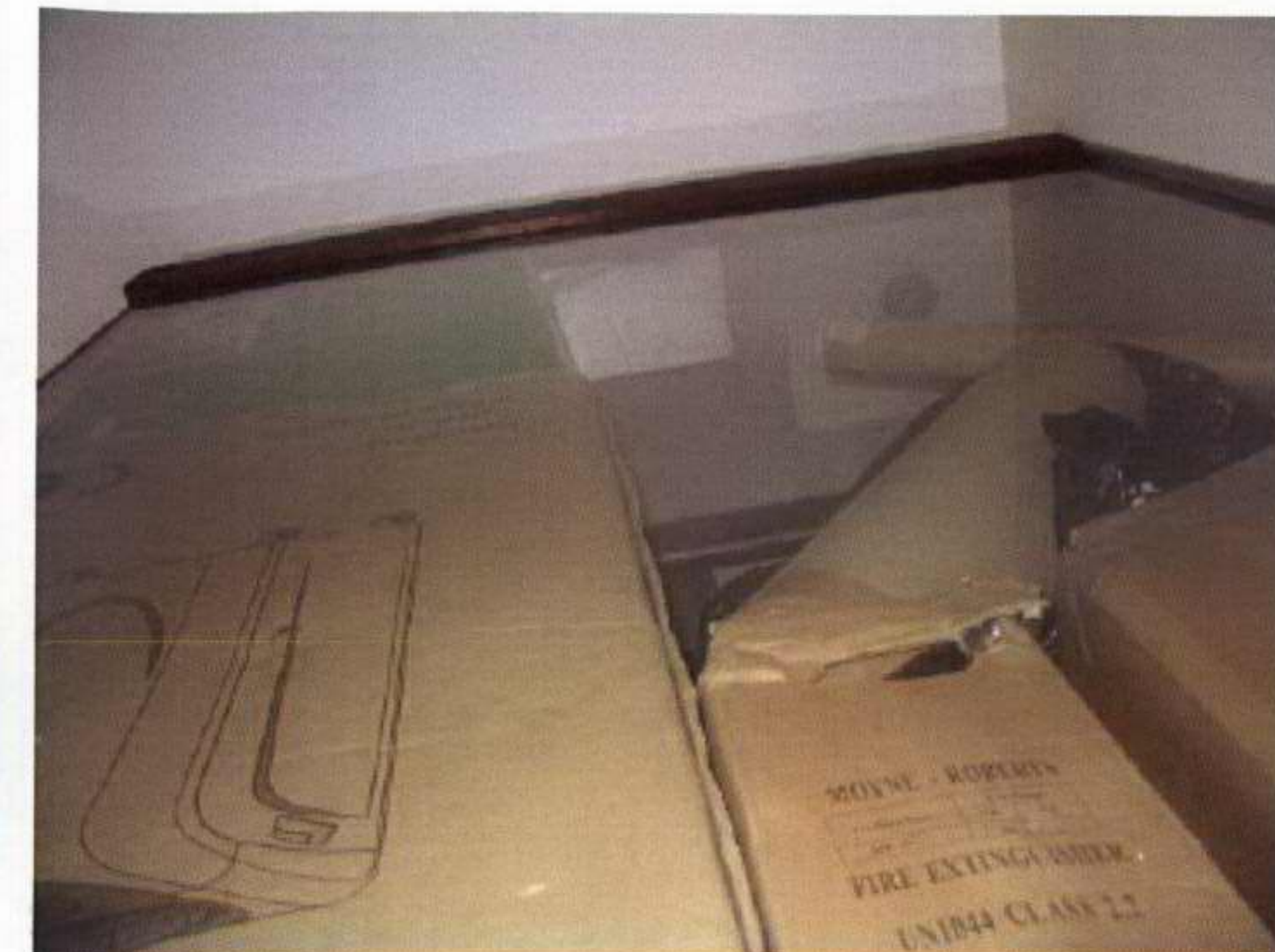
75. Third floor light well ET7
