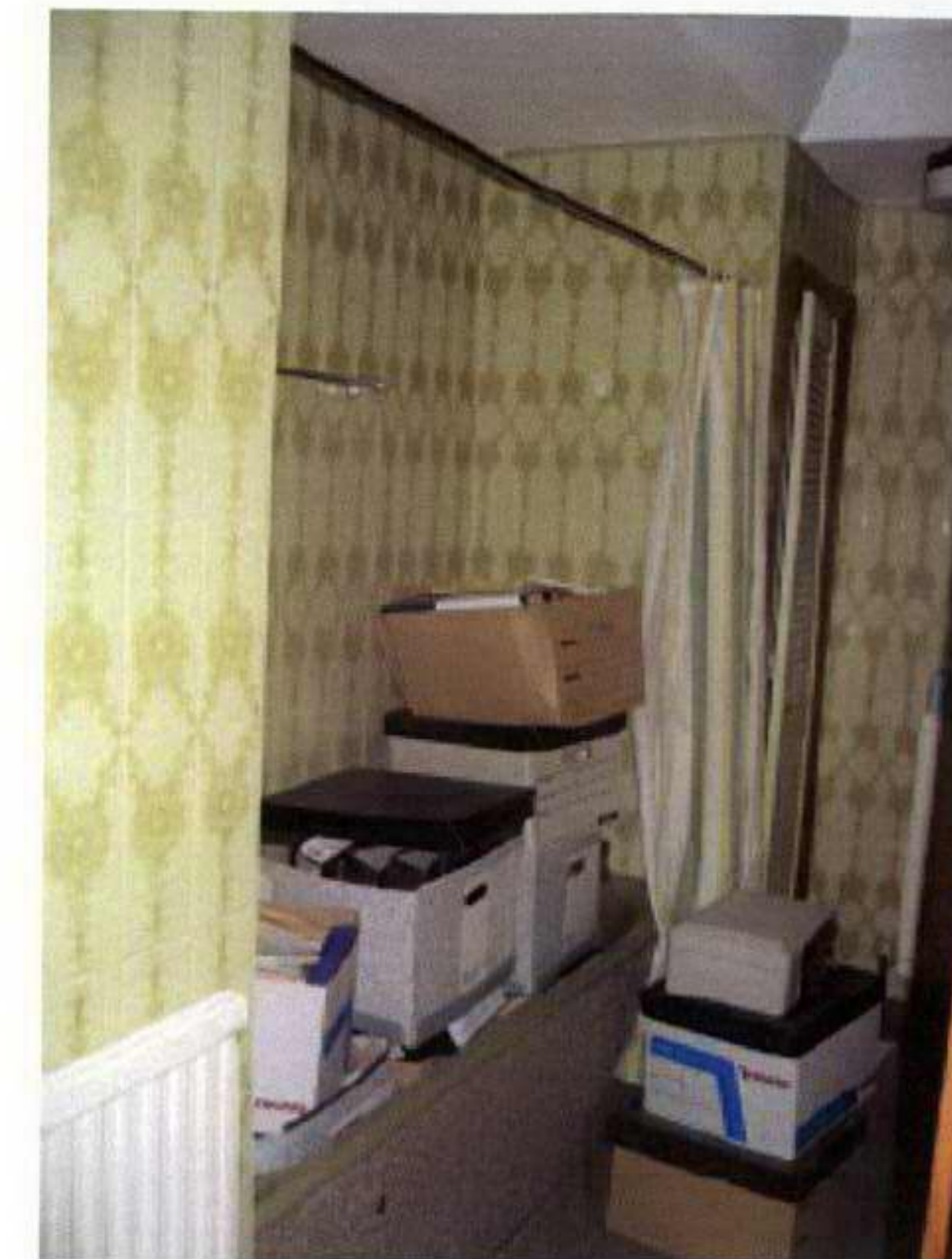
86. Third floor bathroom ET4
