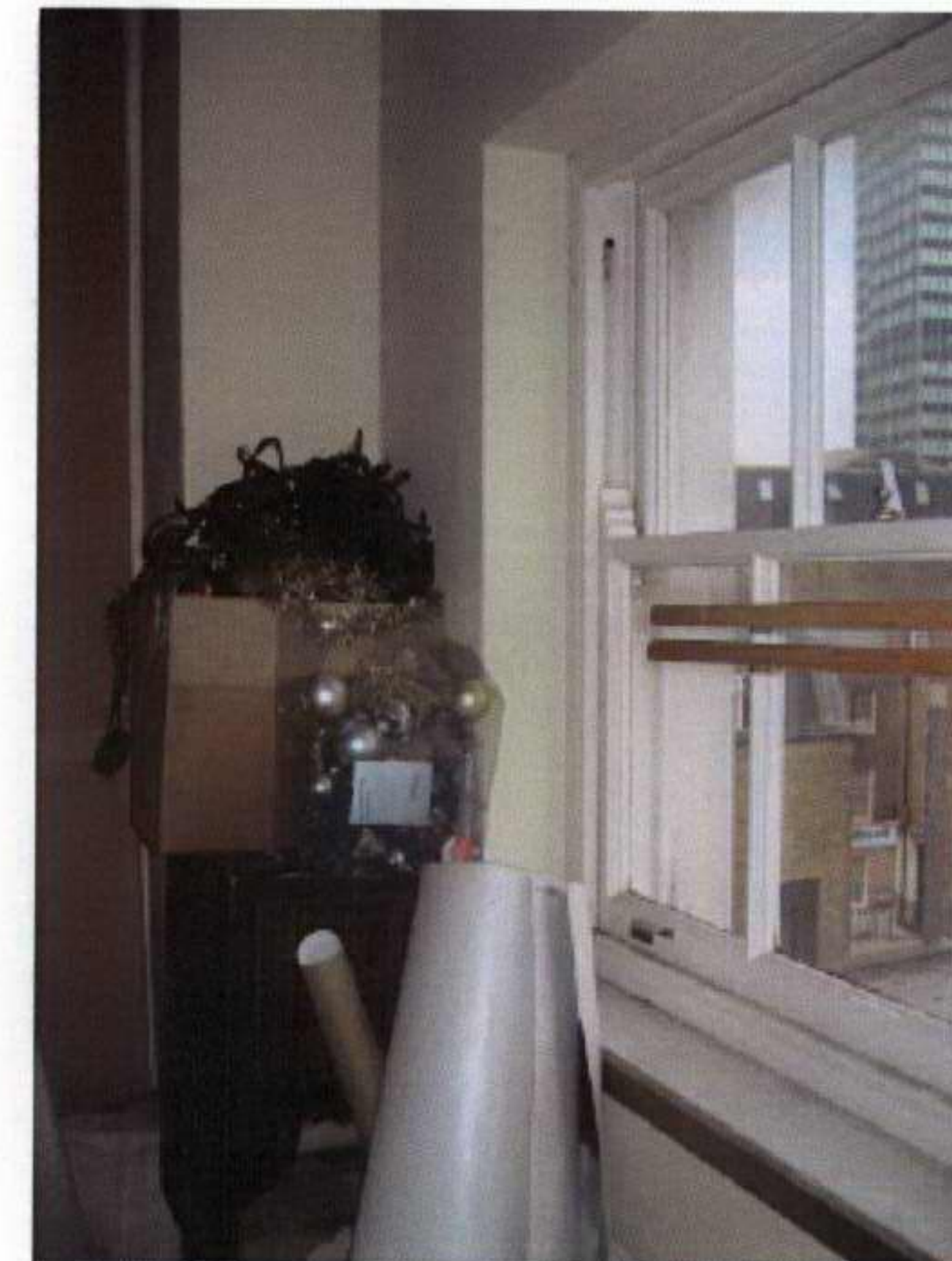
78. Third floor rear office ET6
