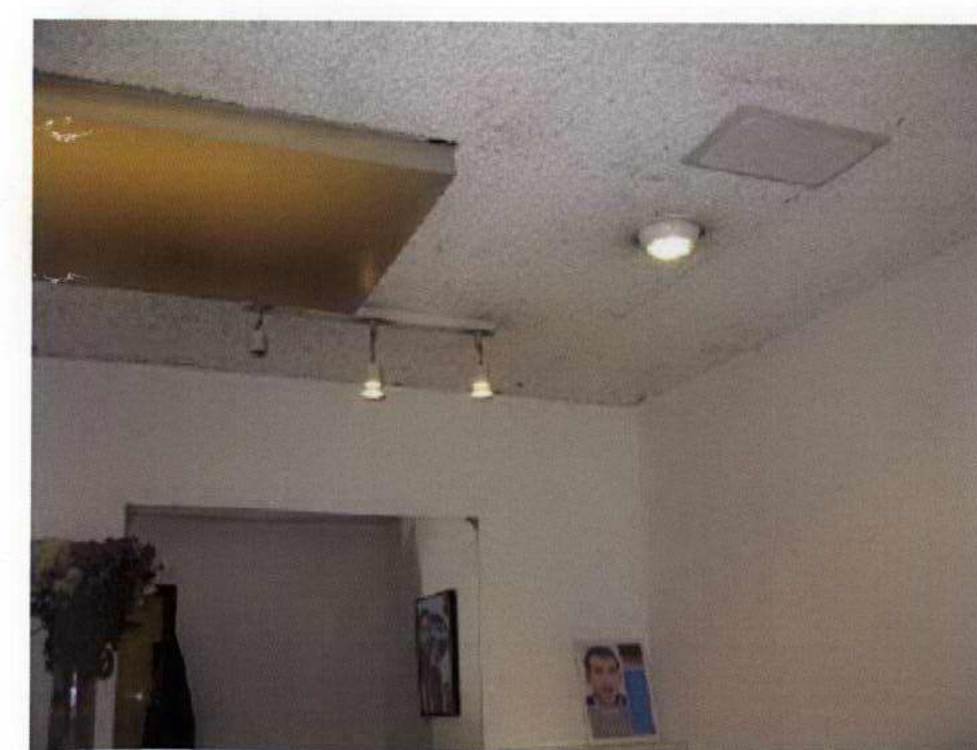
10. Basement suspended ceiling EB9
