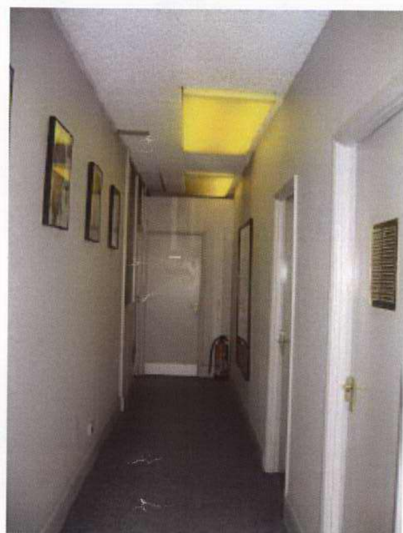
25. Ground floor main corridor EG9
