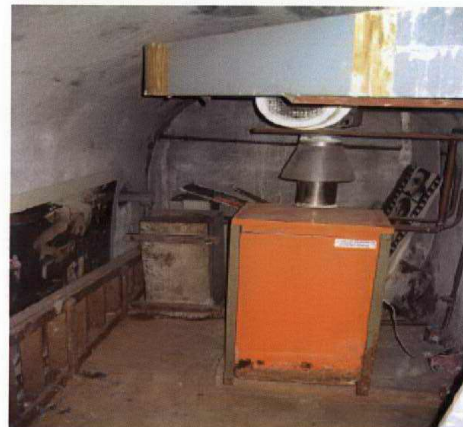
19. Basement central cellar EB2
