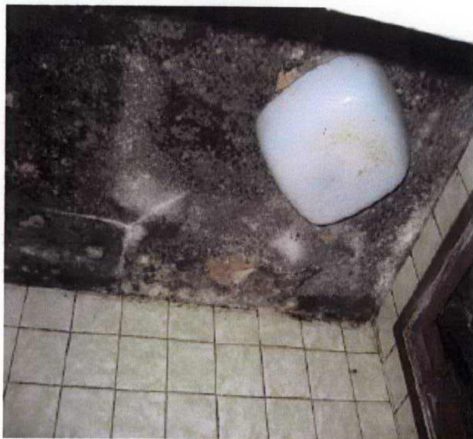
18. Basement ceiling to room EB4
