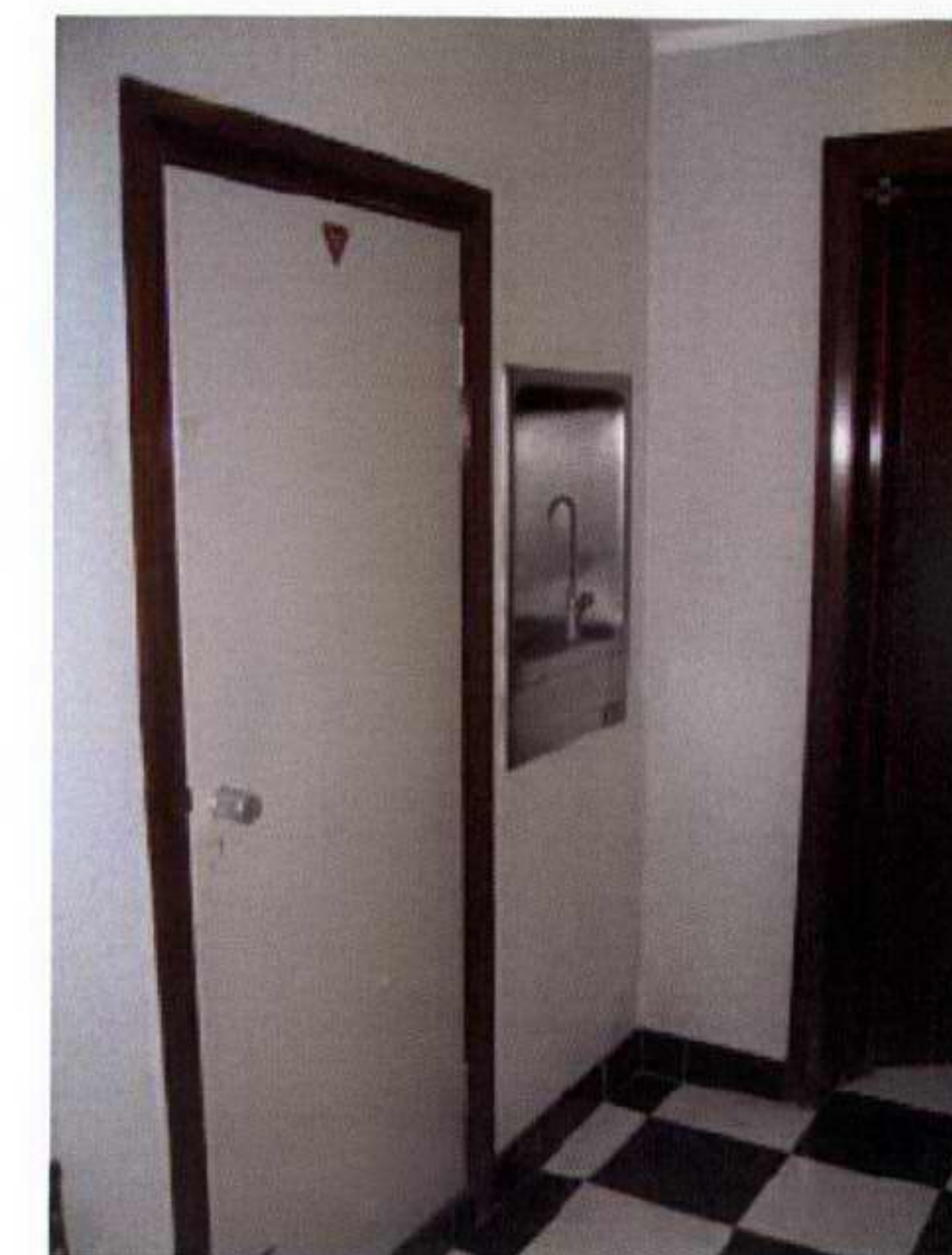
3. Basement door to EB17
