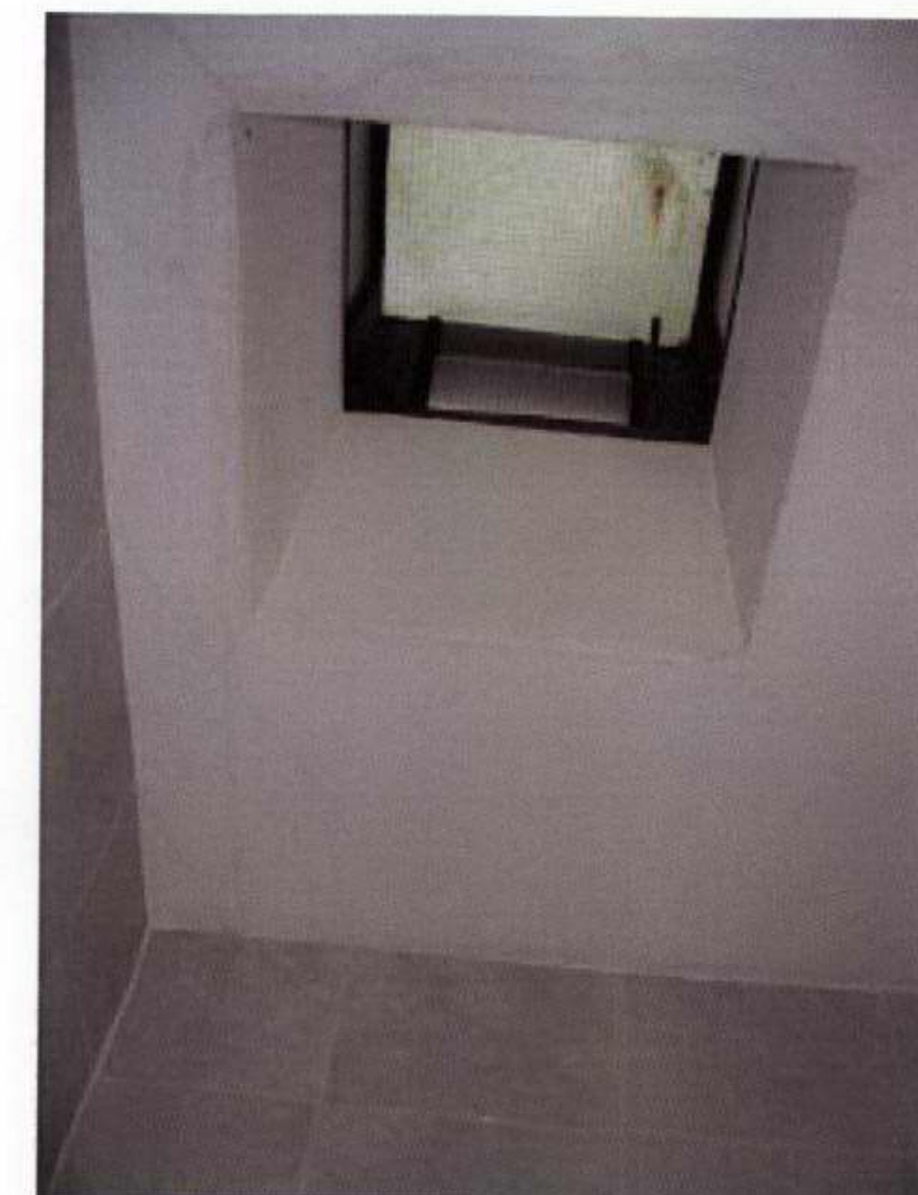
22. Ground floor W.C roof light EG10
