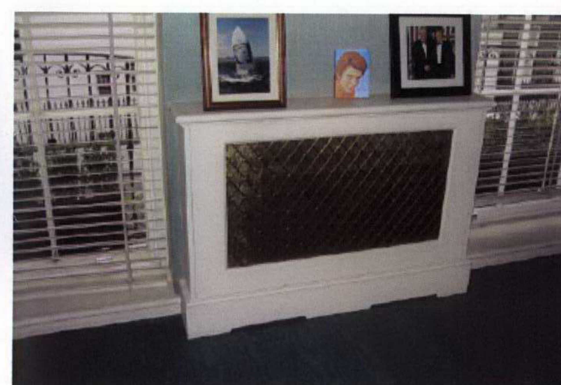
49. First floor radiator EF1
