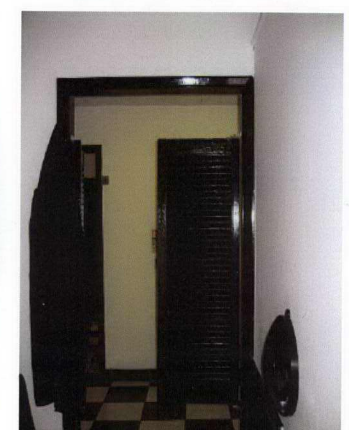
8. Basement treatment room door EB7
