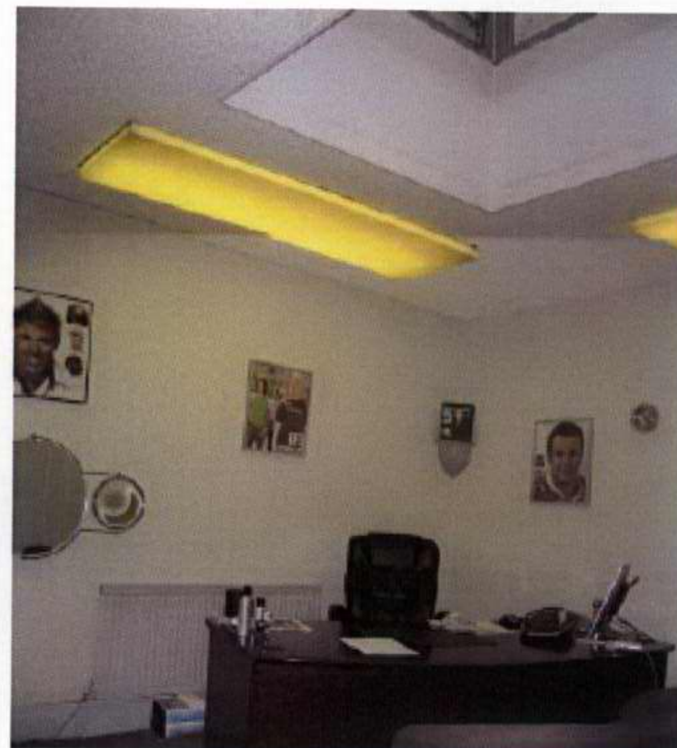
32. Ground floor consultation room EG7
