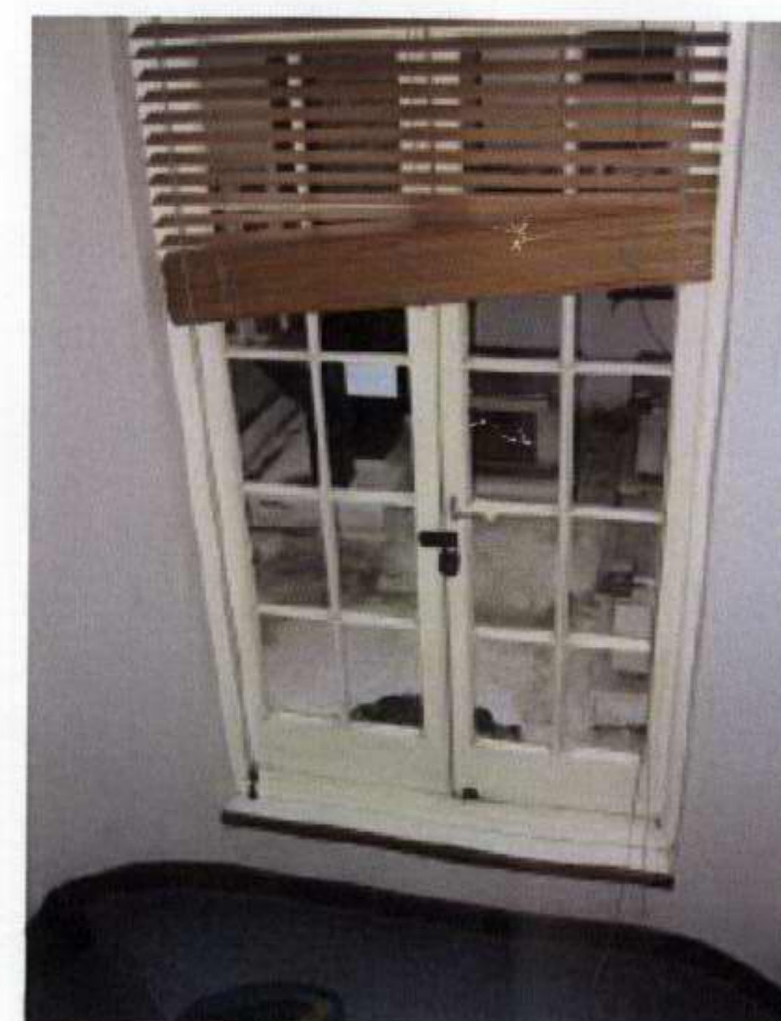
41. Ground floor window on ground/first floor landing EF4
