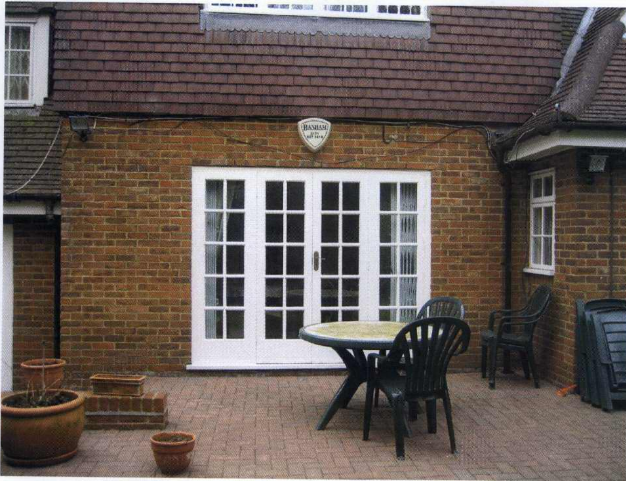
Existing — Part of Rear elevation
