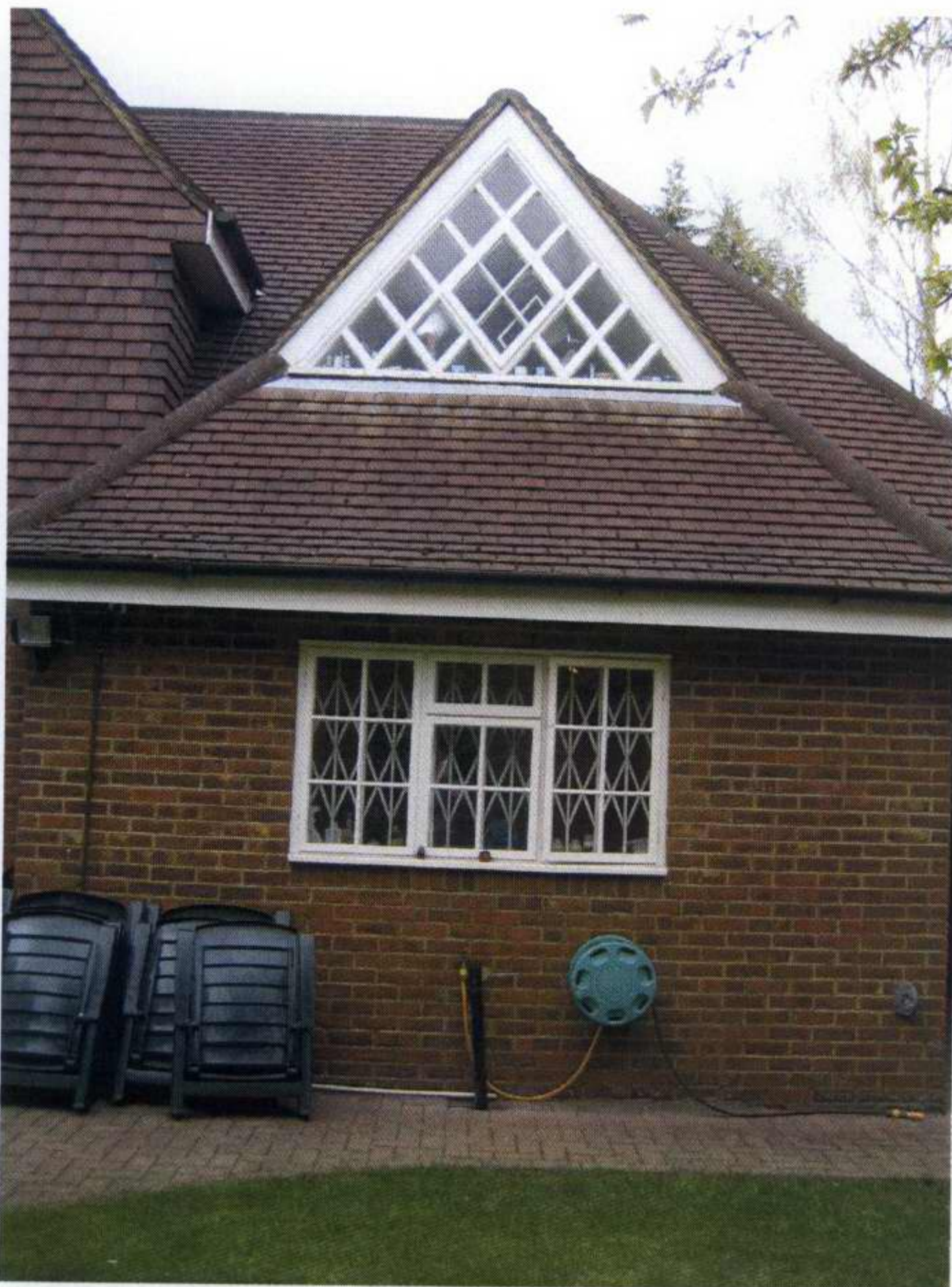
Existing — Part of Rear elevation
