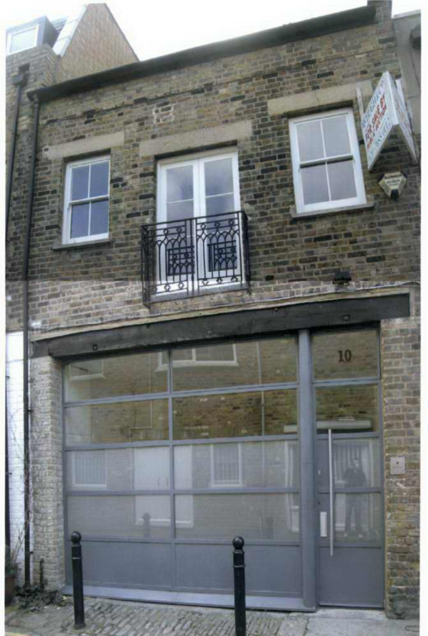
Existing photos of 10 Pratt Mews and surrounding buildings
