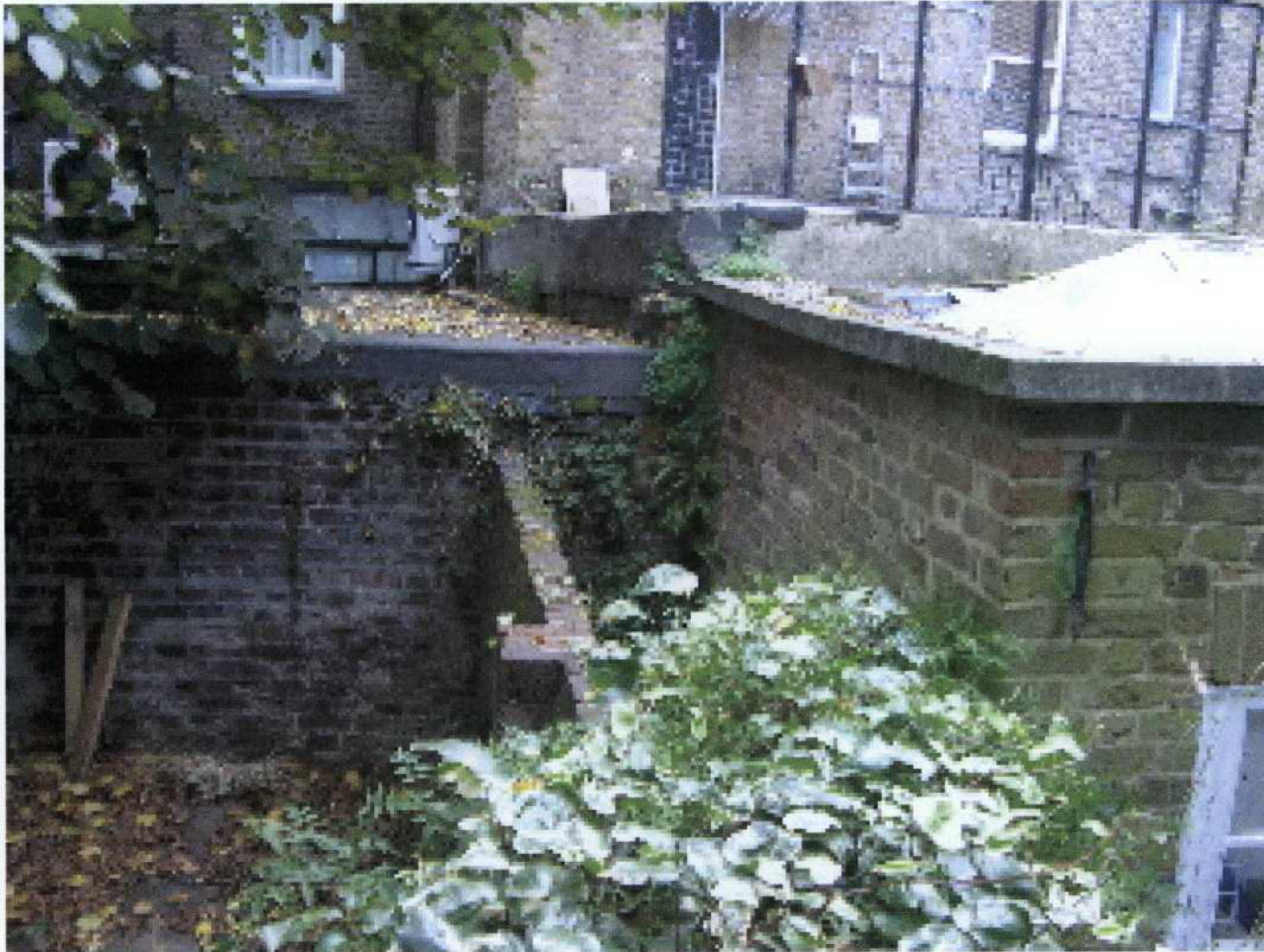
Photo 3: Rear boundary wall showing single skin construction.
