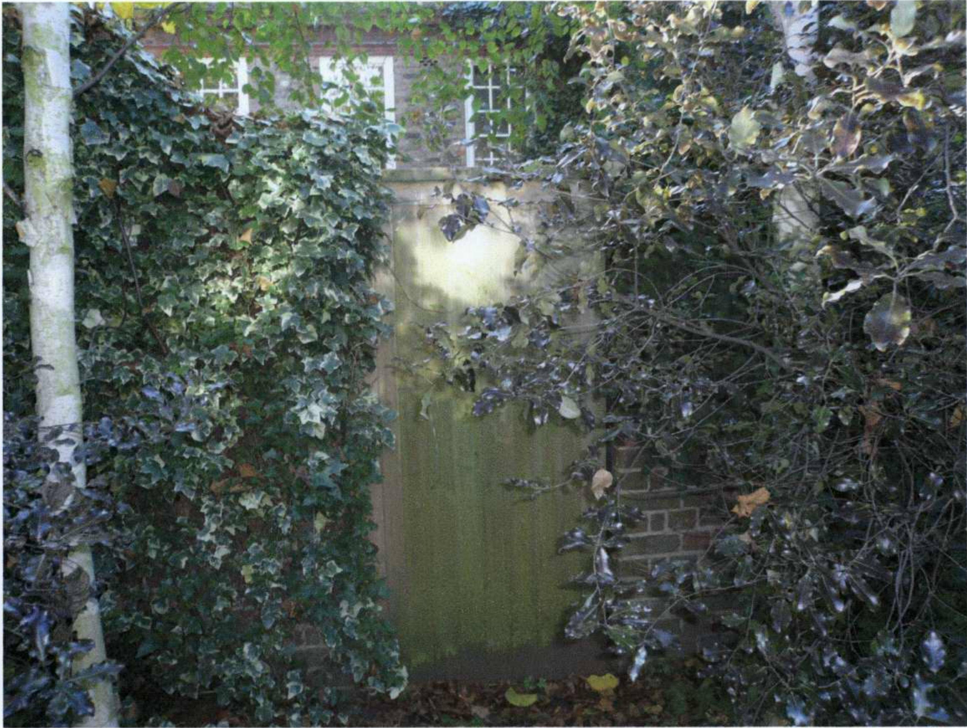
Photo 5: Intermediate garden wall (1990's) to be demolished.
