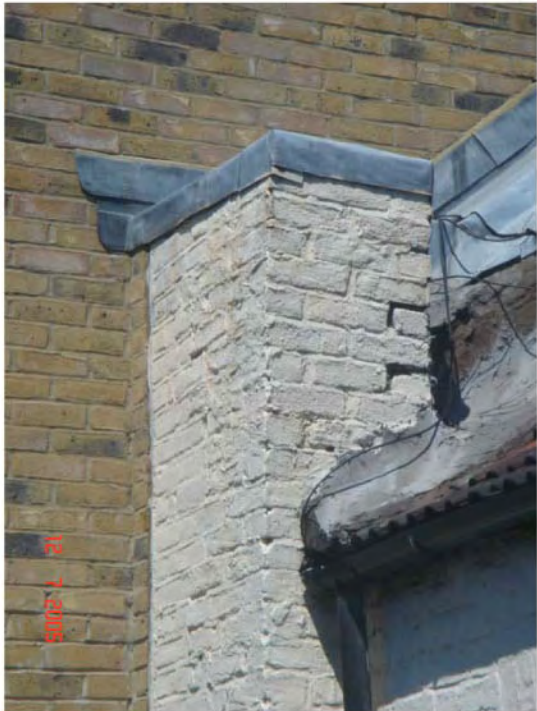
looking at rear of building (roof line) where lead work is dressed into party wall
