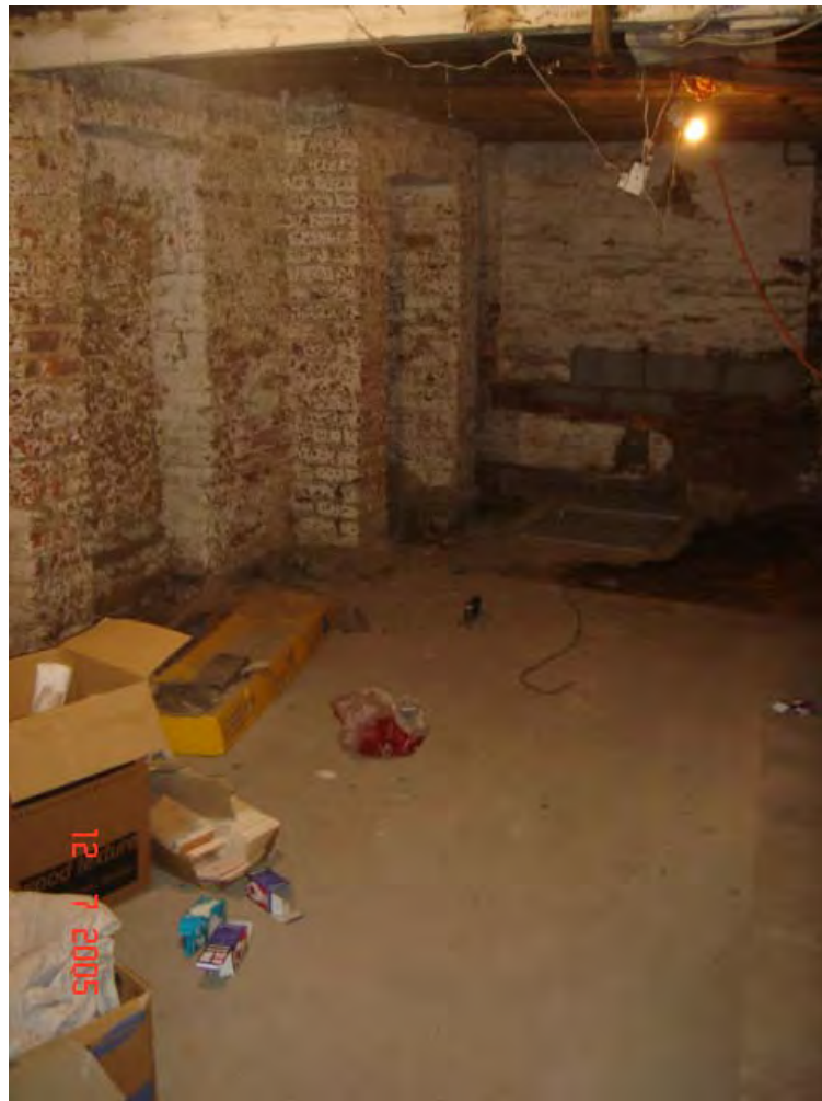
Pictures showing the earth floor in the basement and the low ceiling.
