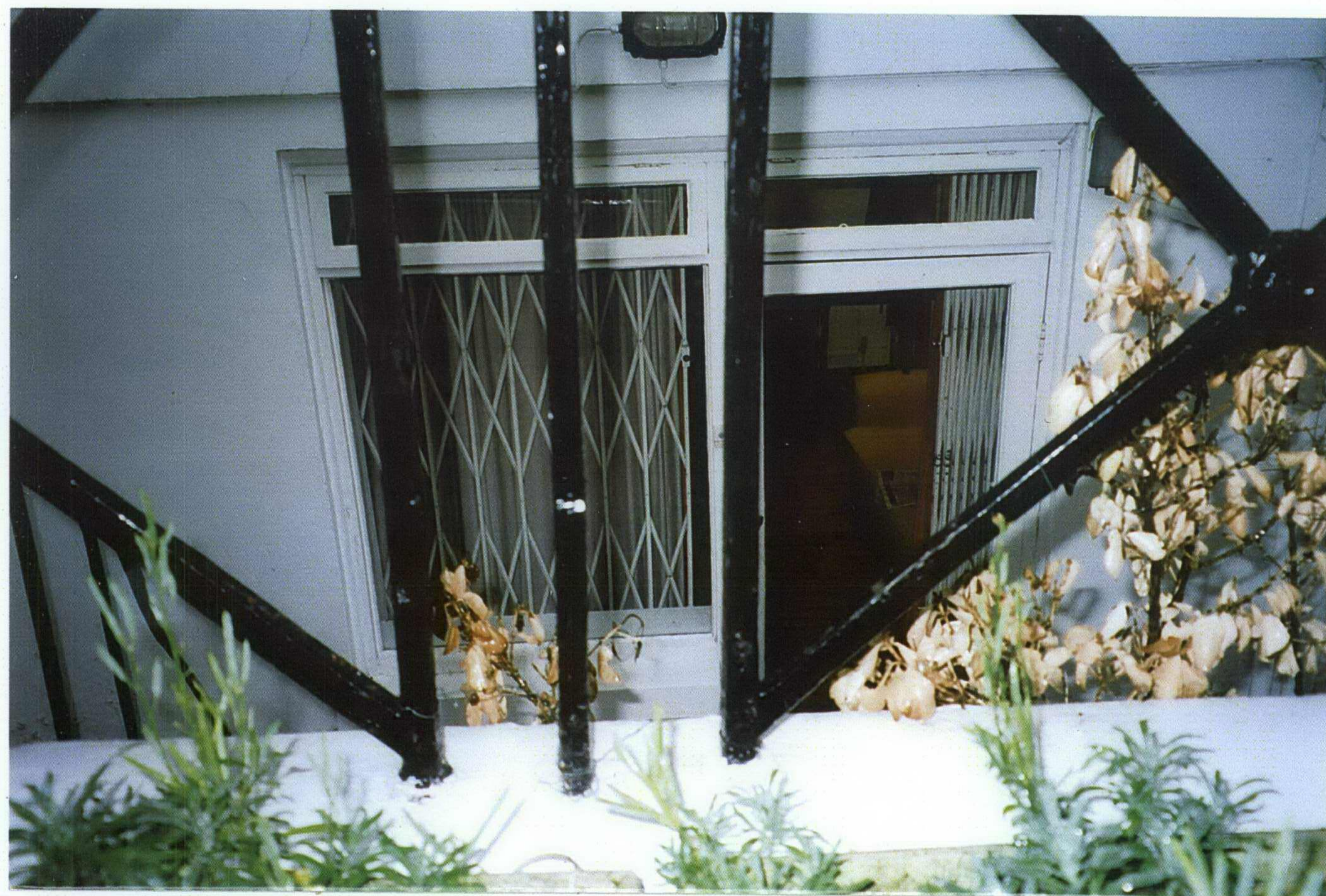
VIEW of BASEMENT FRONT DOOR AND SIDELIGHT
