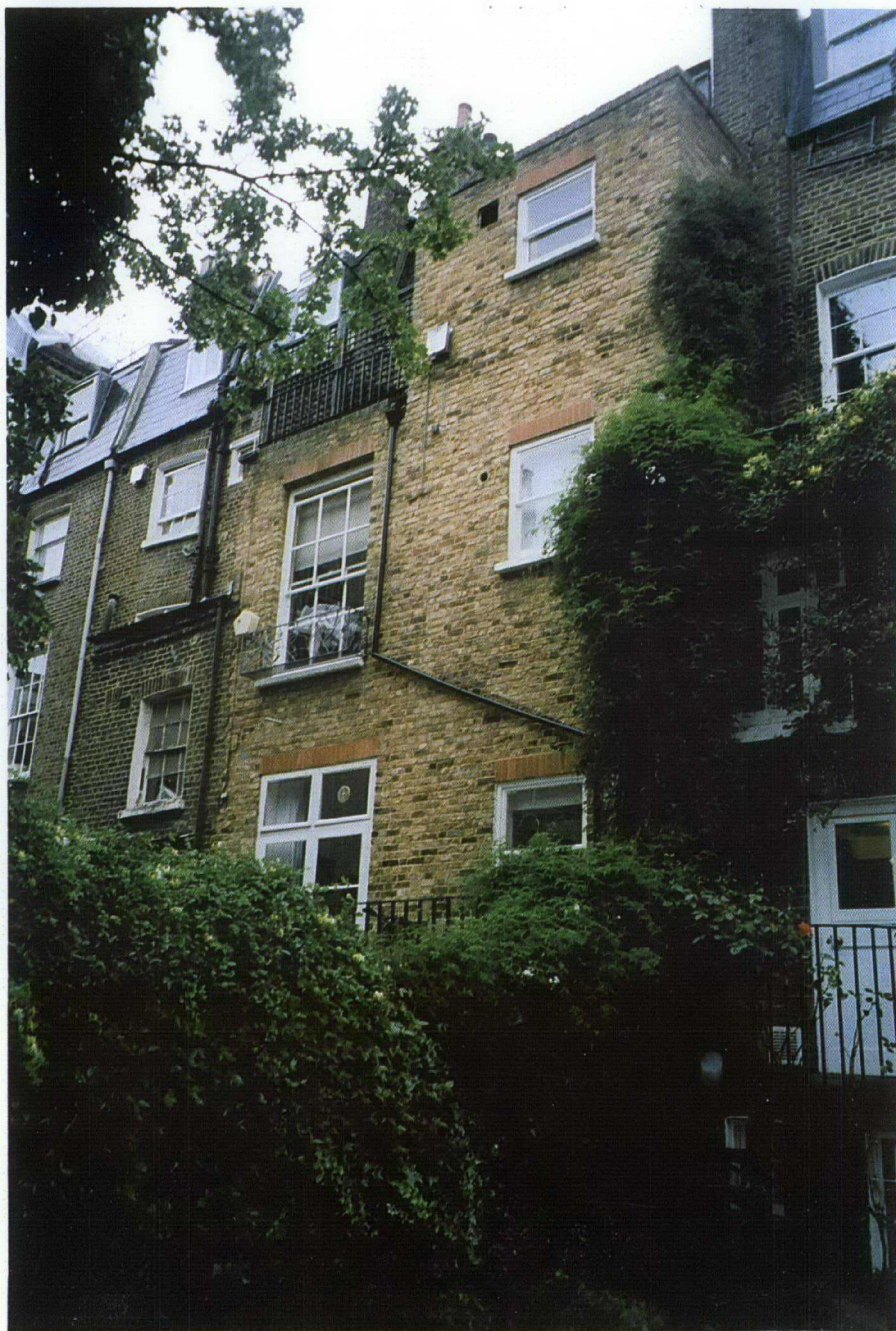
VIEW of REAR at No. 4
