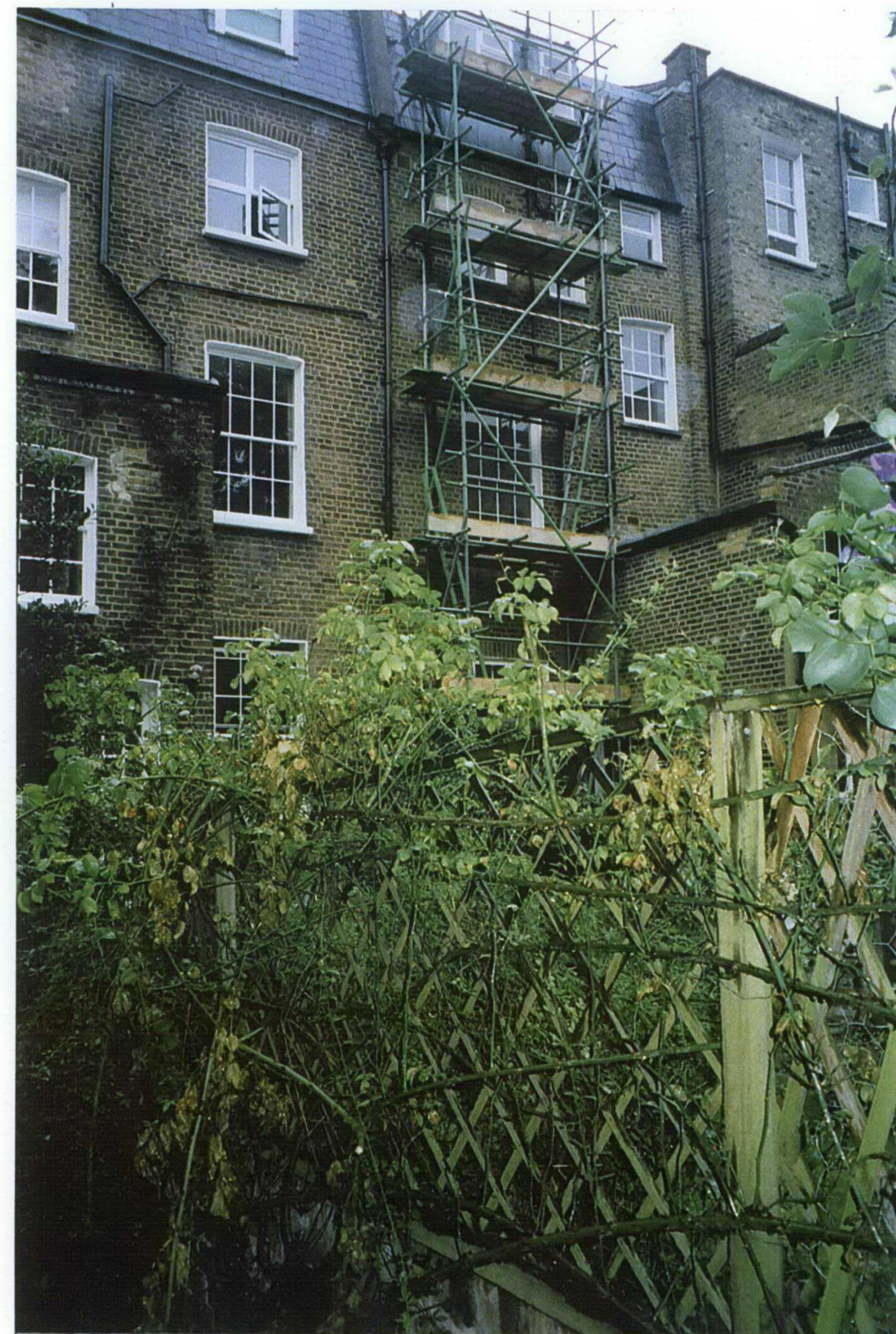
VIEW OF REAR at No. 6
