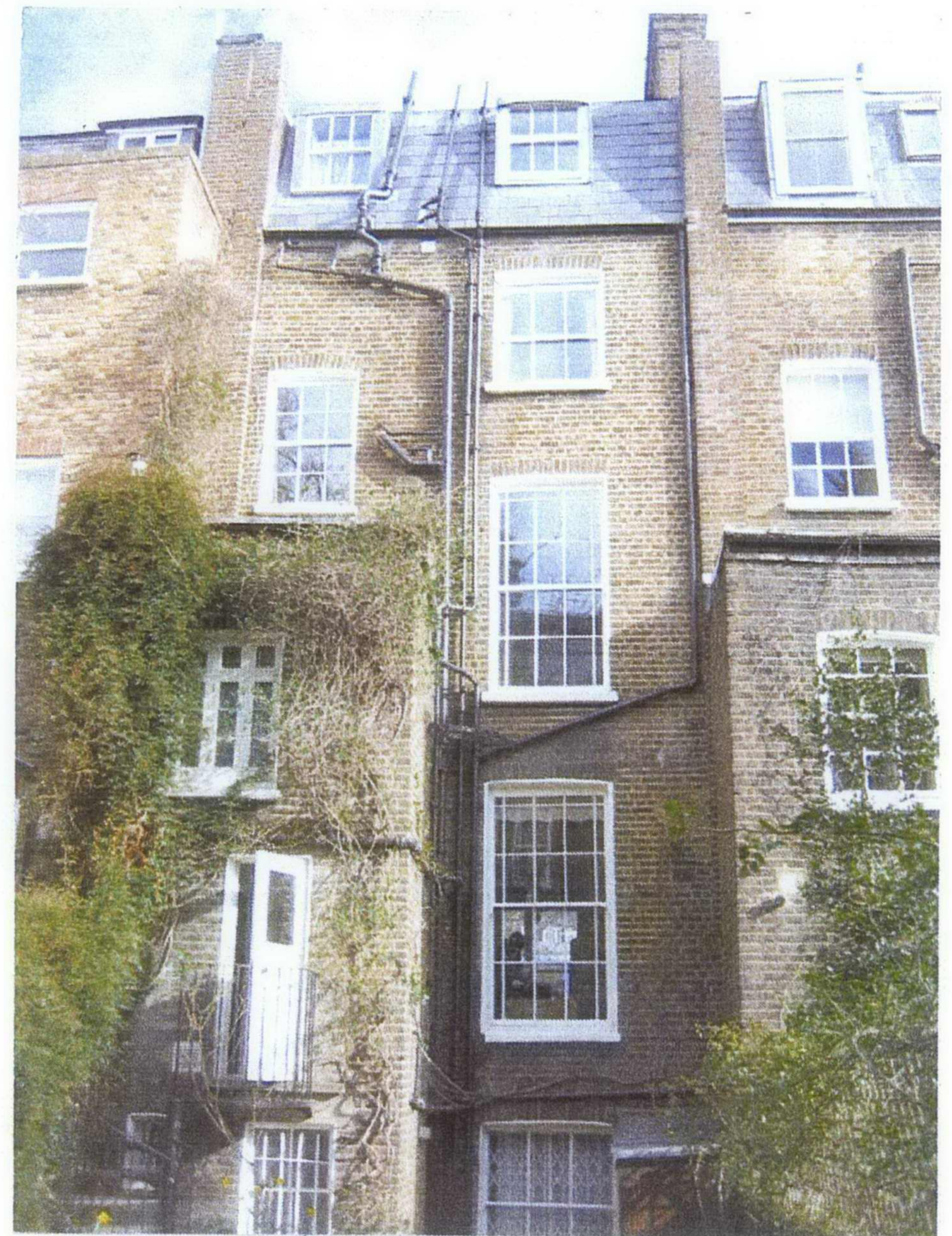
VIEW OF REAR
