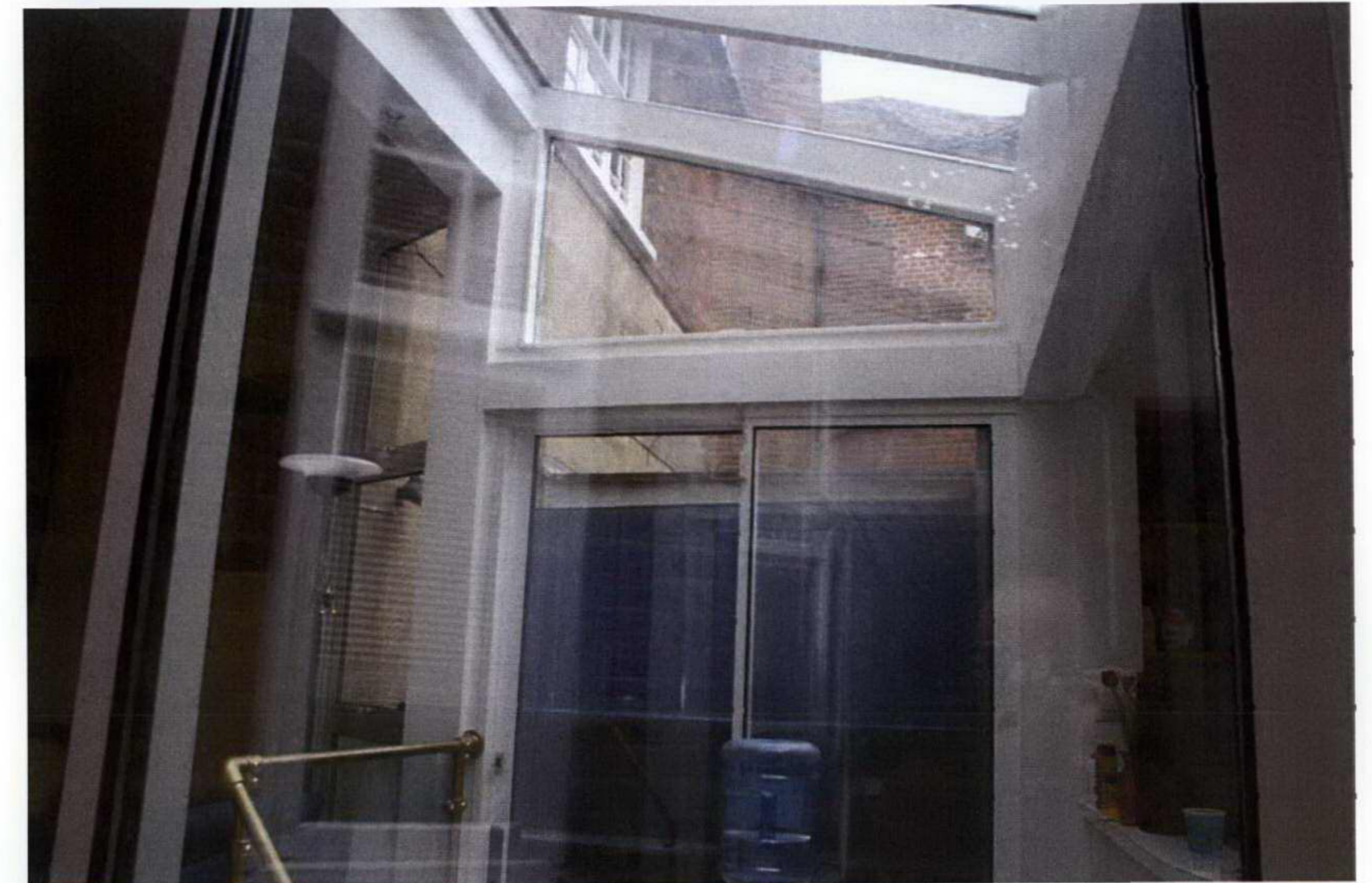
EXISTING GLAZED PASSAGE
